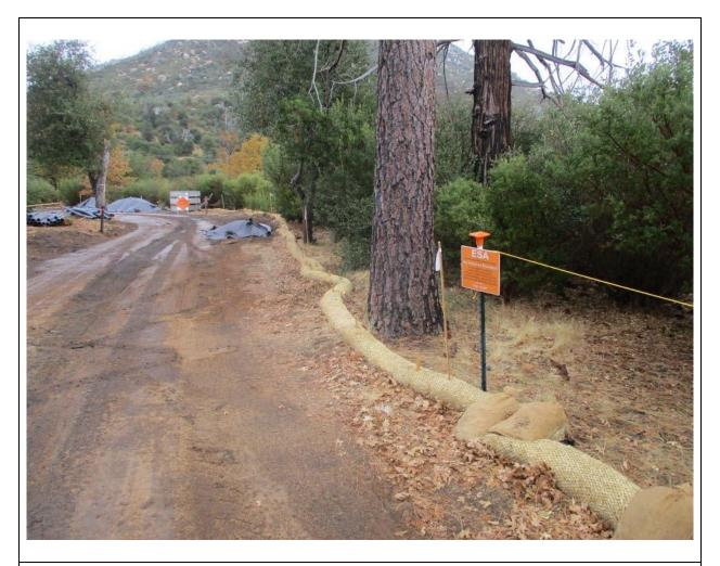
**Photo 3:** Along C 79A, rope and signage delineating cultural resources ESAs were in place and being adhered to by crews in accordance with the HPMP, APM CUL-03, and MM CUL-1. Additionally, fiber rolls were observed to be in good condition and spoils stockpiles were observed to be covered, in accordance with the Erosion Control Plan and SWPPP.
