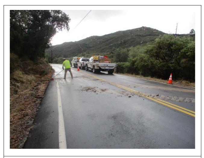
**Photo 6:** In accordance with the ECP and SWPPP, a worker was observed cleaning up trackout left on Viejas Grade Road that was left by drill demobilization. The worker noted that a street sweeper was being mobilized to the area as well.
