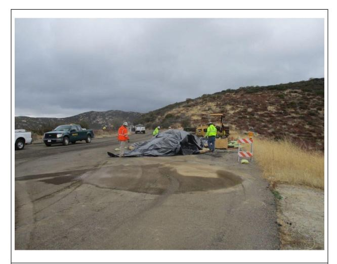
**Photo 5:** Crews were observed covering an asphalt stockpile and securing surrounding fiber rolls at a Staging Area along C 440 in preparation for a forecasted rain event, in accordance with the ECP and SWPPP.
