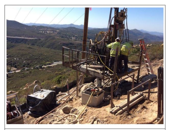
**Photo 1:** A micropile drilling crew at Pole Z273014 (TL 625C) was observed using a covered containment box to trap drill cuttings and reduce dust emissions during micropile drilling in accordance with APM AIR-05.
