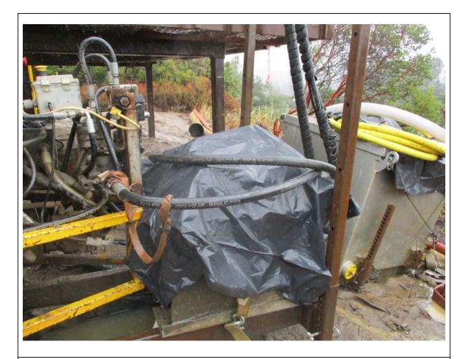
**Photo 4:** In accordance with the SNRP and MM PHS-2, a fuel cell at Pole Z173163 (TL 629A) was observed to be covered during a rain event in order to prevent the containment from filling up and any possible hazardous materials from making contact with the ground.
