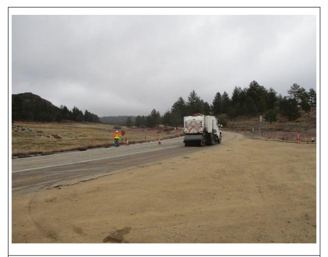
**Photo 5:** A street sweeper was used to clean up debris resulting from saw cutting near station 230+50 (C 440) along Sunrise Highway, in accordance with the ECP and SWPPP.
