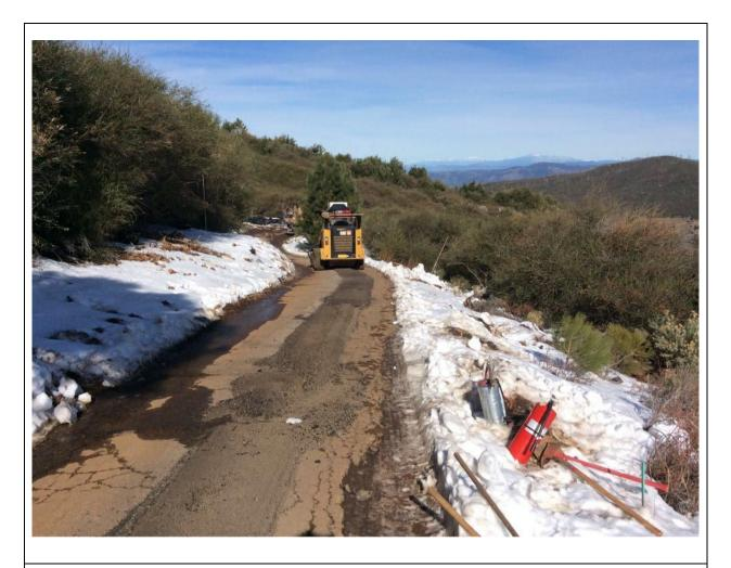
**Photo 4:** During grinding near station 57+50 on C 79A, a full set of fire tools (5-gallon backpack pump, round point shovel, Pulaski, and 2A10BC fire extinguisher) was staged within 50 feet of the activity in accordance with APM HAZ-04 and the CFPPP.
