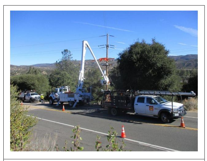
**Photo 6:** During wire work associated with the stringing of a customer service line at Pole Z774865 (TL 629A), cones and flagpersons were used to direct one-way traffic around construction equipment on Pine Valley Road in accordance with APM TRANS-02.
