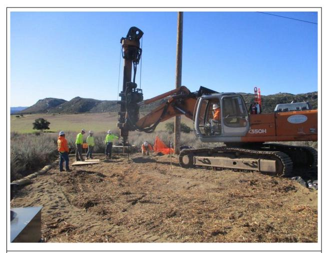
**Photo 1:** A crew was observed drilling a direct bury pole hole at Pole Z46586 (TL 6923) within the approved work limits in accordance with MM BIO-1 and with a complete set of fire tools on the drill equipment in accordance with APM HAZ-04 and the CFPPP.
