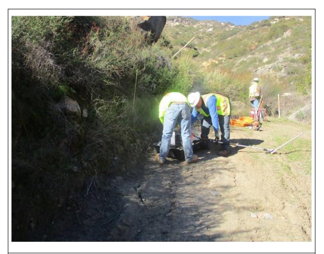
**Photo 4:** A vegetation removal crew was observed using a drip pan while refueling tools at Pole Z571489 (TL 6923) to prevent leaks or spills from being discharged onto the ground in accordance with MM PHS-2 and the SRNP.
