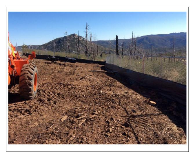
**Photo 5:** Silt fence at Azalea Staging Yard (C 79A) was observed to be in good condition in accordance with the ECP and SWPPP.
