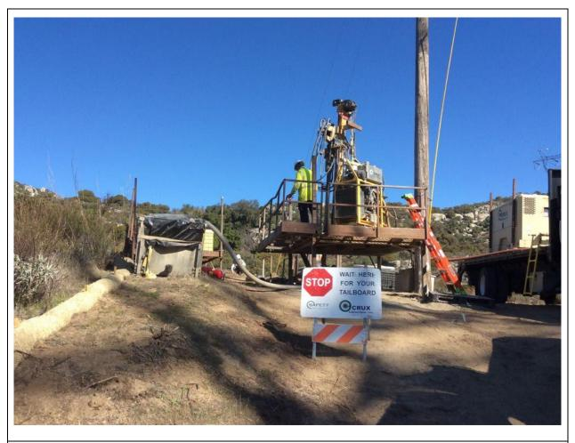
**Photo 1:** During micropile drilling at Pole Z972890 (TL 6923), a containment box was used to trap drill cuttings and reduce dust emissions in accordance with APM AIR-05.
