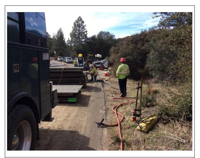
**Photo 3:** A Dedicated fire patrol, equipped with a full set of fire tools (5-gallon backpack pump, round point shovel, Pulaski, and 2A10BC fire extinguisher), was observed monitoring hot work near station 211+20 (C 440) in accordance with the CFPPP. The fire patrol noted that he had also wet down the surrounding area prior to the activity.
