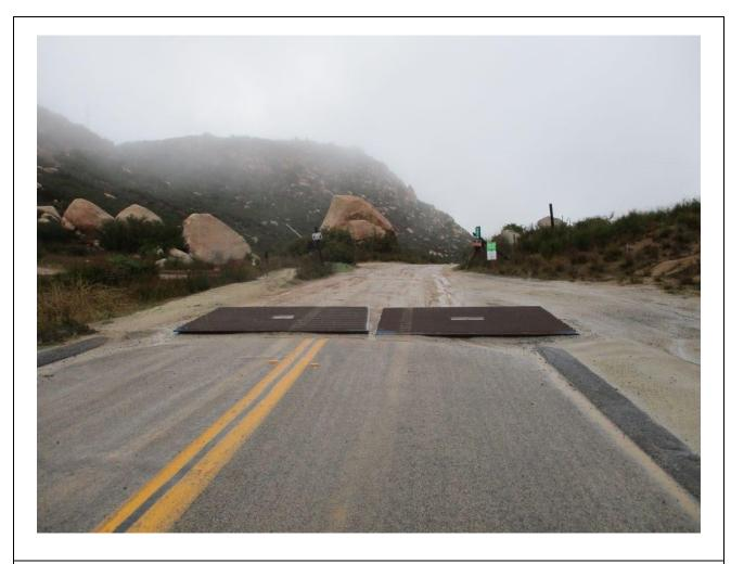
**Photo 6:** Rattle plates were observed at the point of ingress/egress to the Right of Way off Round Potrero Road (TL 6923) in accordance with the ECP and SWPPP.
