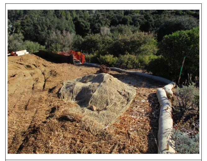
**Photo 3:** Salvaged topsoil was set aside after crane pad grading at pole Z774861. The topsoil will be used for restoration in accordance with the Habitat Restoration Plan and MM-BIO-4.
