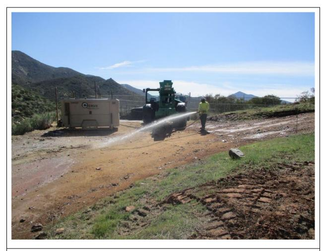
**Photo 1:** A crew member was observed wetting down the work area at Pole Z972788 (TL 6923) prior to helicopter external load operations to minimize dust emissions in accordance with APM AIR-02 and APM AIR-05.
