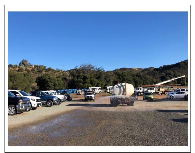
**Photo 3:** Water was applied to the ground at Bookout Staging Yard (TL 625C) to minimize dust emissions during crew egress from the yard in accordance with APM AIR-02.
