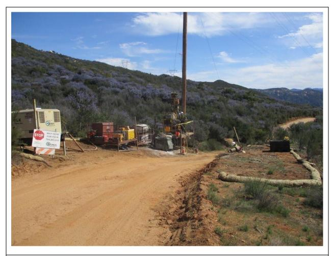
**Photo 1:** During micropile drilling at Pole Z571478 (TL 6923), perimeter erosion control BMPs were observed to be in good condition in accordance with the ECP and SWPPP.
