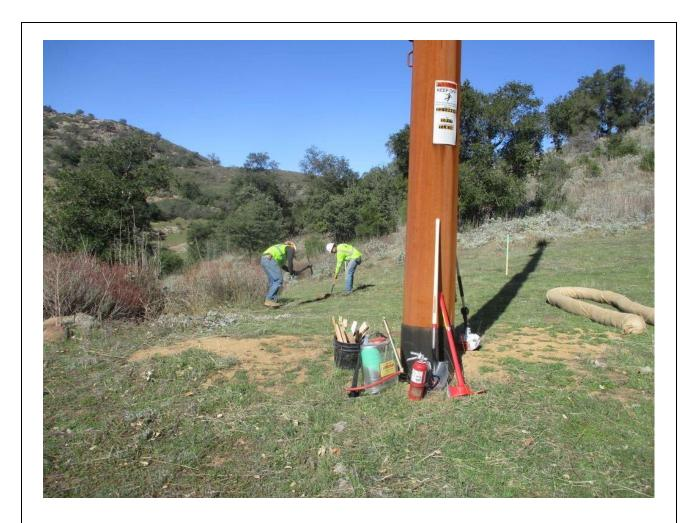
**Photo 6:** During erosion control BMP installation at Pole P259375 (TL 626 Conversion North), a full set of fire tools (5-gallon backpack pump, Pulaski, round point shovel, and 2A10BC fire extinguisher) was observed within 50 feet of the activity in accordance with APM HAZ-04 and the CFPPP.
