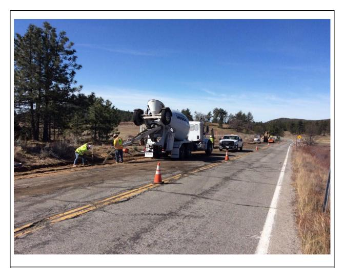
**Photo 2:** Crews were observed trenching, installing conduit, and slurrying in the conduit package along Sunrise Highway (C 440). A pilot vehicle was used to lead one-way traffic through the work area in accordance with the Traffic Control Plan and APM TRANS-02.
