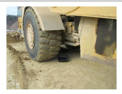
**Photo 6:** In accordance with APM-HYD-1, secondary containment was used under staged construction equipment to prevent potential leaks from being discharged into the soil.
