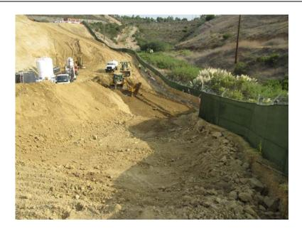
**Photo 1:** Earthwork activities occurring along the eastern limits of the project site following the completion of groundwater removal activities.
