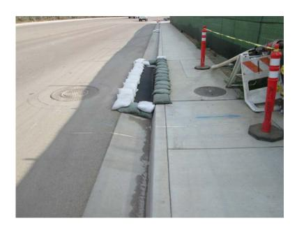
**Photo 5:** In accordance with APM-HYD-1, inlet protection BMPs were utilized at all applicable storm drains to minimize the potential for sediment laden water from entering waterways.
