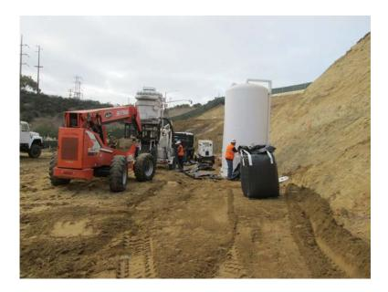
**Photo 2:** Decommissioning of the groundwater dewatering system occurred during this reporting period. Construction crews were observed hauling filler material offsite that was extracted from filtration tanks.
