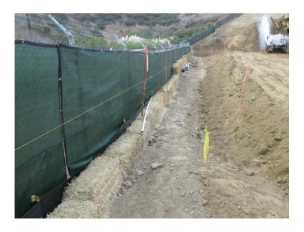
**Photo 4:** In accordance with APM-HYD-1, storm water control BMPs were used along the eastern site perimeter to prevent erosion and silt laden runoff from entering the adjacent wetland ESA.
