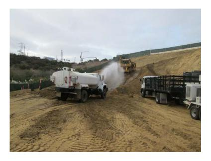
**Photo 7:** In accordance with APM-HYD-1, water was applied in areas of active construction and along access roads to prevent wind erosion and dust.
