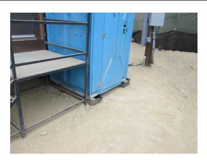
**Photo 3:** In accordance with APM-HYD-1, secondary containment has been placed beneath portable bathrooms to prevent potential leaks from being discharged into the soil.
