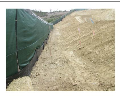
**Photo 1:** In accordance with APM-HYD-1, BMPs consisting of silt fence have been installed along the eastern perimeter of the project site.
