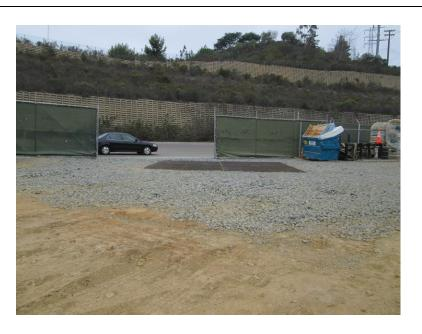
**Photo 6:** In accordance with APM-HYD-1, rumble plates and a rock apron have been installed at the project entrance to minimize the potential for sediment being tracked onto Mira Sorrento Place.
