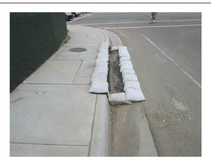
**Photo 2:** In accordance with APM-HYD-1, inlet protection BMPs are being utilized at storm drains to minimize the potential for sediment laden water from entering waterways.
