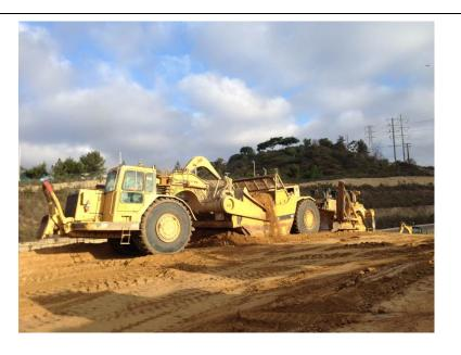
**Photo 2:** Earthwork activities along the northern project limits were completed during this reporting period to establish an access route for importing fill material that will be utilized for erecting the retaining wall.
