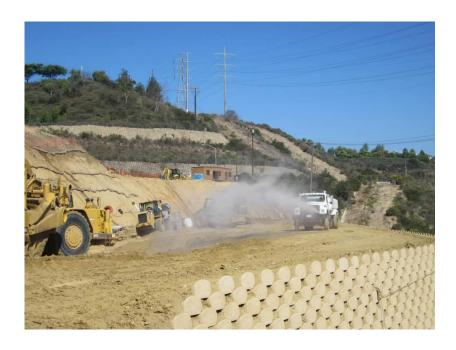
Photo 2: Construction crews utilize water for dust control and compaction purposes.
