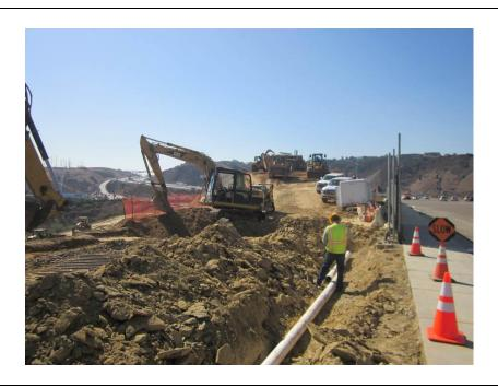
**Photo 3:** Storm drain piping being installed along the southern limits of Mira Sorrento Place.
