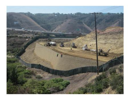
**Photo 1:** Construction activities associated with erecting the eastern retaining wall continued during this reporting period.
