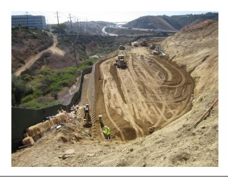
**Photo 4:** Silt fence and straw bales are being maintained along the eastern limits of the project site in accordance with the SWPPP.
