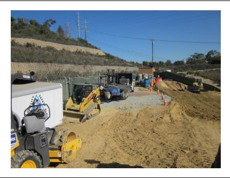
**Photo 4:** A rock apron and rattle plate is being maintained at the project entrance to minimize the potential for trac-out along Mira Sorrento Place.
