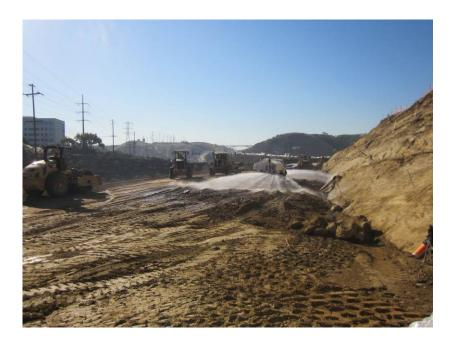
**Photo 1:** Soils being compacted through use of heavy construction equipment and water along the top of the retaining wall.
