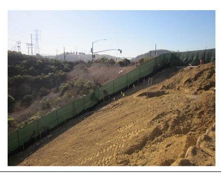
**Photo 3:** In accordance with MM-HYD-1, Best Management Practices (BMPs) consisting of silt fence and straw bales are being maintained along the eastern perimeter of the project site.
