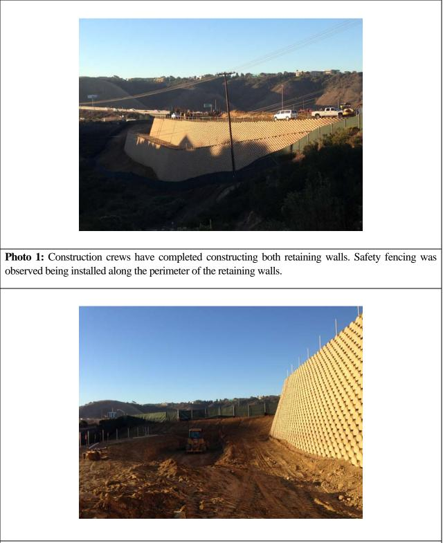
**Photo 2:** Excavation associated with constructing the retention basin located in the southwest corner of the project site continued during this reporting period.
