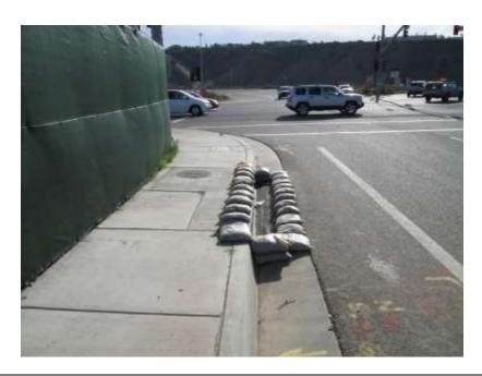
**Photo 4:** Gravel bags and filter fabric were observed being maintained at stormwater inlet structures located adjacent to construction activities in accordance with APM-HYD-1
