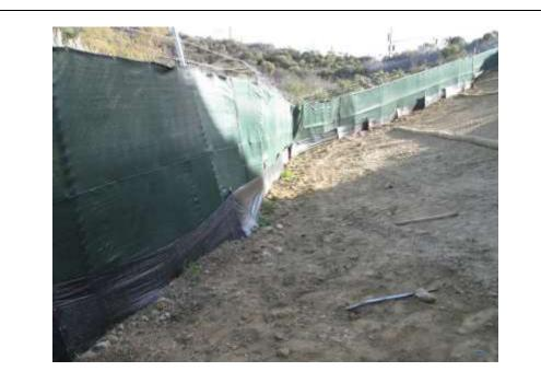
**Photo 3:** Silt fencing was observed being maintained along the eastern limits of the substation adjacent to environmental sensitive areas in accordance with APM-HYD-1
