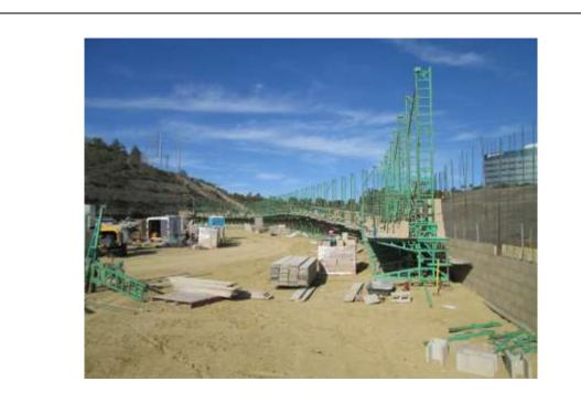
**Photo 1:** Construction crews continued work associated with erecting the screening wall along the perimeter of the substation pad.
