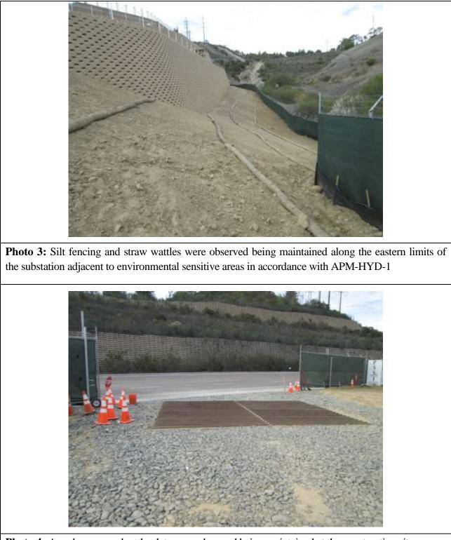
**Photo 4:** A rock apron and rattle plate were observed being maintained at the construction site entrance to minimize trac-out in accordance with APM-HYD-1.
