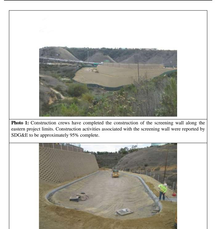
**Photo 2:** Crews were observed completing fine grading for the drainage basin located in the southwest portion of the project site.
