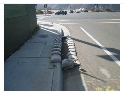
**Photo 3:** Gravel bags and filter fabric are being maintained at storm drains inlet structures located adjacent to the project site in accordance with the SWPPP and APM-HYD-1.
