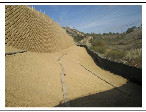
**Photo 4:** BMP's consisting of straw wattles and silt fence are being maintained along the eastern slopes of the project site in accordance with the SWPPP and APM-HYD-1.
