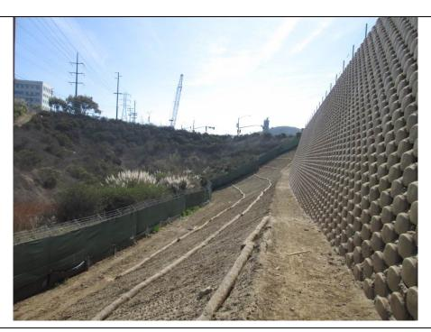
**Photo 3:** Silt fencing and straw wattles are being maintained along the eastern perimeter in accordance with the project SWPPP and APM-HYD-1.
