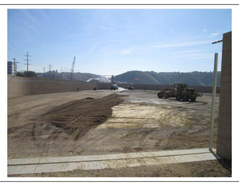
**Photo 1:** Construction crews were observed placing class 2 fill at the substation pad.
