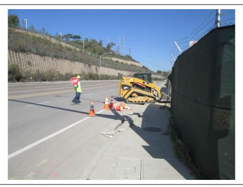
**Photo 4:** A flagger was observed being utilized when construction equipment had to temporarily access Mira Sorrento Place in accordance with the traffic control plan and MM-TT-1.
