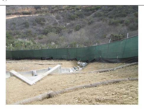
**Photo 2:** Silt fencing, straw wattles, and gravel bag check dams are being maintained along the eastern perimeter of the project site in accordance with the project SWPPP and APM-HYD-1.
