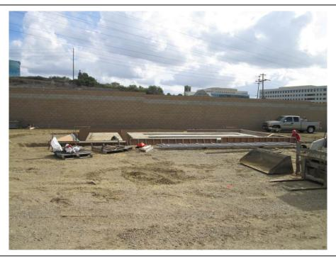
**Photo 1:** Construction crews were observed building foundations for the transformer pads during this reporting period.
