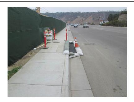
**Photo 4:** In accordance with APM-HYD-1, inlet protection BMPs designed to avoid or minimize silt from entering waterways, including filter fabric and gravel bags, were observed at two inlets along Mira Sorrento Place.
