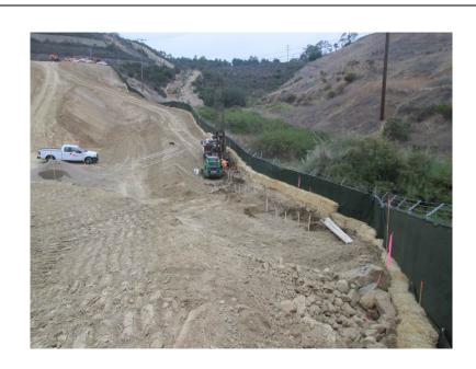
**Photo 1:** A series of groundwater wells were drilled along the eastern limits of the project site that will be utilized for groundwater extraction.
