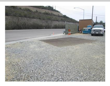
**Photo 6:** In accordance with APM-HYD-1, anti-dirt tracking control BMPs including a rock apron and rumble plates, were observed at the site ingress/egress point to prevent dirt from being tracked onto Mira Sorrento Place.
