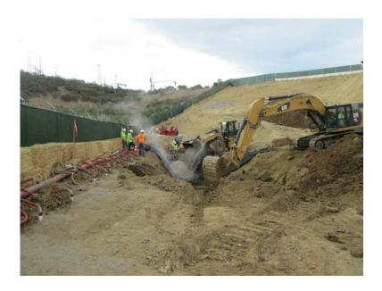
**Photo 1:** Dewatering continued along the eastern perimeter of the construction site, as soil saturated with groundwater was excavated and replaced with gravel fill in preparation for wall construction.
