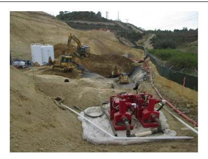
**Photo 4:** In accordance with APM-HYD-1, secondary containment was placed under staged construction equipment to prevent potential leaks from being discharged into the soil.
