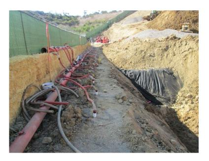
Photo 1: Groundwater wells constructed along the eastern limits of the project site.
