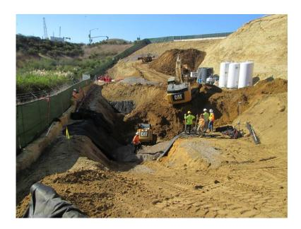
**Photo 2:** Soil saturated with groundwater, adjacent to the groundwater dewatering wells, was excavated and replaced with gravel fill in preparation for wall construction.
