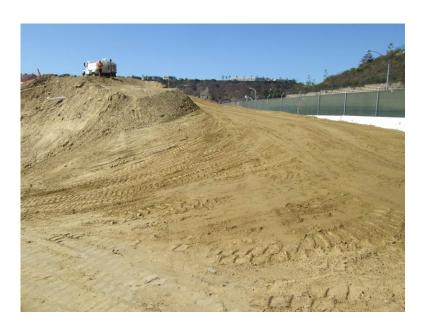
**Photo 6:** In accordance with APM-HYD-1, water was applied to the work area and to access roads to prevent wind erosion and dust creation.
