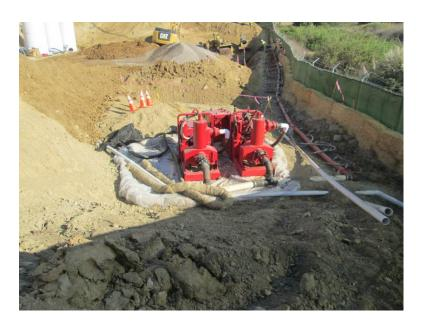
**Photo 3:** In accordance with APM-HYD-1, secondary containment is placed beneath staged construction equipment to prevent potential leaks from being discharged into the soil.
