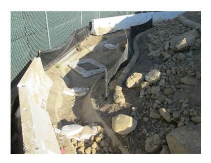
**Photo 5:** In accordance with APM-HYD-1, inlet protection BMPs were utilized at all applicable storm drains to prevent sediment laden water from entering waterways.
