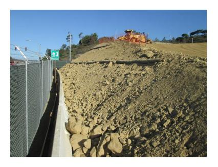
**Photo 4:** In accordance with APM-HYD-1, storm water control BMPs were observed along the site perimeter and on open cut slopes to prevent silt laden water from entering waterways.
