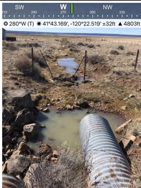
Photo 37. Irrigation canal (D14-2x, 21-2x) with break in slope and change in vegetation cover indicating OHWM.
