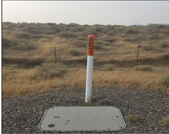
Figure 3.2-7. Example of a Typical Line Marker
