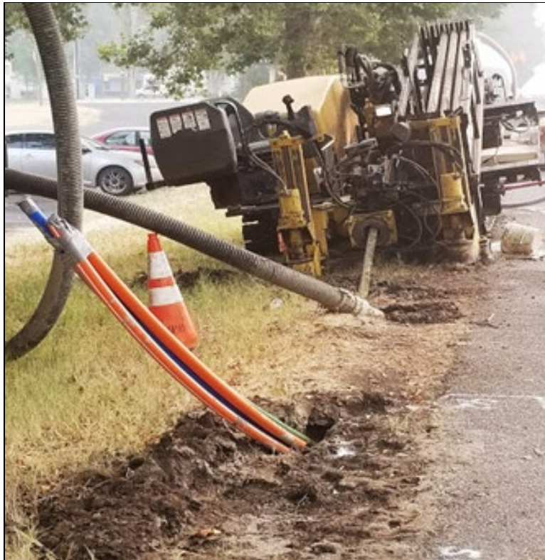
Figure 2.3-8. Example of Horizontal Drilling Rig and Conduit
