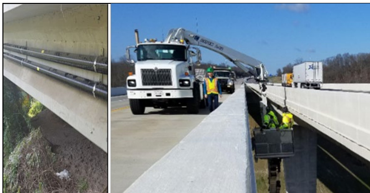
Figure 2.3-9. Examples of Bridge Attachment
