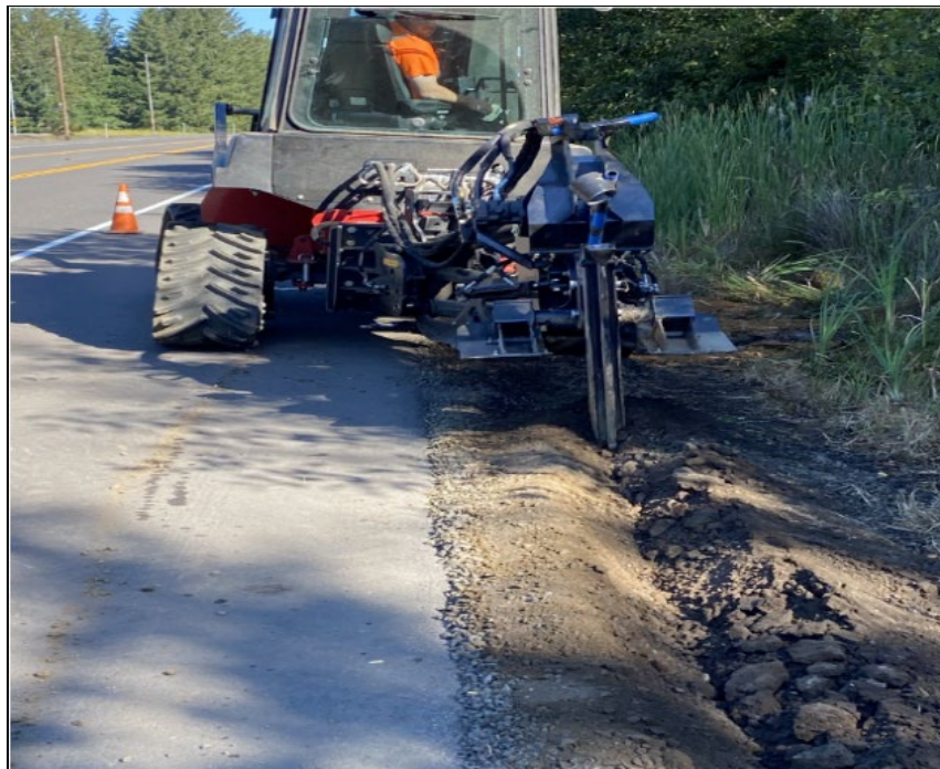
Figure 2.3-7. Typical Fiber Optic Conduit Plow
