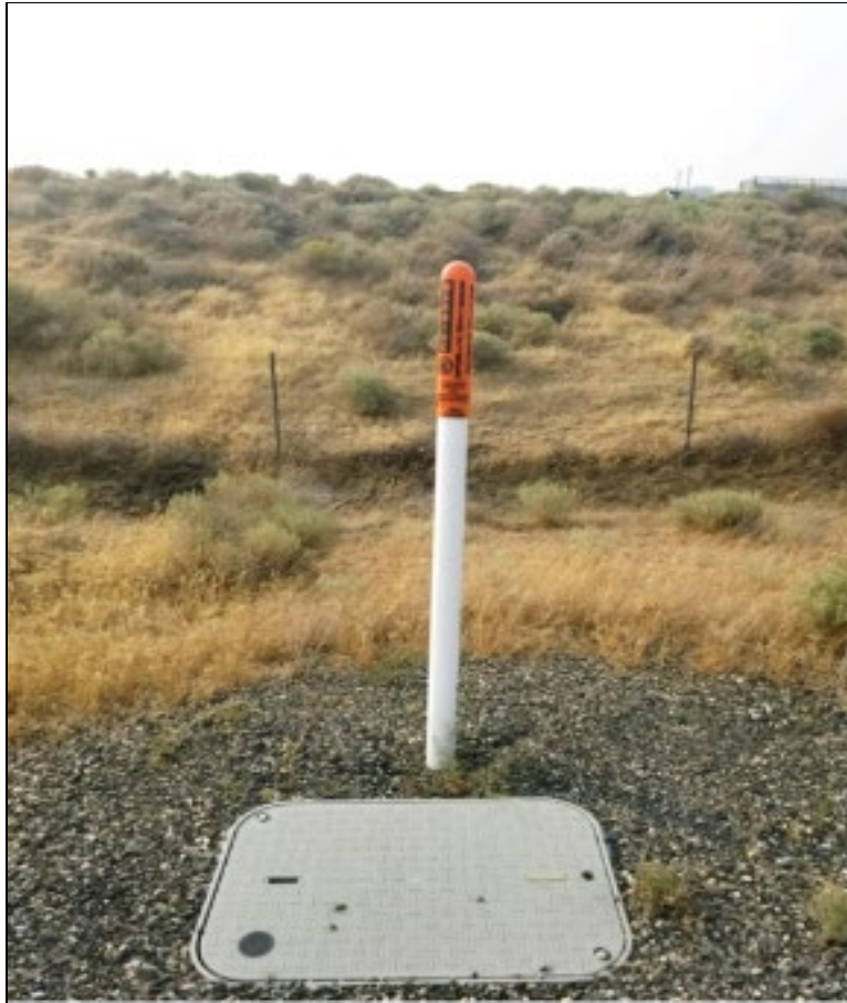
Figure 2.3-6. Typical Vault and Line Marker
