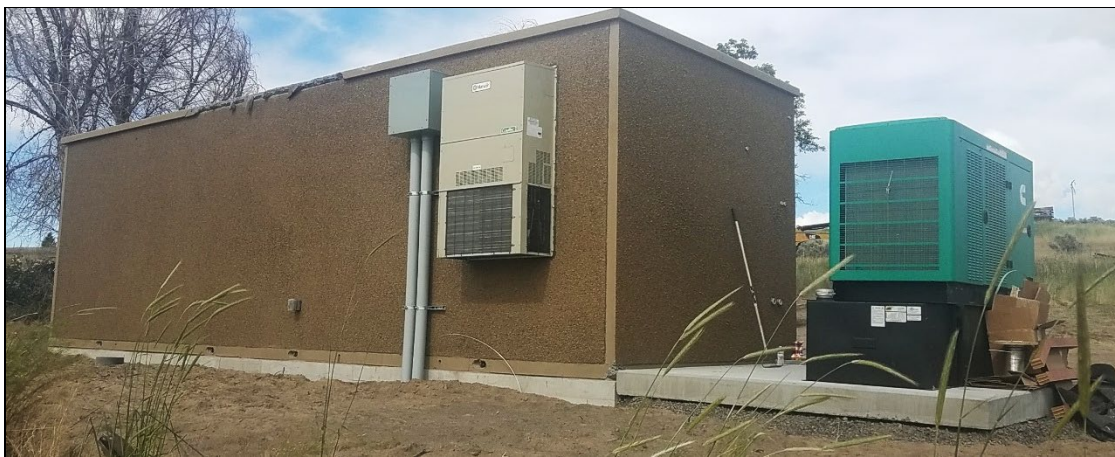
Figure 2.3-5. Example Regeneration Hut Housing an In-Line Amplifier
