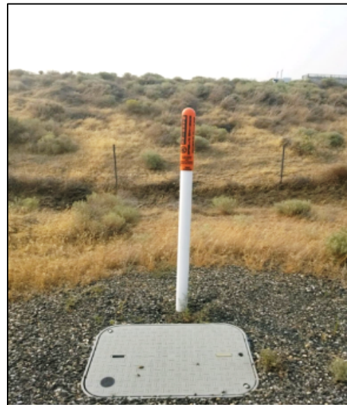
Figure 3-4: Typical Vault and Line Marker
