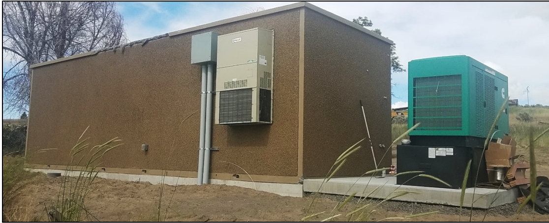
Figure 3-3: Example Regeneration Hut Housing an In-Line Amplifier
