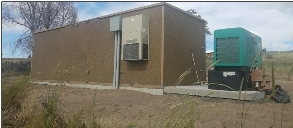
Figure 5.1-5: Example of a Typical Regeneration Hut
