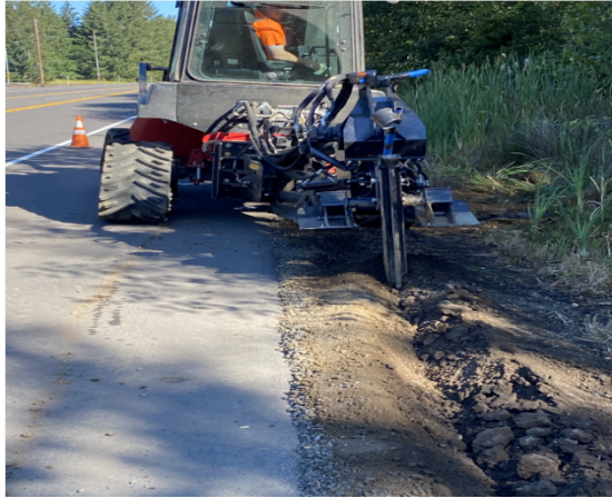
Figure 3-6: Typical Fiber Optic Conduit Plow
