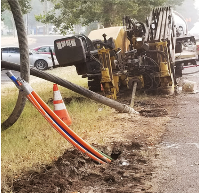
Figure 3-7: Horizontal Drilling Rig and Conduit
