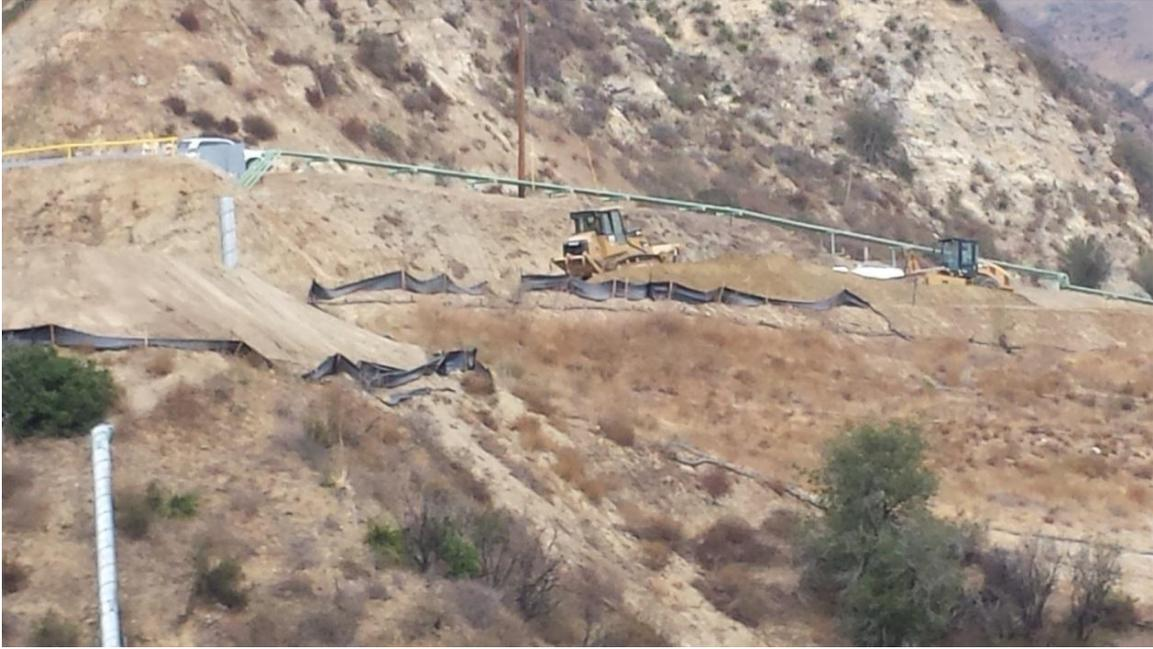
Photo 1: Maintain silt fence at P-32 Fill Site, November 11, 2014
