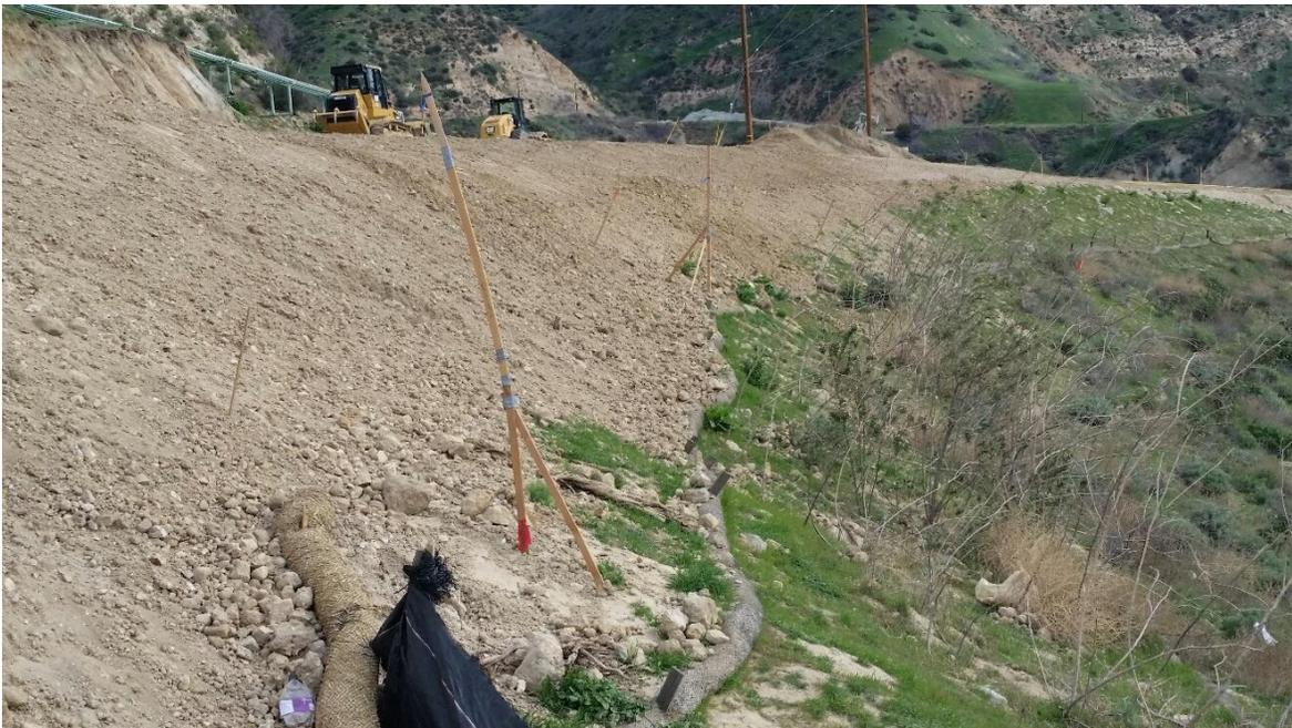
Photo 2: Maintain silt fence at P-32 Fill Site, January 26, 2015
