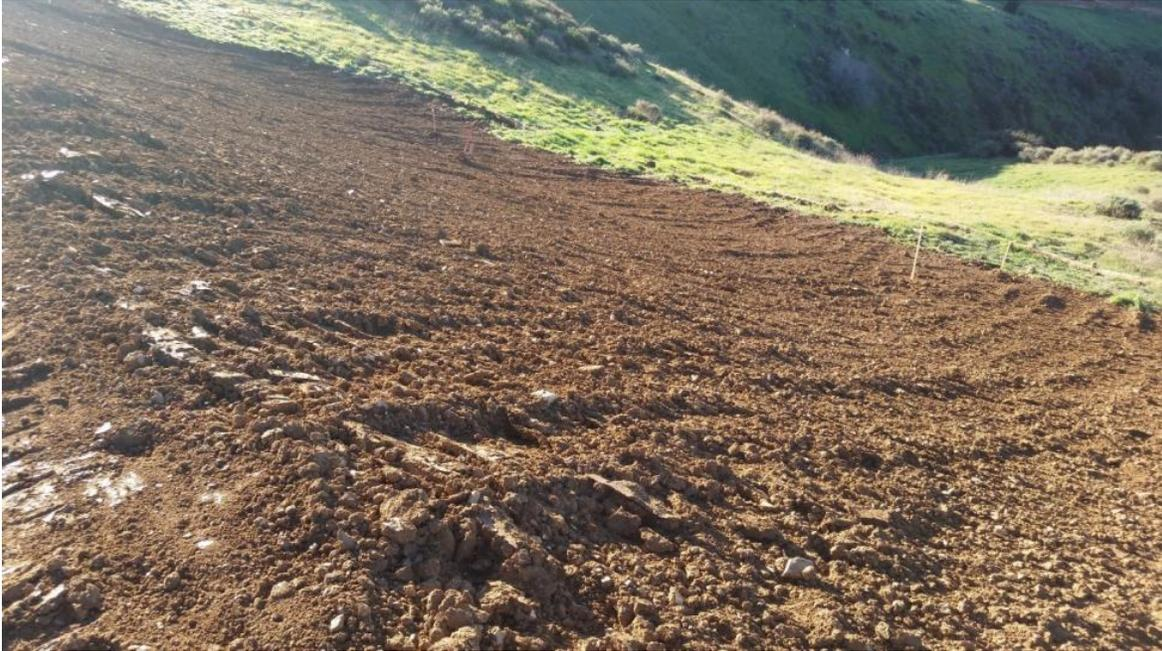
Photo 3: Provide cover for inactive slope and place fiber rolls every 10 ft. and trench in fiber rolls at the Natural Substation, February 9, 2015
