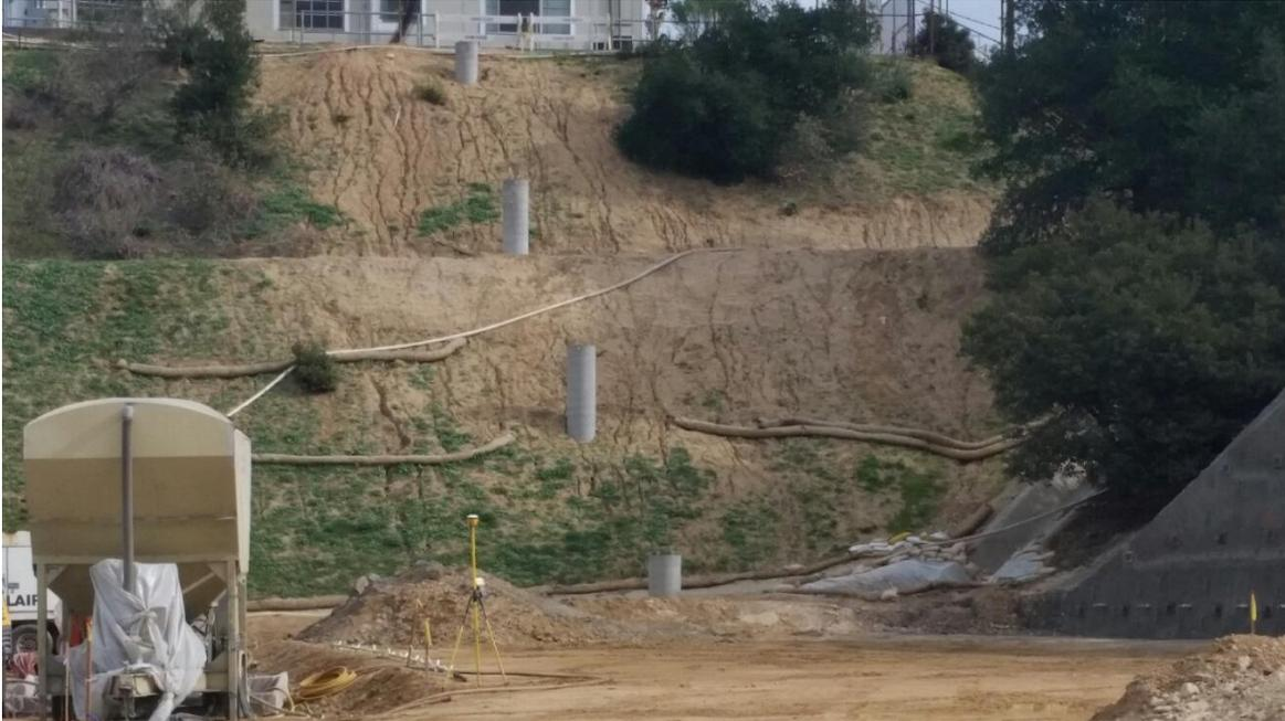
Photo 7: Provide either chemical or mechanical cover for inactive slopes at the Central Compressor Station, January 26, 2015
