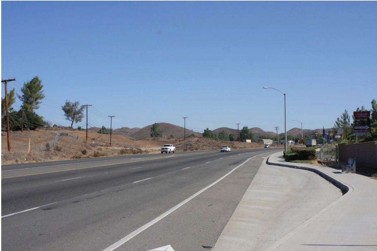
2. Highway 74 at Allan Street looking north (Segment 2)
