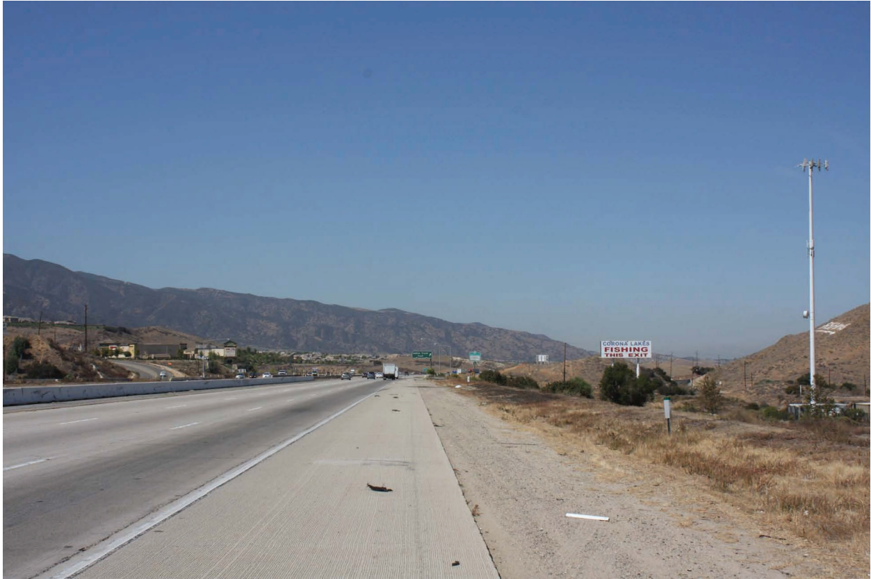
9. Interstate 15 looking northwest (Segment 7 crossing)
