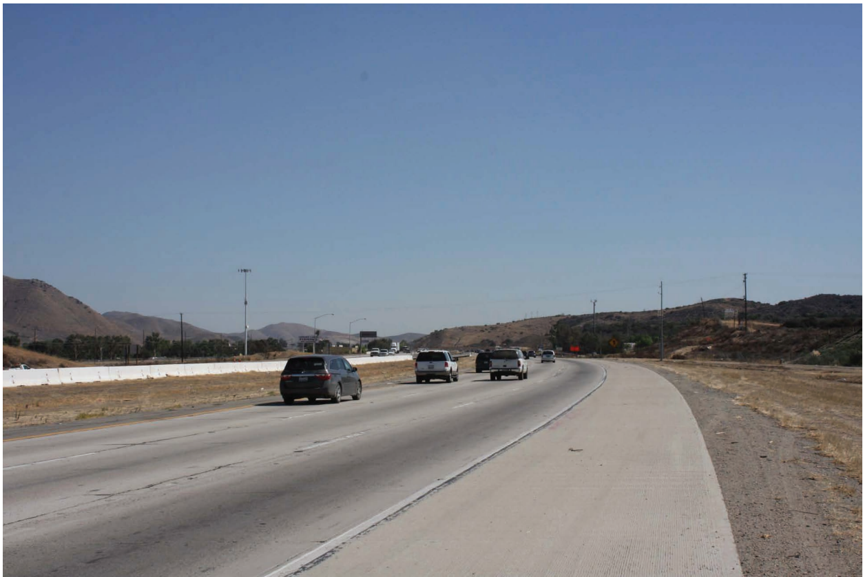
10. Interstate 15 at Indian Truck Trail looking southeast (Segment 7 crossing)
