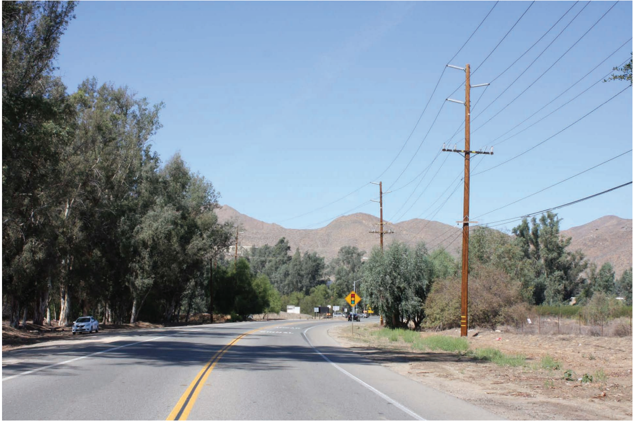
7. Lake Street near Temescal Canyon Road looking north (Segment 5)
