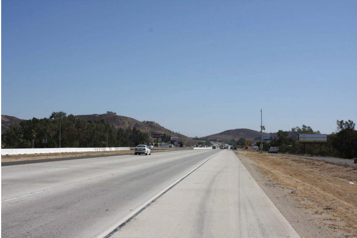
4. Interstate 15 near Central Avenue looking southeast (Segment 3 - 3rd Street crossing)
