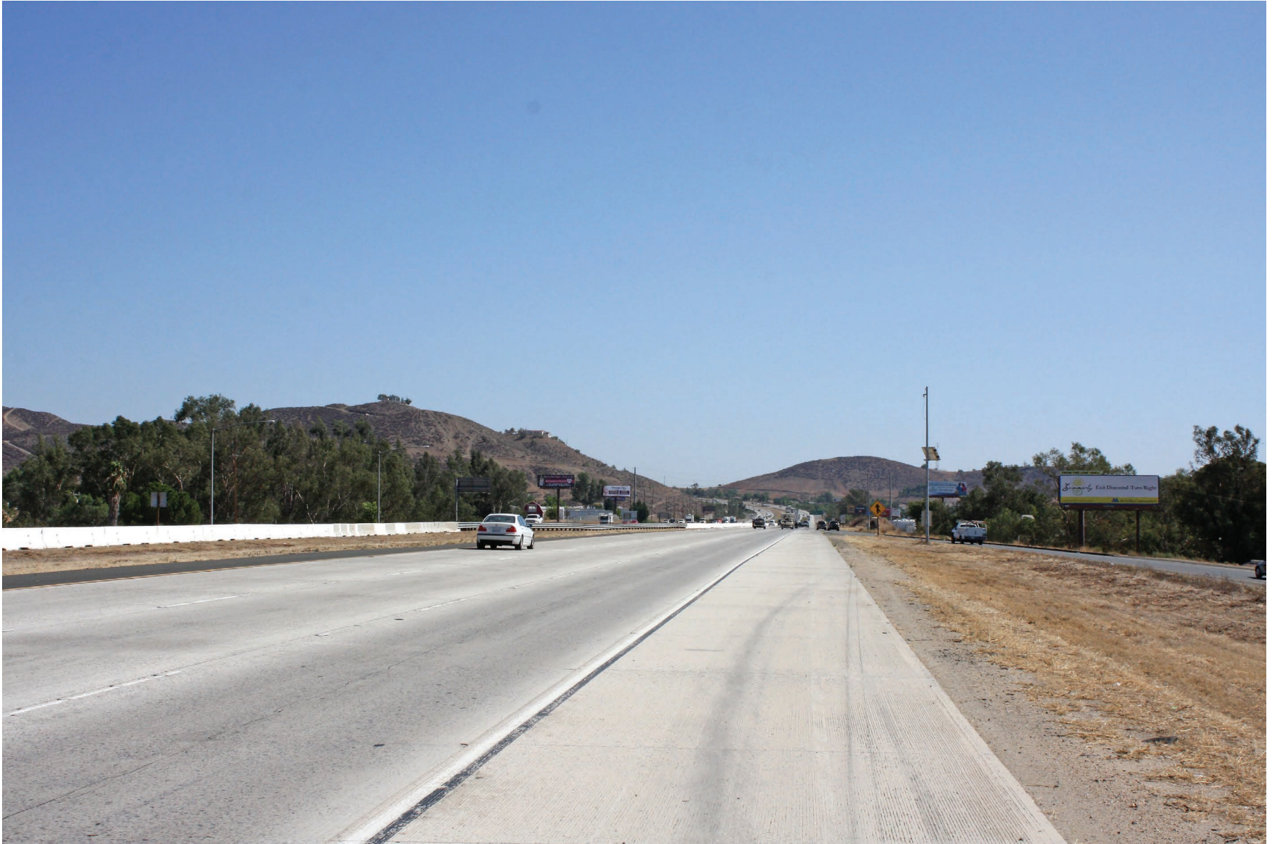
Existing View from Interstate 15 near Central Avenue looking southeast
