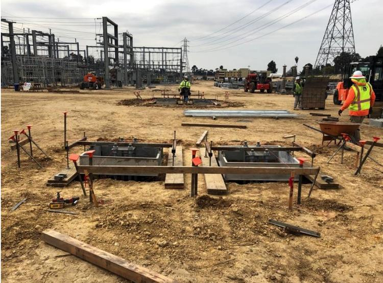
A wide-angle photograph of a construction site. In the foreground, there are two rectangular concrete foundation forms supported by wooden beams and red plastic chairs. The ground is dirt and sand. In the background, there are steel structures for a switchrack, utility poles, and a large transmission tower under a cloudy sky. Several workers in high-visibility vests are visible. | Photo 6 – Foundation work within the 220-kV switchrack area. Photo facing west. |
