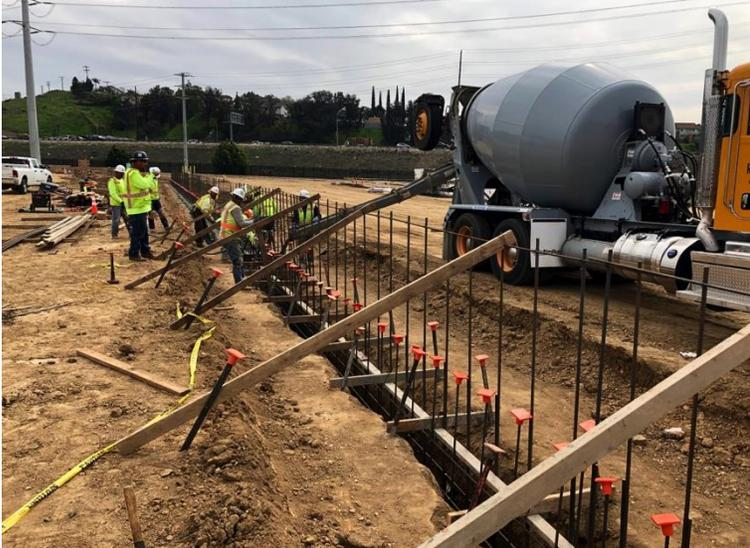
A photograph showing a concrete mixer truck at a construction site. The truck is positioned next to a long, narrow concrete formwork structure. Rebar is visible within the formwork. Several workers in high-visibility vests are standing nearby. The background shows a dirt area, utility poles, and a green hillside under a cloudy sky.                                                | Photo 7 – Pouring foundation for the interior wall. Photo facing south.         |
