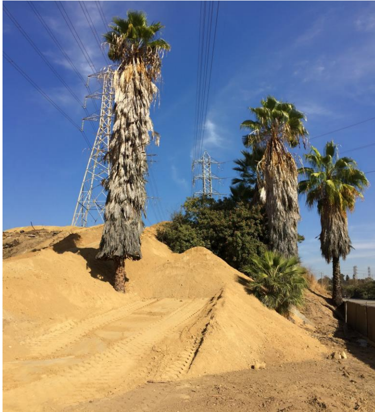
Photo 3: A soil stockpile that had been placed within a Kiewit work area on 12/4/2017 prior to a pre-construction clearance sweep, impacting adjacent Mexican fan palms and a Brazilian pepper tree (Photo by SCE; FRED Incident ID #000051).
