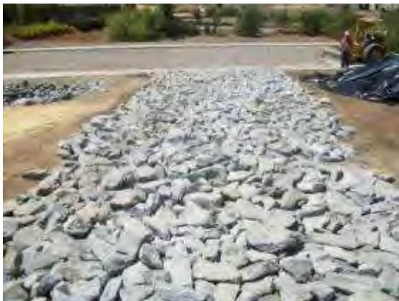
Effective large angular material
