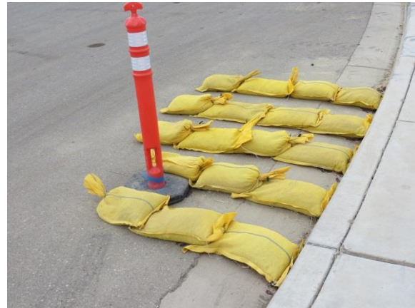
Runoff and sediment/perimeter control
