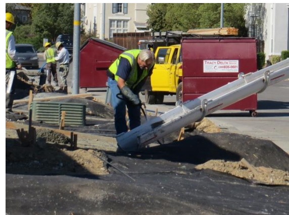
Concrete placement
