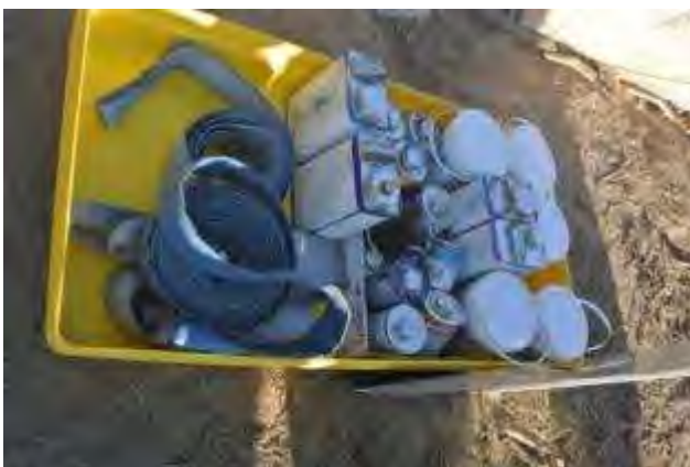
Properly contained in secondary containment
