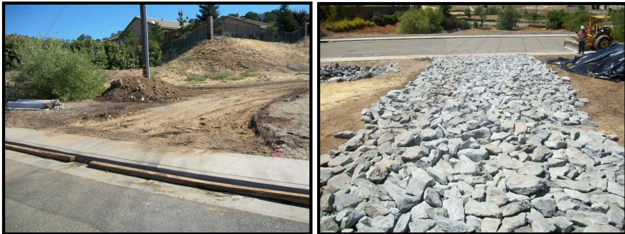
Construction entrance/exit before and after installation.
