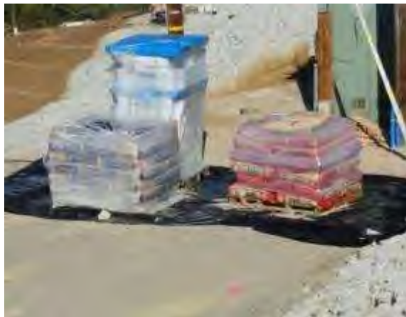
Properly wrapped in plastic, on pallet, and on plastic
