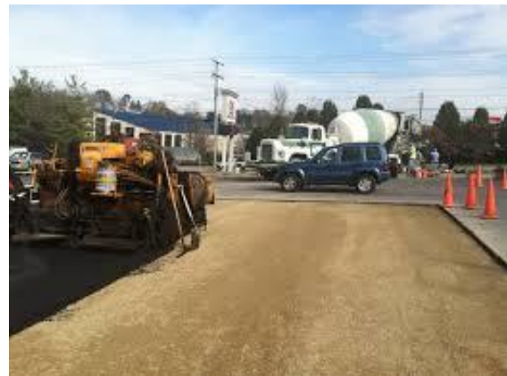
Active Asphalt Paving
