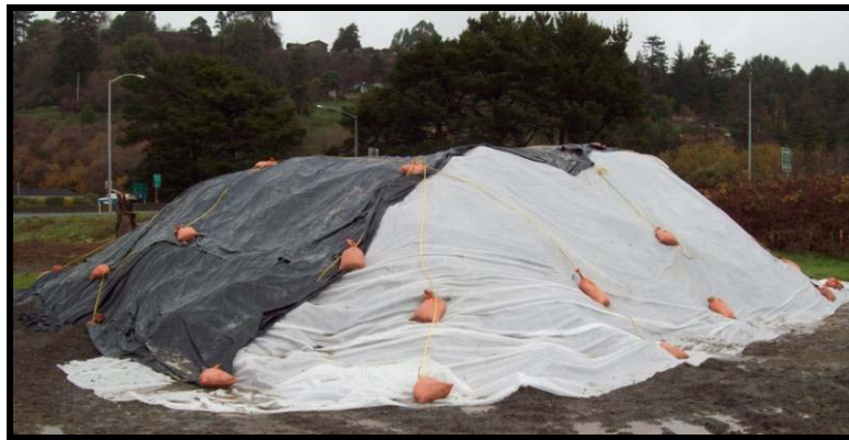
Proper securing of plastic sheeting.
