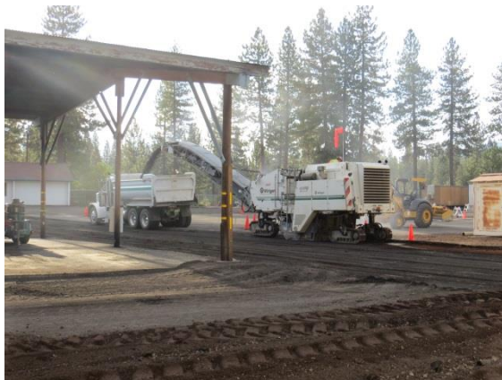
Grinding of existing asphalt
