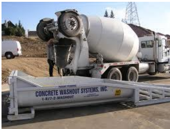
Concrete washout system
