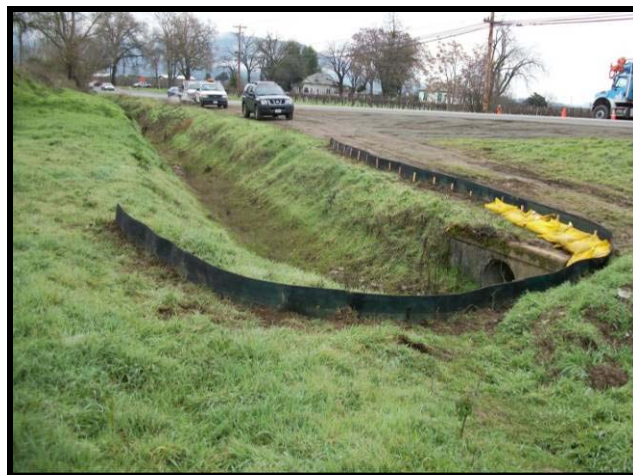
Silt fence reinforced with gravel bags.
