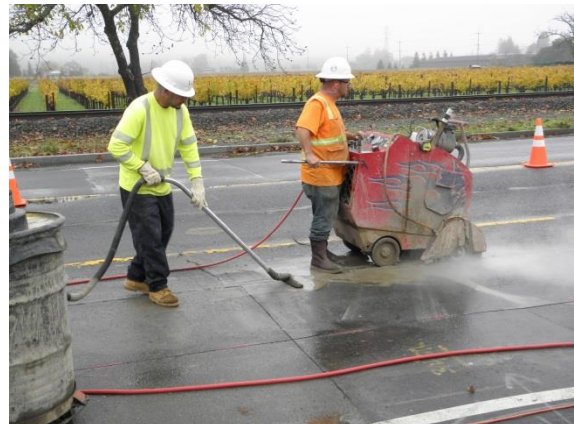
Sawcutting in preparation of excavation
