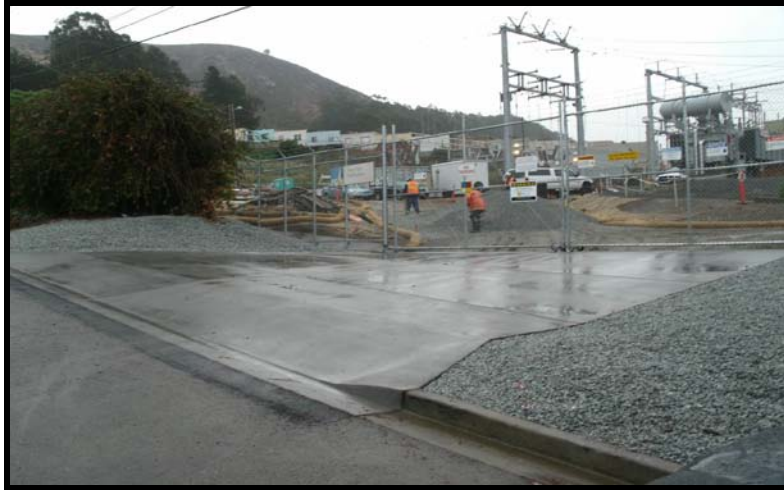
Clean and well maintained construction entrance/exit.
