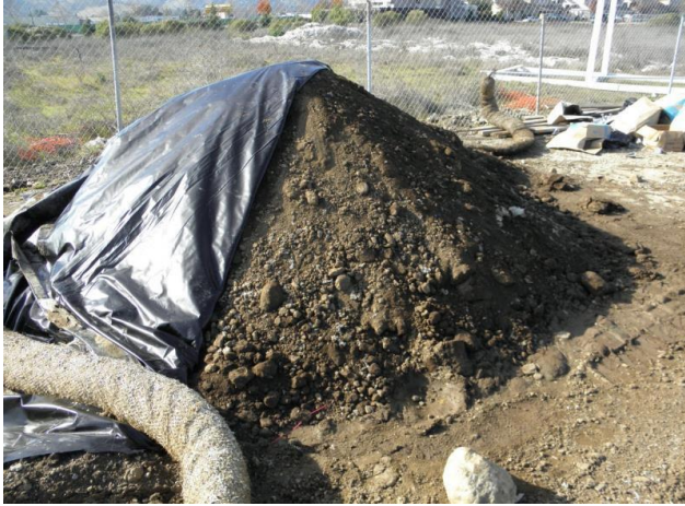
Figure 1. Cover pulled back for access during use
