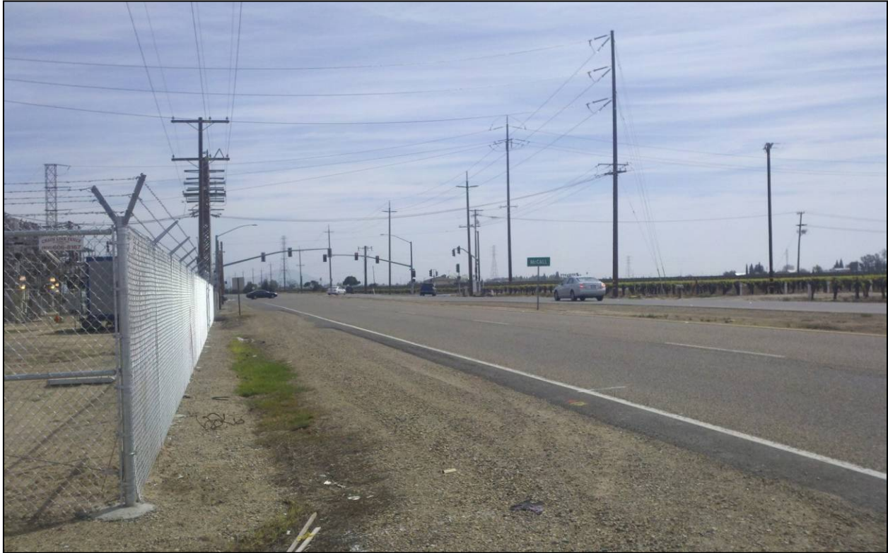
Figure 3.4-4 Urban/Semi-Urban – View east toward the intersection of East Jensen Avenue and South McCall Avenue immediately south of the existing Sanger Substation (to left side of photograph). Photograph dated March 30, 2012.
