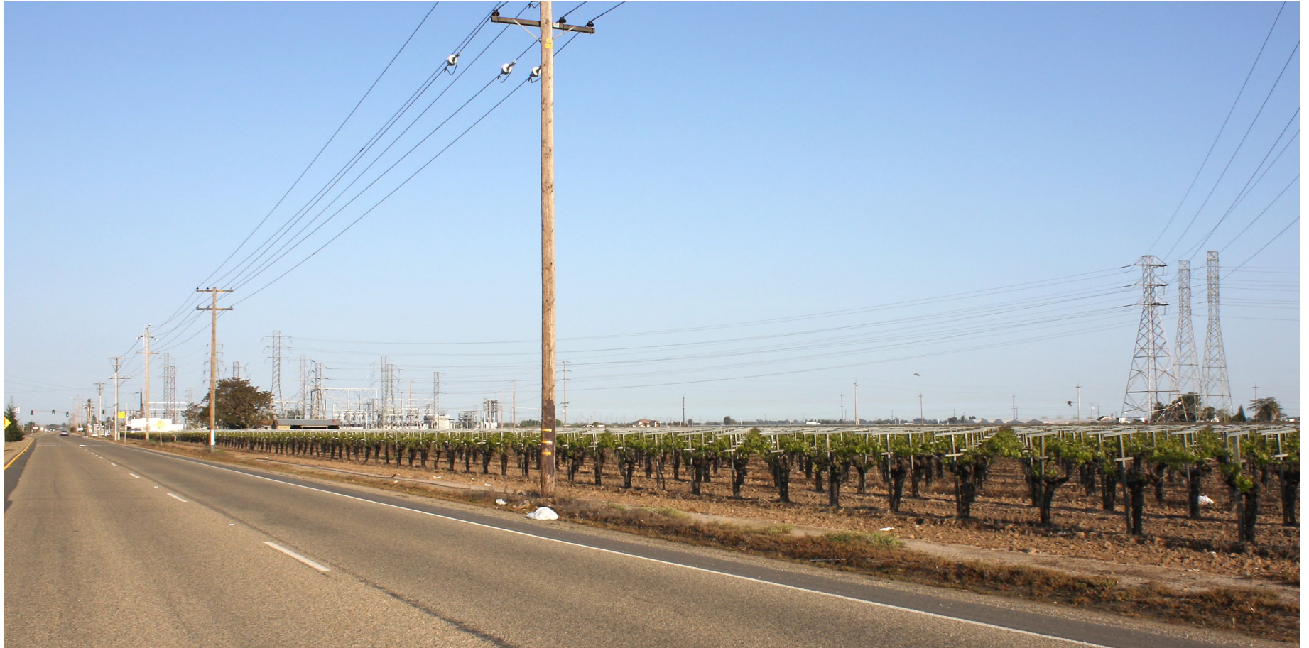
Existing View from East Jensen Avenue looking Northwest (VP 7)
