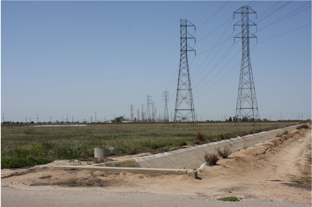
13. South Dockery Avenue looking southwest
