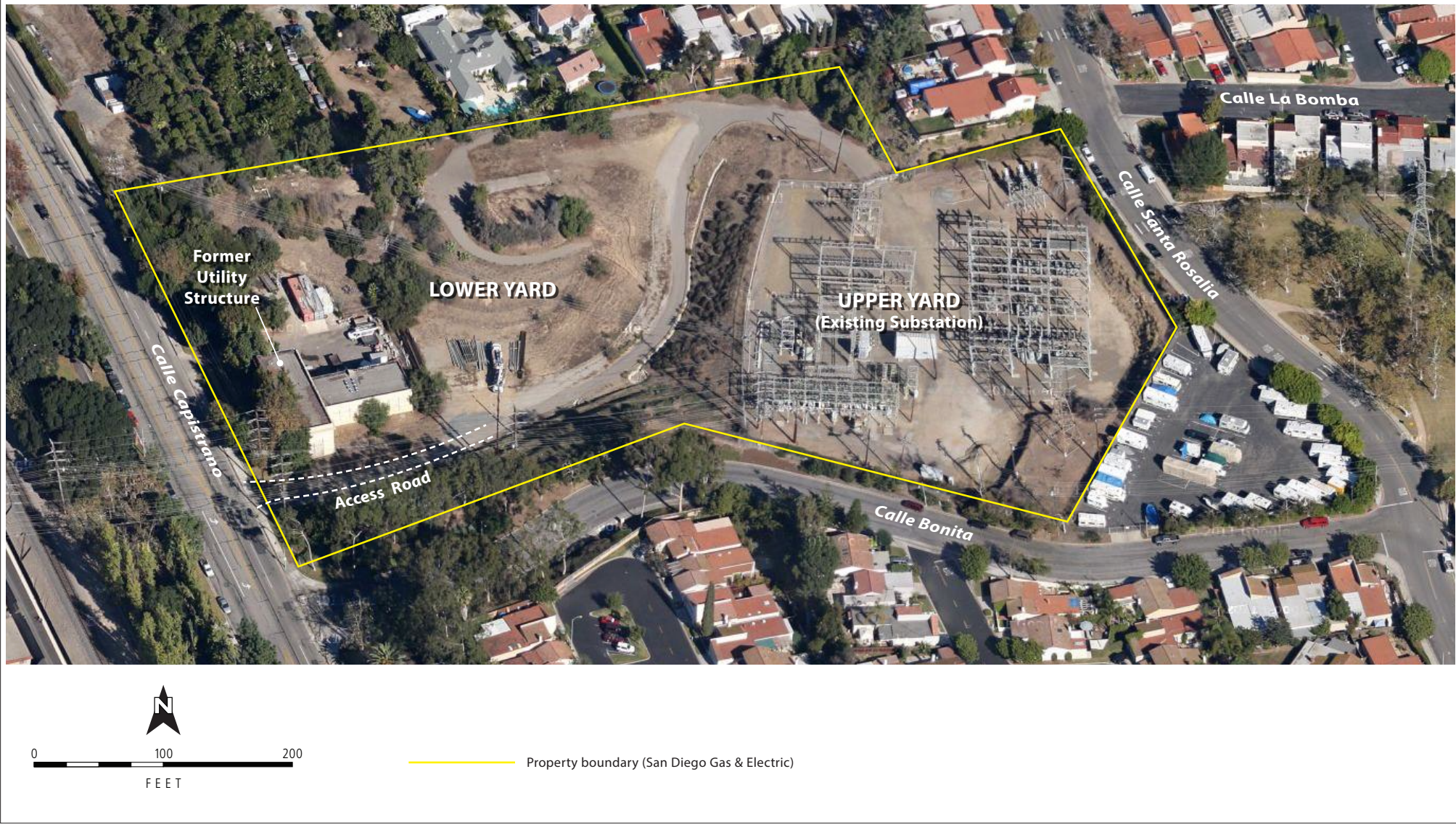
Figure 2-3 Capistrano Substation Site South Orange County Reliability Enhancement Project
