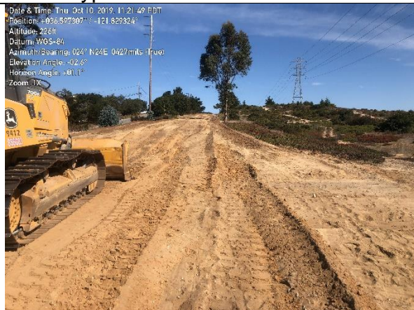
Photo 4. Offsite spoils site (Mescal Street)
