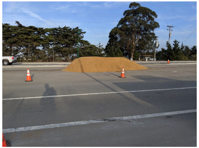
temporary soil depot in median on general jim Moore, facing W
