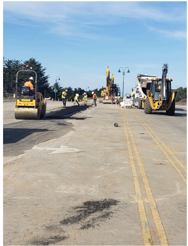
install asphalt end of the day
