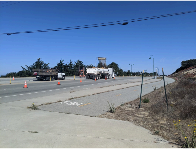
cover over soil transport truck for dust control, facing NW
