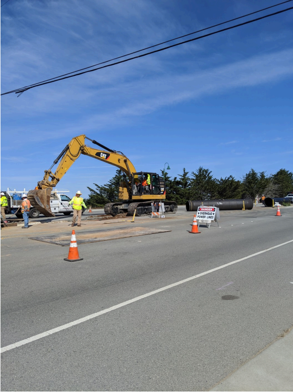
Sign placed for overhead wires
