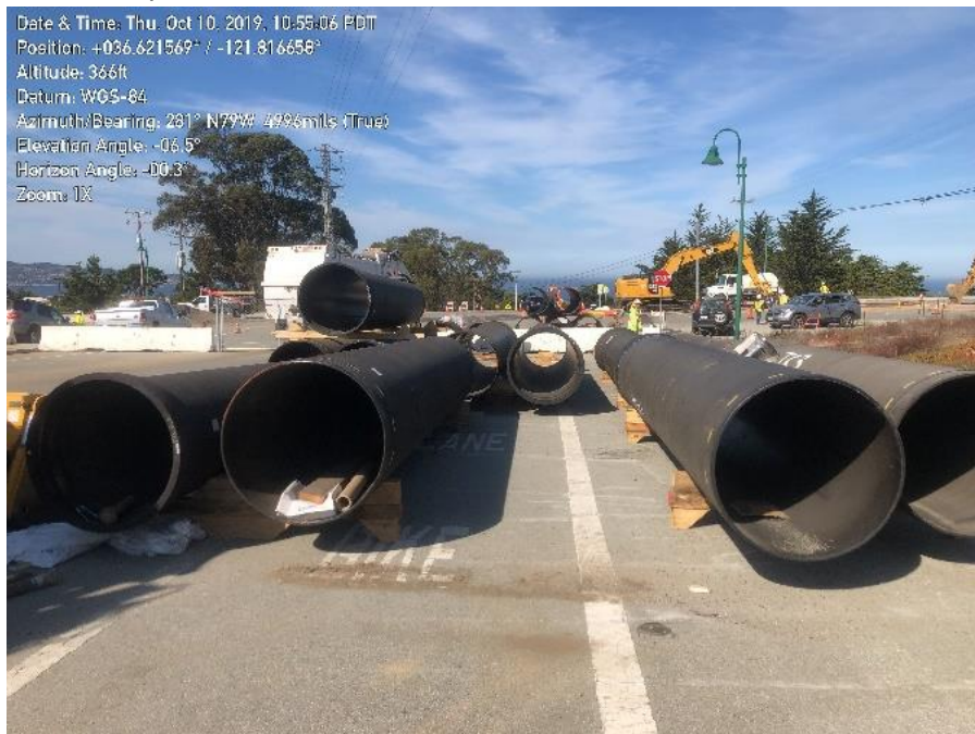
Photo 2. Equipment and materials staging on Eucalyptus Road
