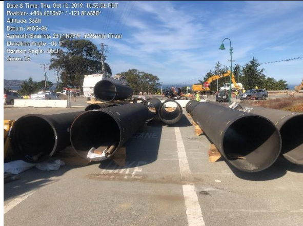
Photo 2. Equipment and materials staging on Eucalyptus Drive.
