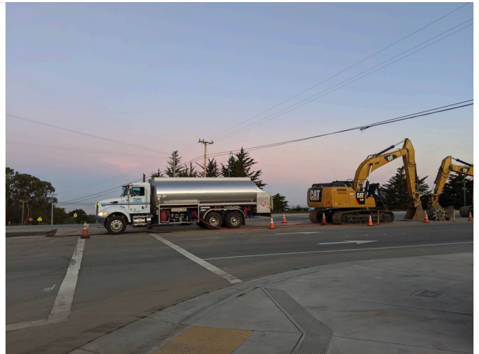
fueling of equipment in center of median, facing NW
