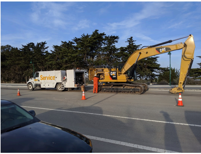
servicing of backhoe in median, facing SW
