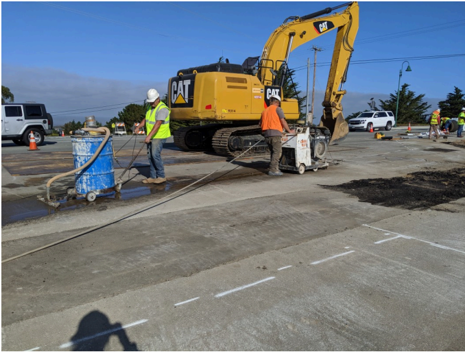
Additional saw cutting
