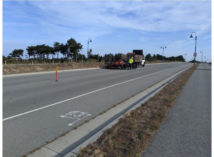
establishing traffic diversion along general Jim Moore, facing N
