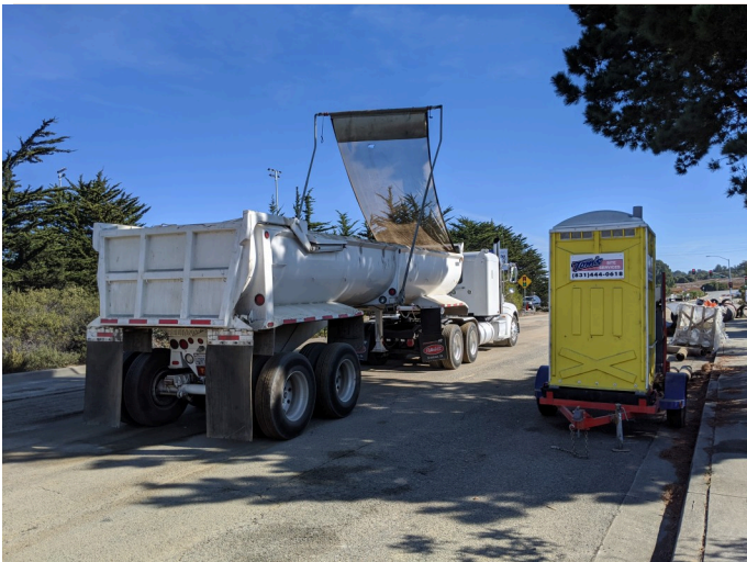
dust mitigating cover over soil transportation truck on Lightfighter, facing E
