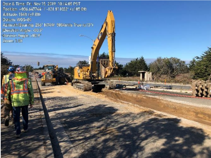
Photo 1. Trench excavation on Lightfighter Drive
