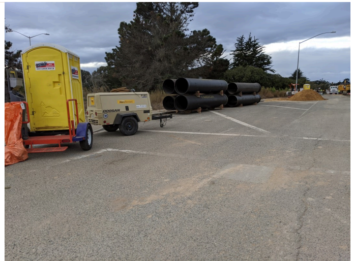
staging in unplanned area on turnout on Lightfighter drive, facing SW
