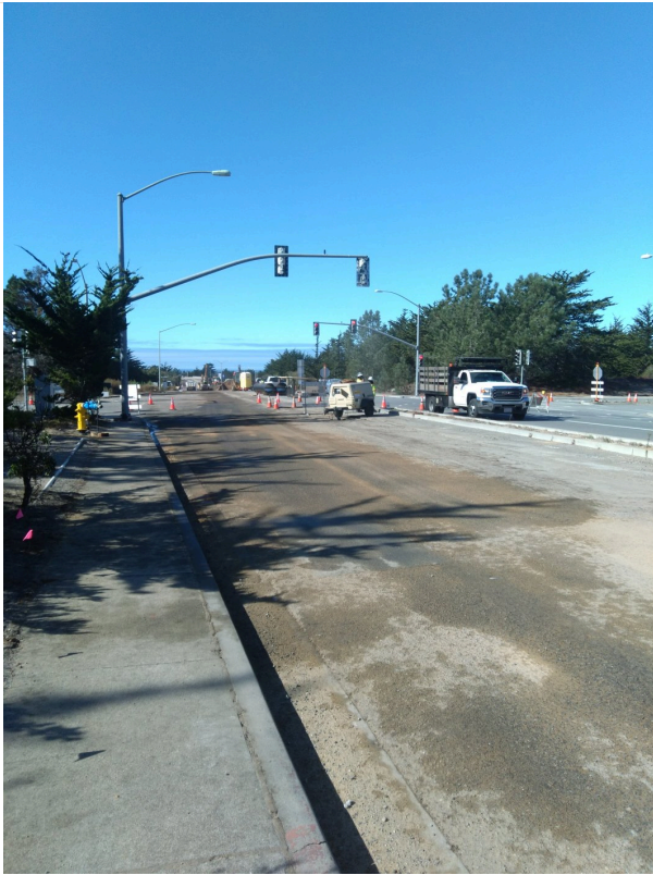
Garney installing pipe along Light Fighter
