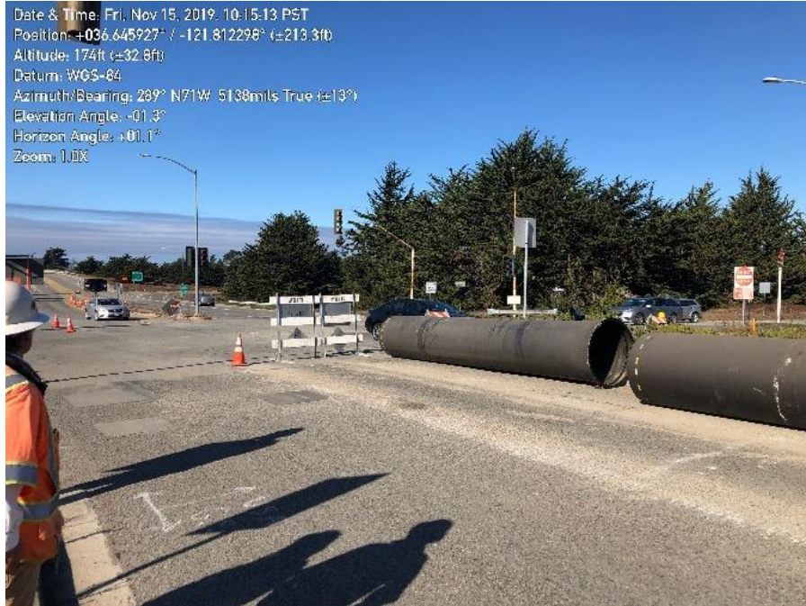
Photo 3. End of work area on Lightfighter Drive at 1 st Street
