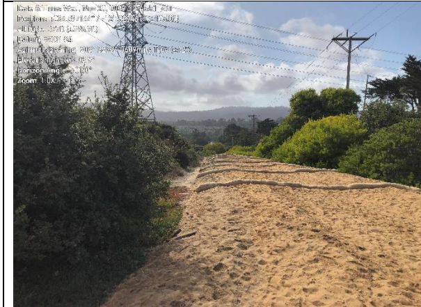
Photo 3. Straw wattle in place at Mescal Street spoils disposal area
