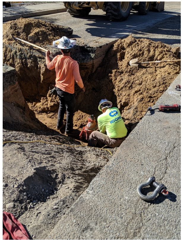
Air Valve was installed at STA 25+27
