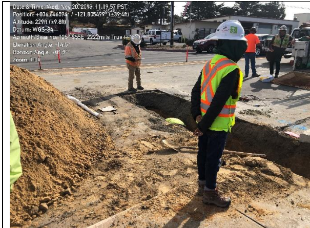
Photo 1. Air valve installation on General Jim Moore Blvd.
