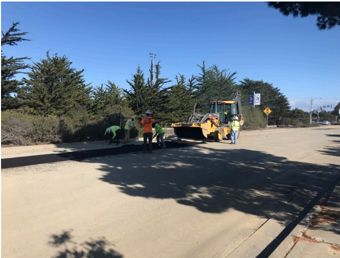
re paving Light Fighter Ave
