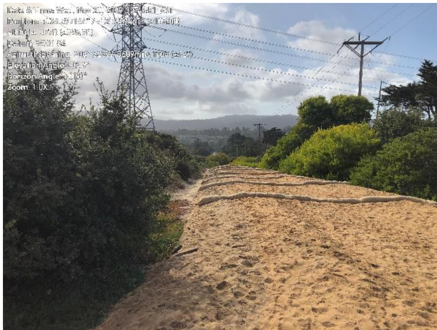
Photo 4. Straw wattle in place at Mescal Street spoils disposal area
