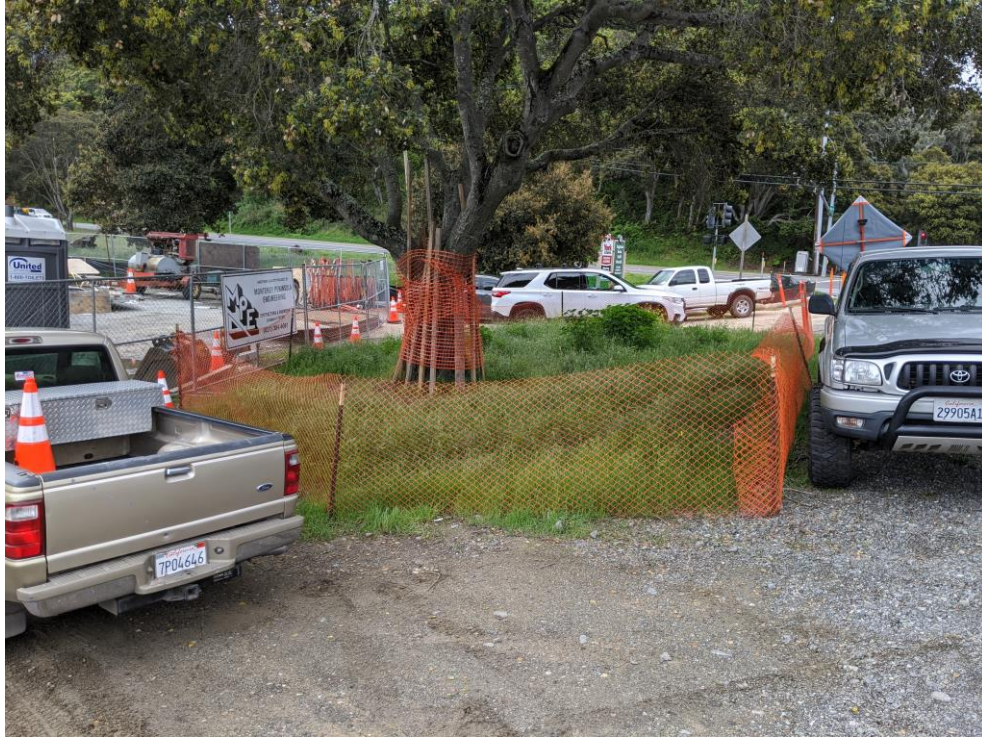
Photo 3. Intact ESA fencing around protected coast live oak tree adjacent to staging area. (3-27-2020)
