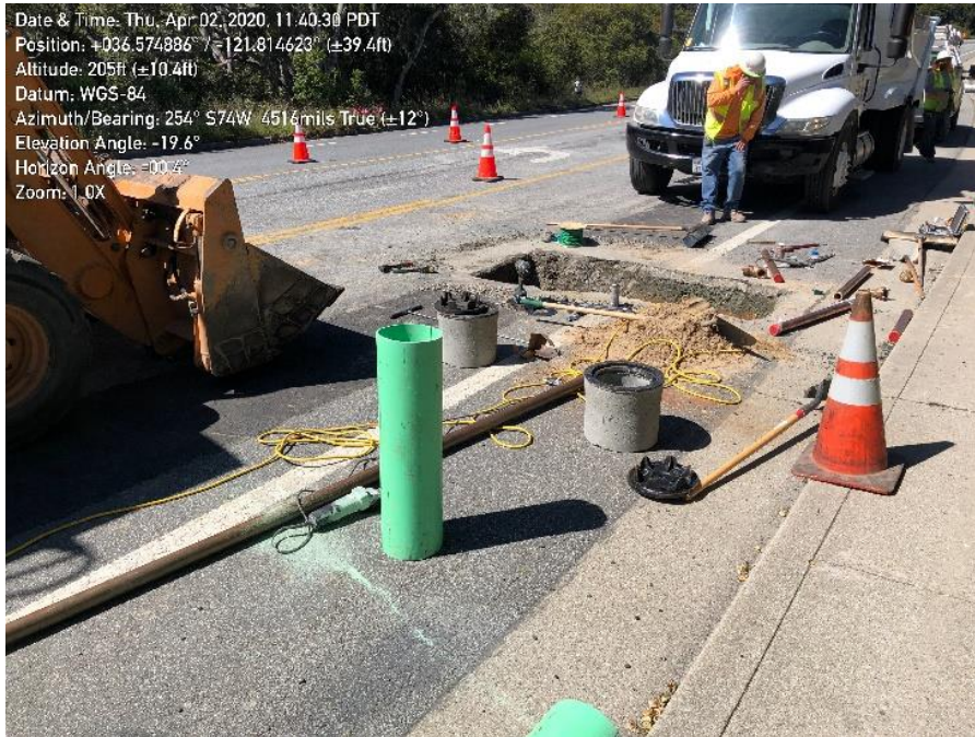
Photo 1. MPE installation of blow off valves on Lower Ragsdale Drive..
