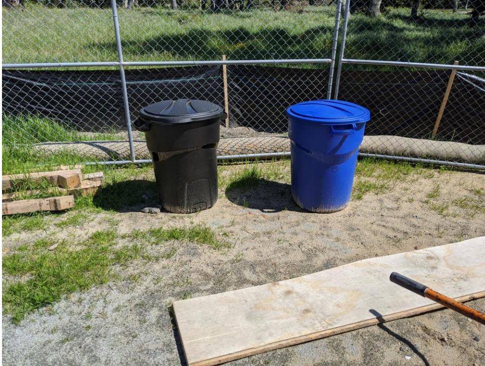
Photo 5. Confirmed additional trash receptacles at staging area. (3-30-2020)
