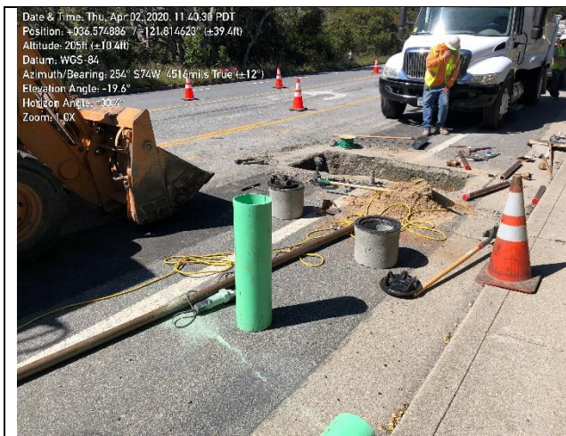
Photo 1. MPE installation of blow off valves on Lower Ragsdale Drive.
