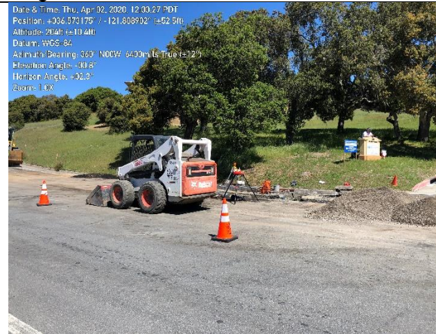
Photo 4. MPE installation of blow off valves on Wilson Road.
