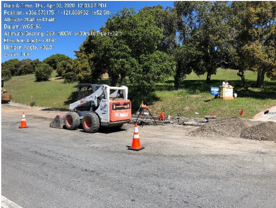
Photo 4. MPE installation of blow off valves on Wilson Road.
