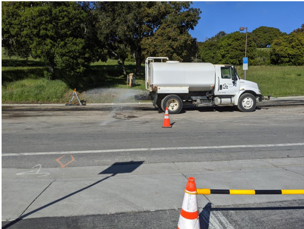
Photo 8. Minimal water usage on roadway to limit dust along alignment. (3-31-2020)
