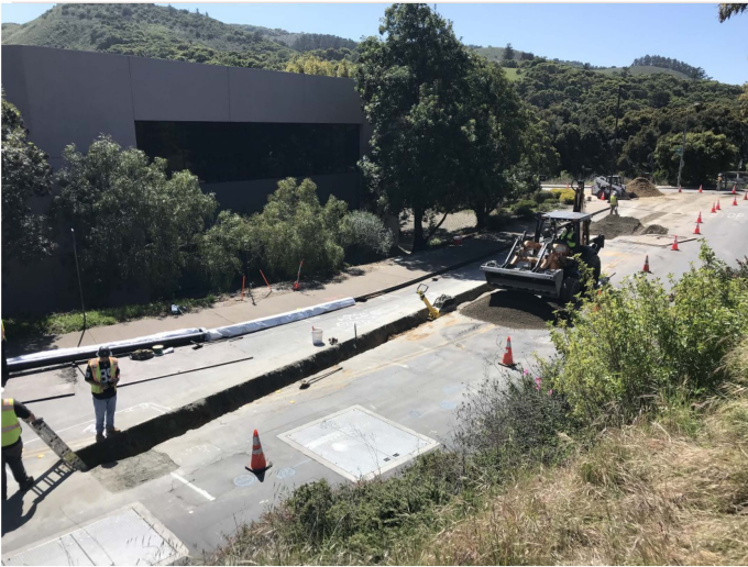
pipeline installation along Blue Larkspur Ln
