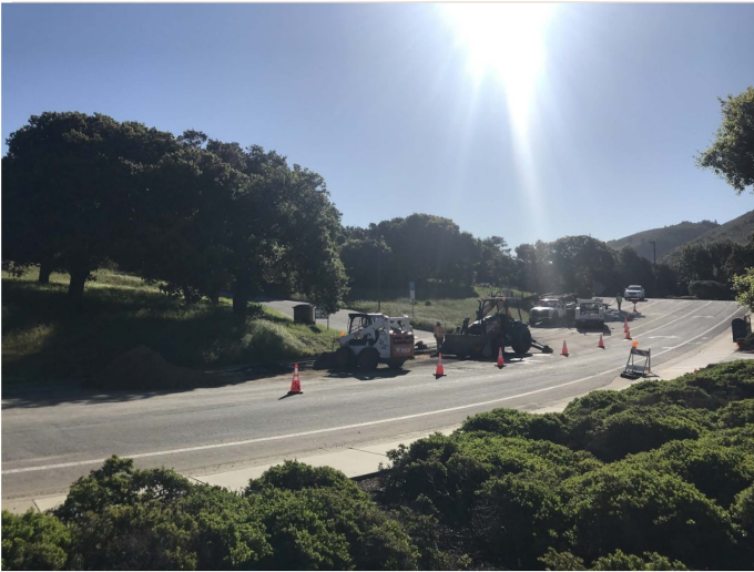
installation of blowoff along Wilson Rd
