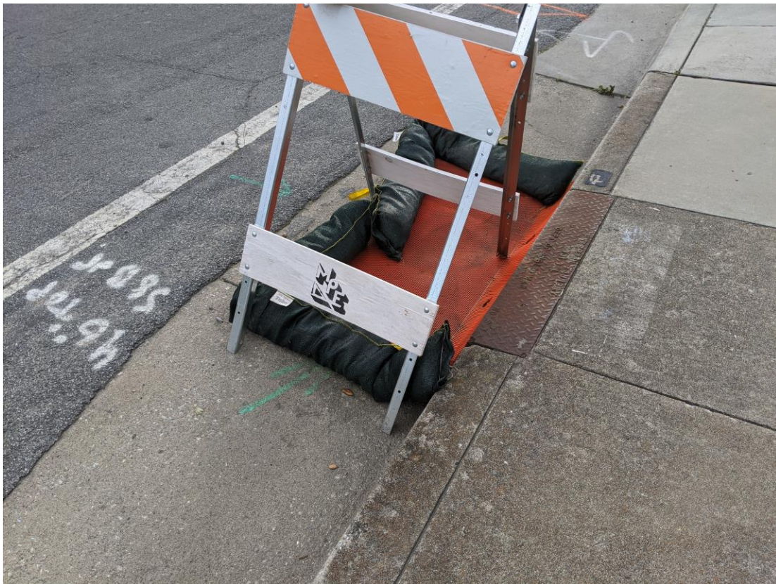
Photo 2. Confirmed integrity of stormwater drain protection adjacent to construction. (3-27-2020)
