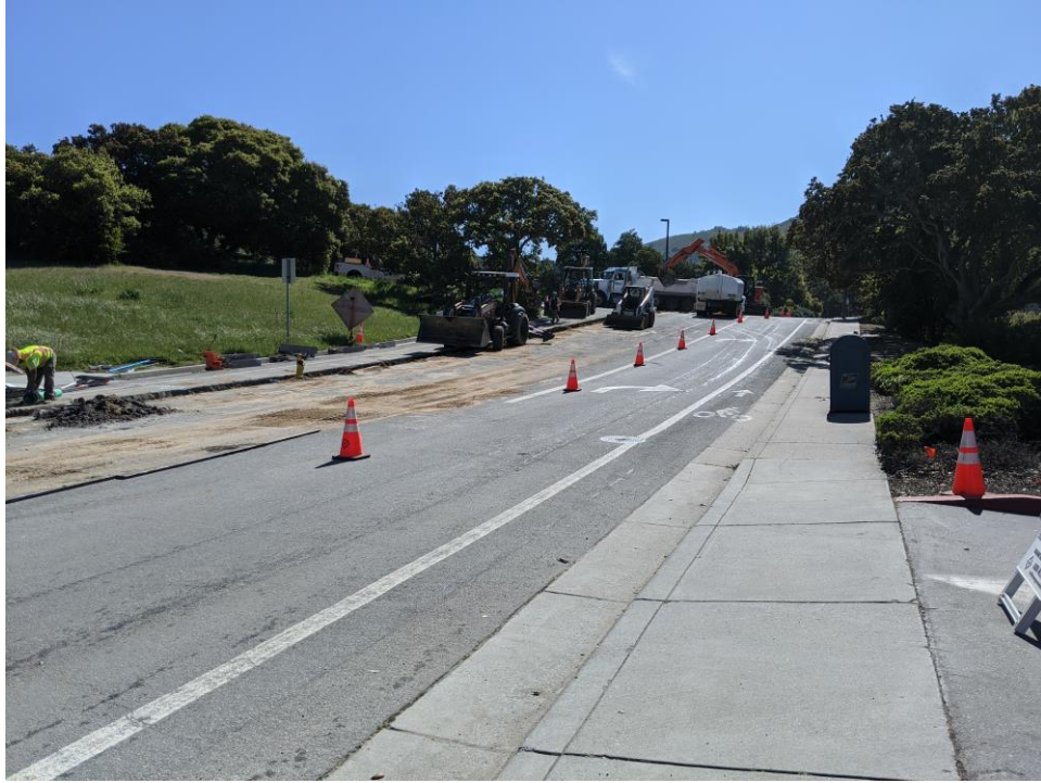
Photo 7. Relocated traffic cones to allow for additional space for traffic to avoid coast live oak tree. (3-31-2020)
