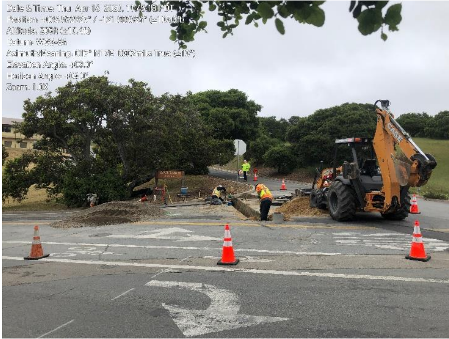
Photo 1. MPE installation of air release valve on Wilson Road.
