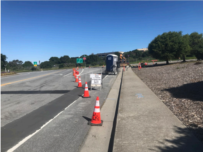
installation of blowoff at the intersection of Lower Ragsdale and Ragsdale
