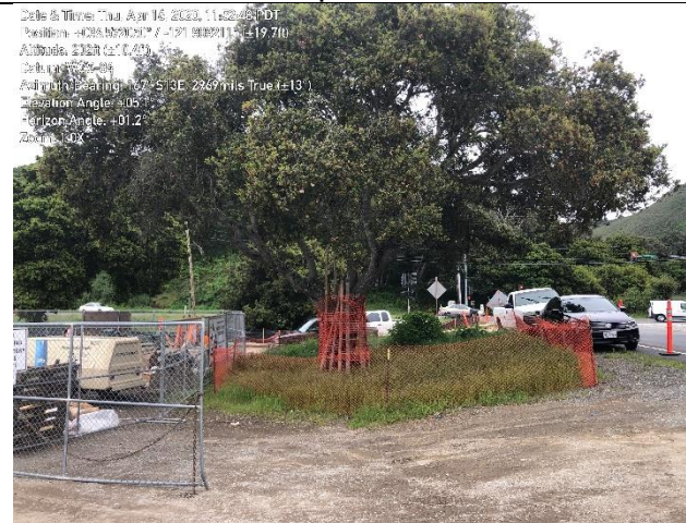
Photo 4. Tree protection and silt fence at staging area in good condition.
