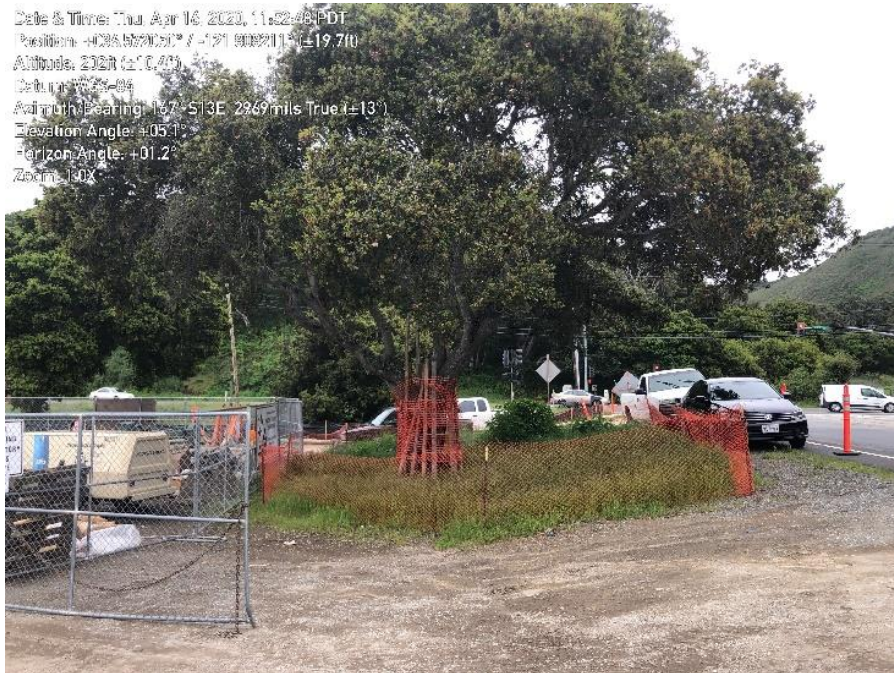
Photo 4. Tree protection and silt fence at staging area in good condition.
