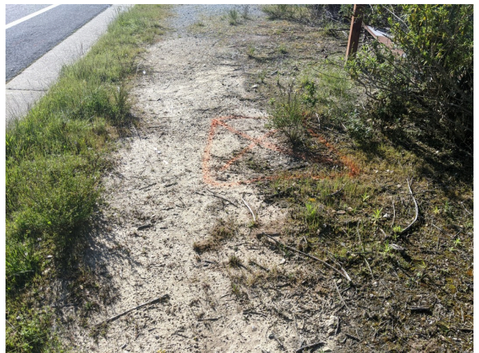
secondary view of final ARV site on Lower Ragsdale ct
