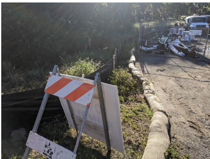
secondary view of intact silt fencing surrounding staging area
