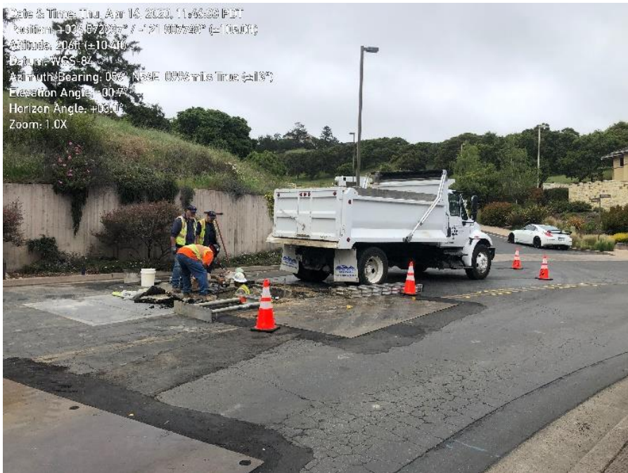
Photo 2. MPE installation of air release valve on Blue Larkspur Lane.
