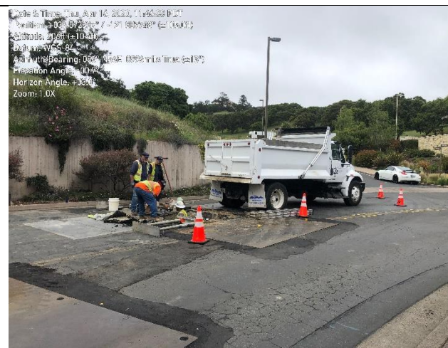
Photo 2. MPE installation of air release valve on Blue Larkspur Lane.
