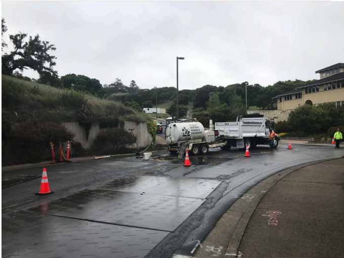
installation of blow off along Blue Larkspur Ln
