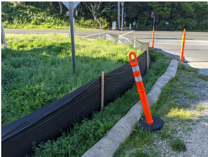
View of intact silt fencing surrounding staging area
