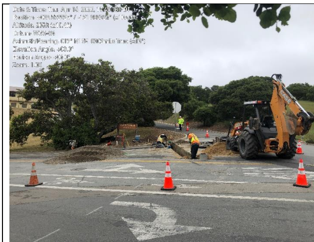
Photo 1. MPE installation of air release valve on Wilson Road.
