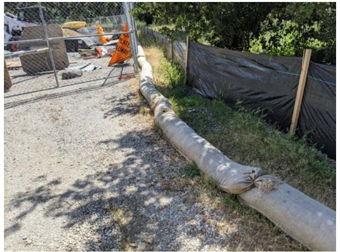
Infact silt fencing surrounding staging area.
