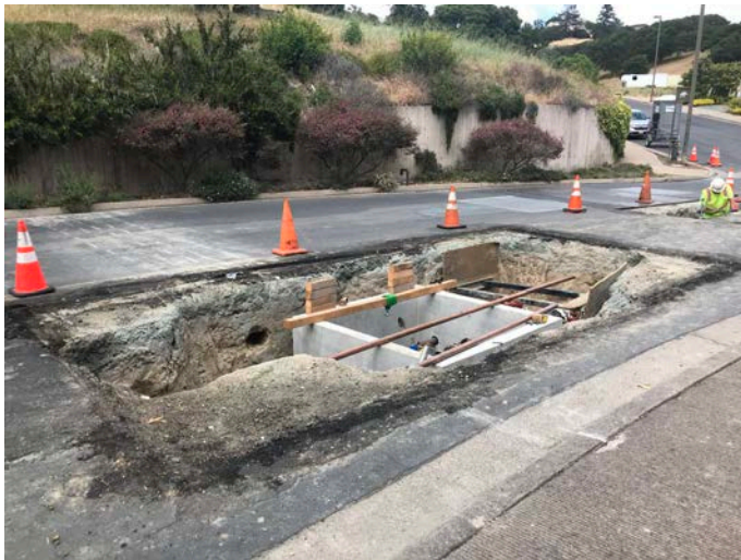
MPE Prepping and Pressure testing PRV along Blue Larkspur Ln
