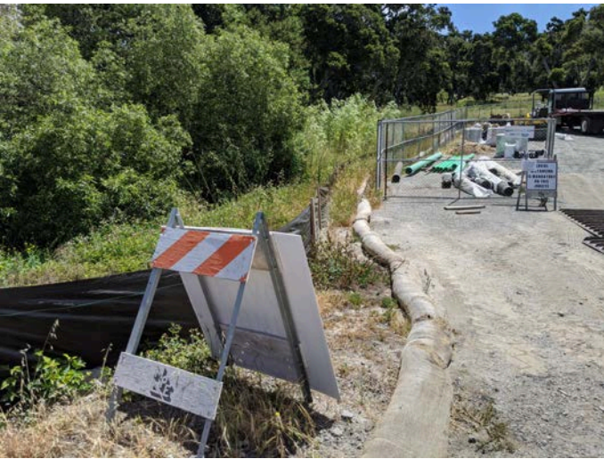
Infact silt fencing surrounding staging area.
