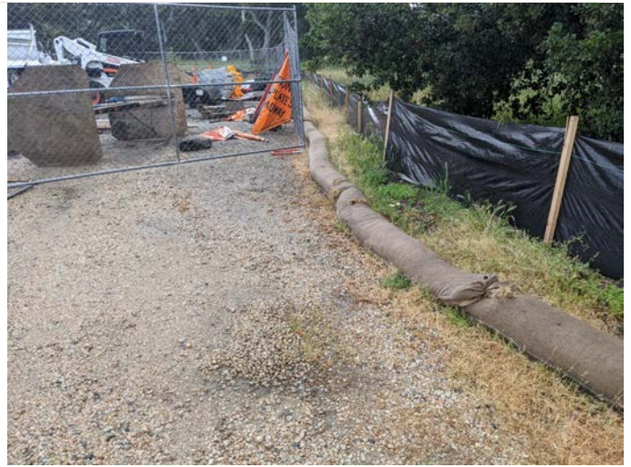
Intact silt fencing surrounding staging area.
