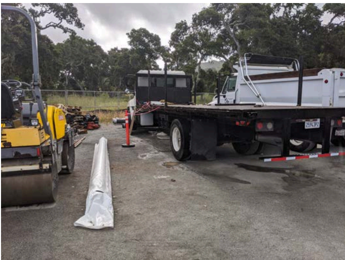
Intact protective flagging surrounding protected black phoebe nest within staging area.
