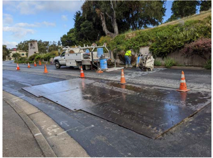
MPE installing backflow components on Blue Larkspur Lane.
