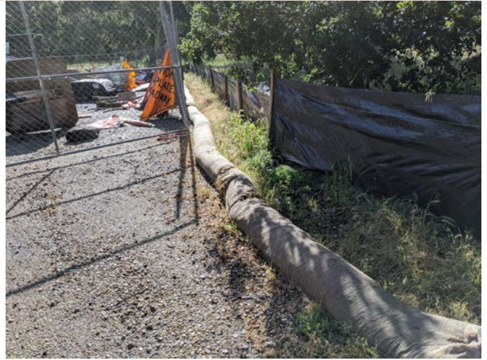
Intact silt fencing surrounding staging area.
