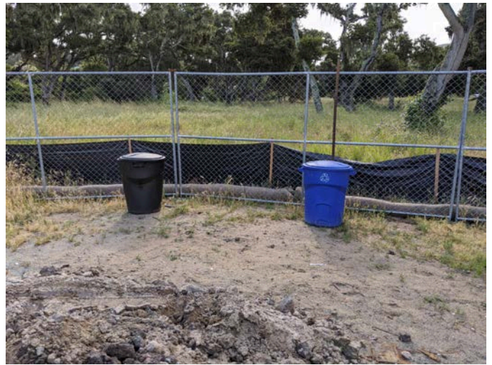
Emptied trash and recycling receptacles within staging area.
