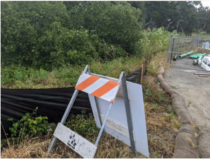
Intact silt fencing surrounding staging area.
