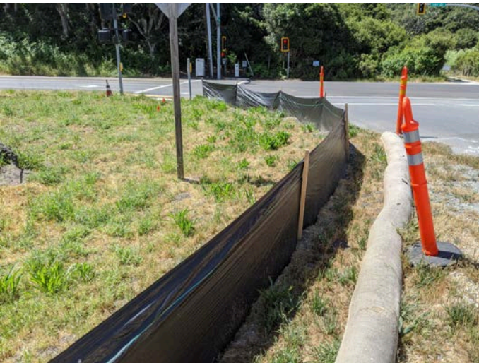
Infact silt fencing surrounding staging area.
