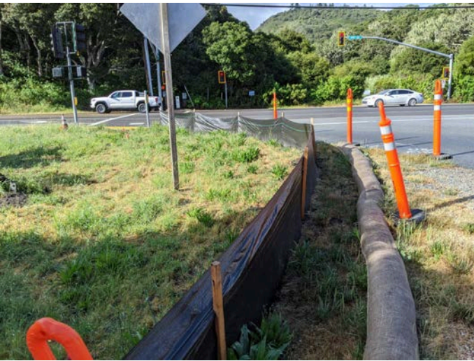
Intact silt fencing surrounding staging area.
