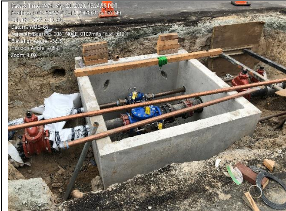
Photo 1. MPE excavation on Blue Larkspur Lane.
