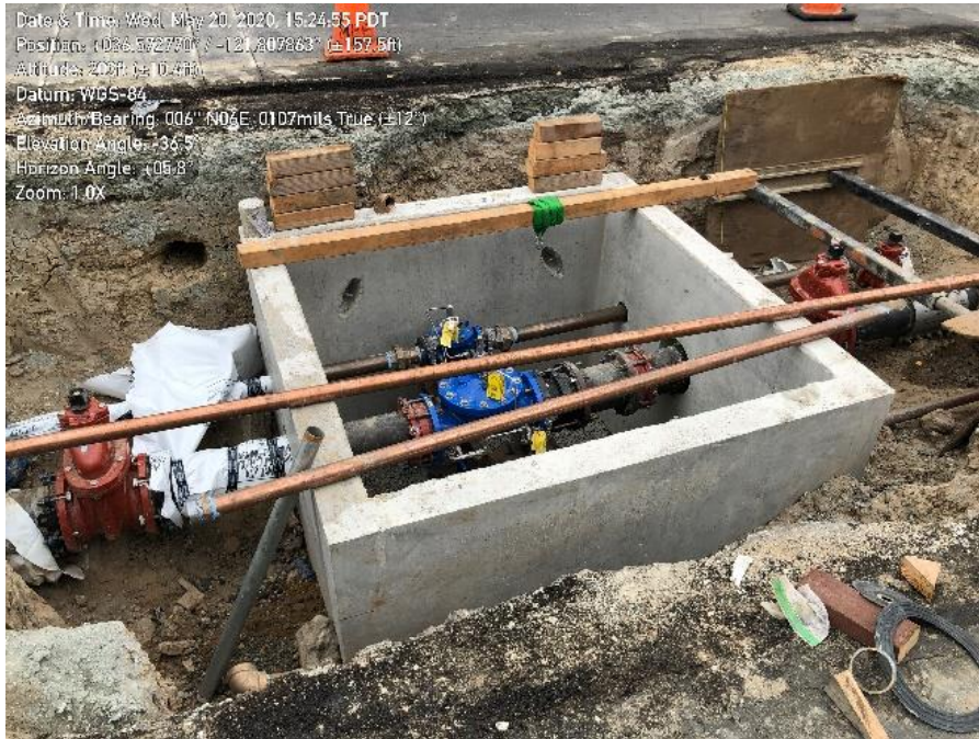
Photo 1. MPE excavation for installation of PRV components on Blue Larkspur Lane.
