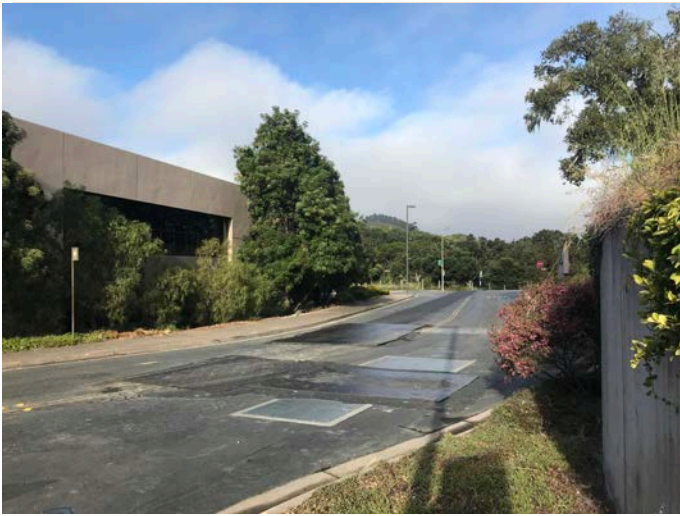
Construction site prior to the days activities.
