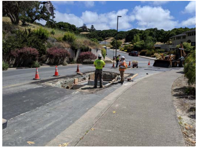
MPE installing PRV vault components on Blue Larkspur Lane
