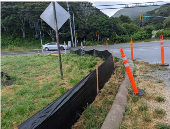
Intact silt fencing surrounding staging area.
