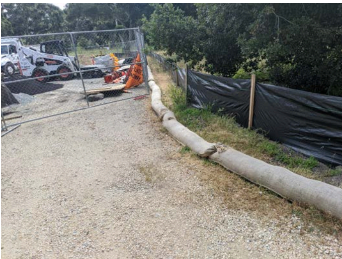
Intact silt fencing surrounding staging area.
