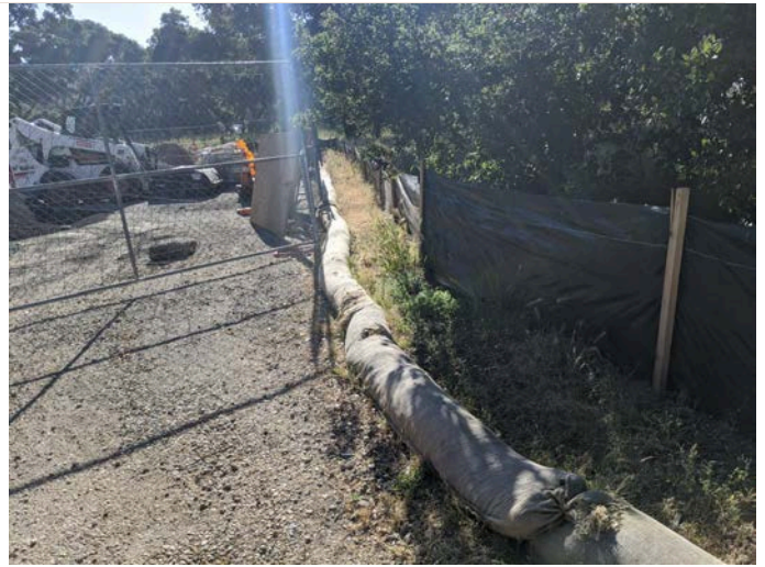
Intact silt fencing surrounding staging area.
