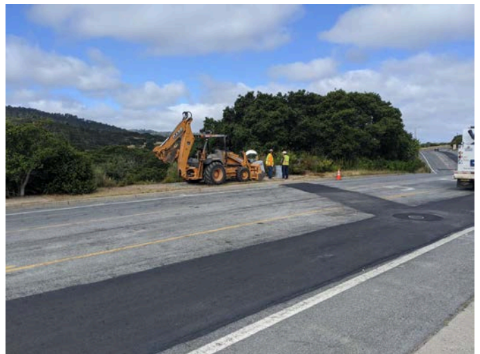
MPE installing protective cages around ARV valves on Lower Ragsdale Drive.
