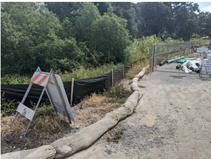
Intact silt fencing surrounding staging area.
