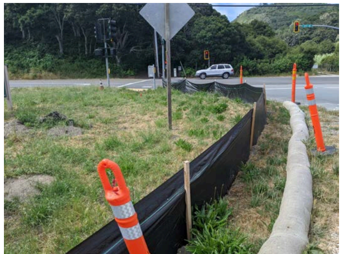
Intact silt fencing surrounding staging area.
