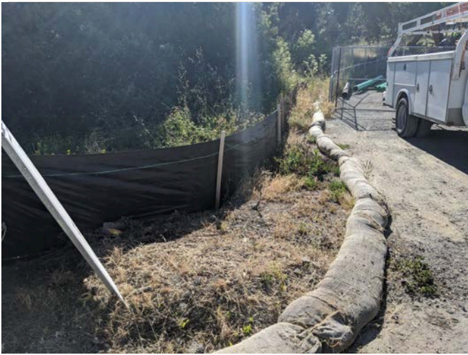
Intact silt fencing surrounding staging area.
