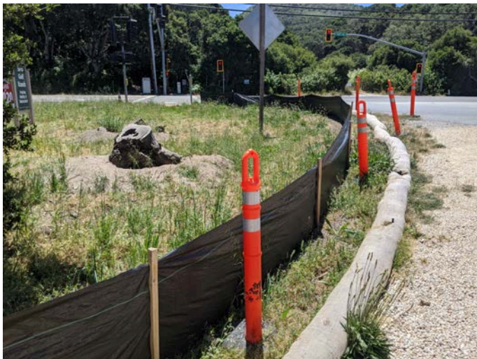
Intact silt fencing surrounding staging area.
