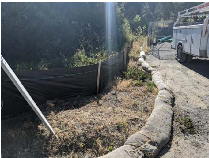
Intact silt fencing surrounding staging area.
