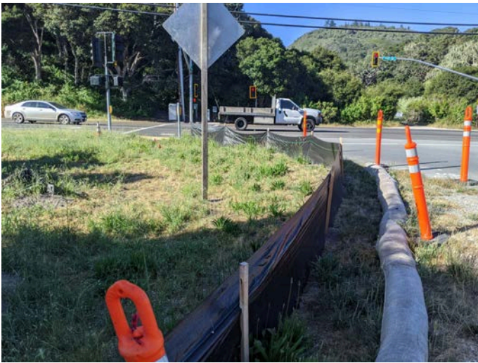
Intact silt fencing surrounding staging area.
