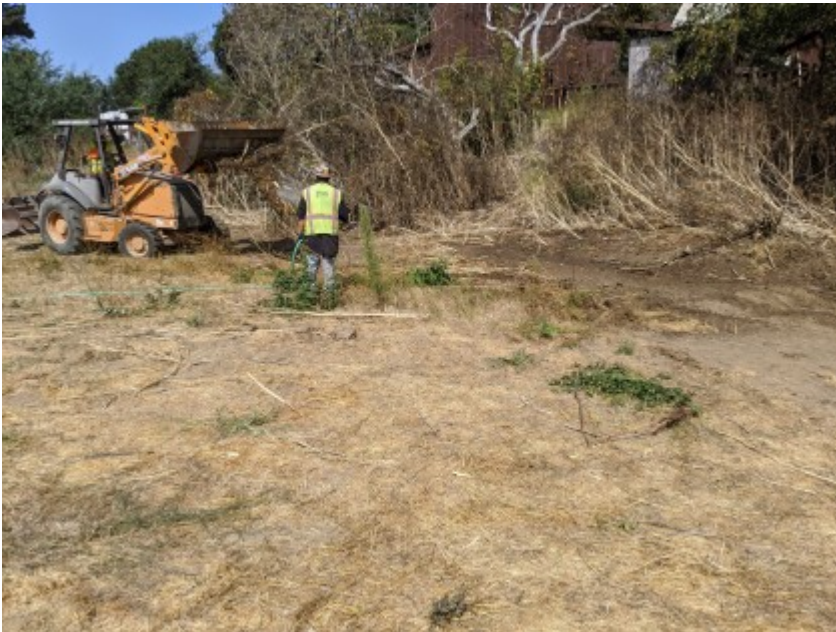
09/16/2020 - Initial vegetation clearing within limits of grading.
