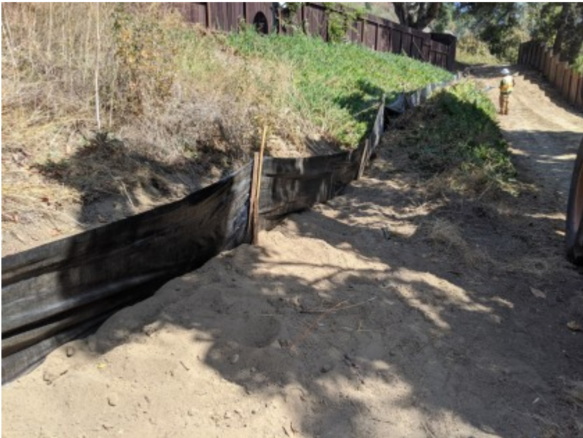
09/18/2020 - Completed silt fencing surrounding staging area and access route.
