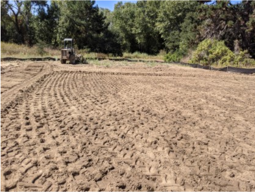
09/18/2020 - Graded and compacted area within construction site.
