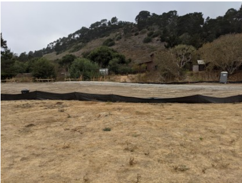
10/22/2020 - Intact exclusionary fencing surrounding construction area.
