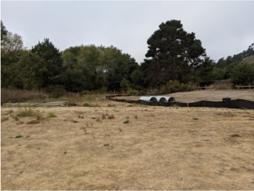
10/22/2020 - Intact exclusionary fencing surrounding construction area.
