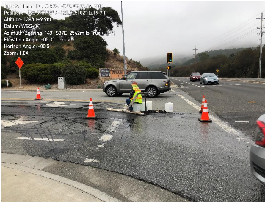
Photo 2. Ryan Ranch – Bishop Interconnection Improvements: Flushing activities on Ragsdale Drive.
