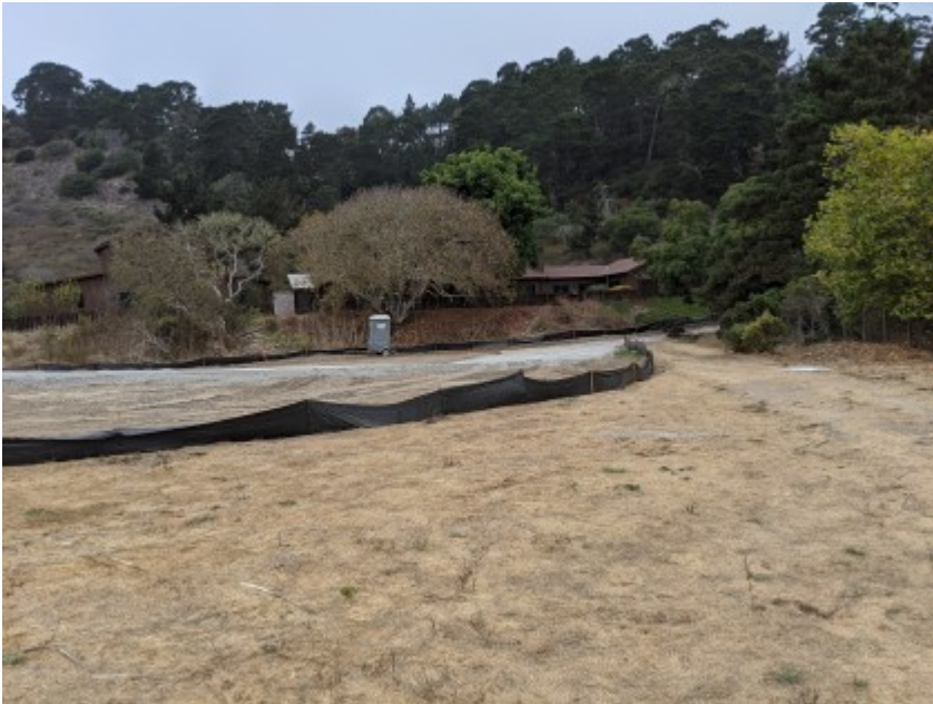
10/22/2020 - Intact exclusionary fencing surrounding construction area.
