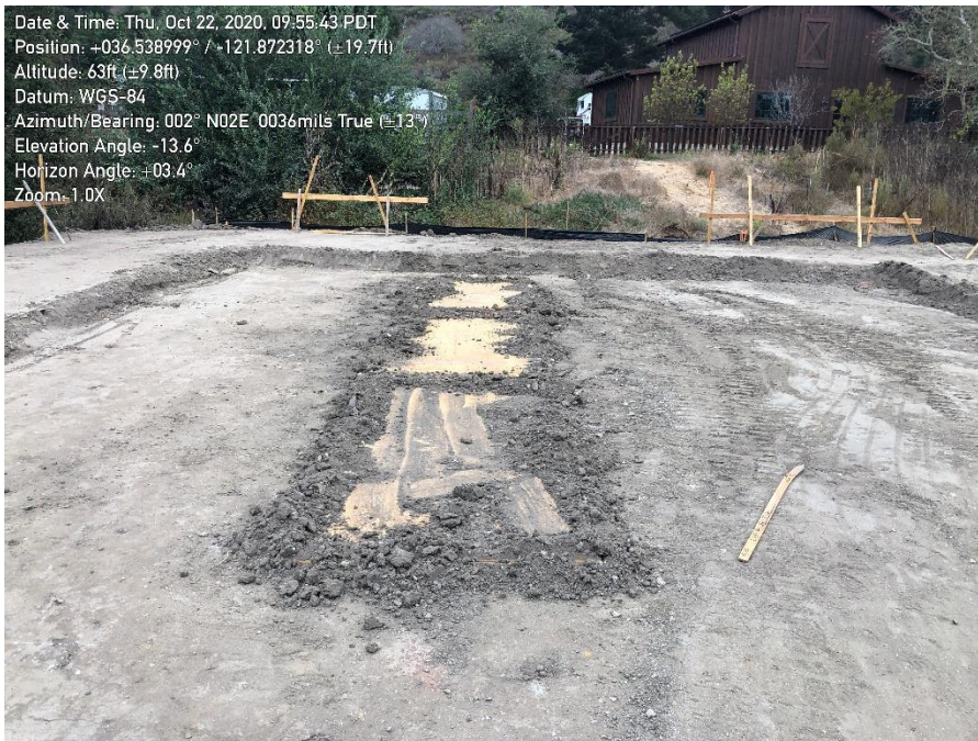
Photo 3. Carmel Valley Pump Station: Minor gap repaired along excavation covers.
