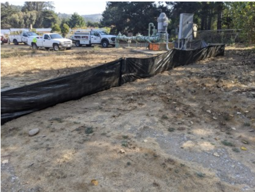
10/26/2020 - Installed exclusionary fencing surrounding construction area.
