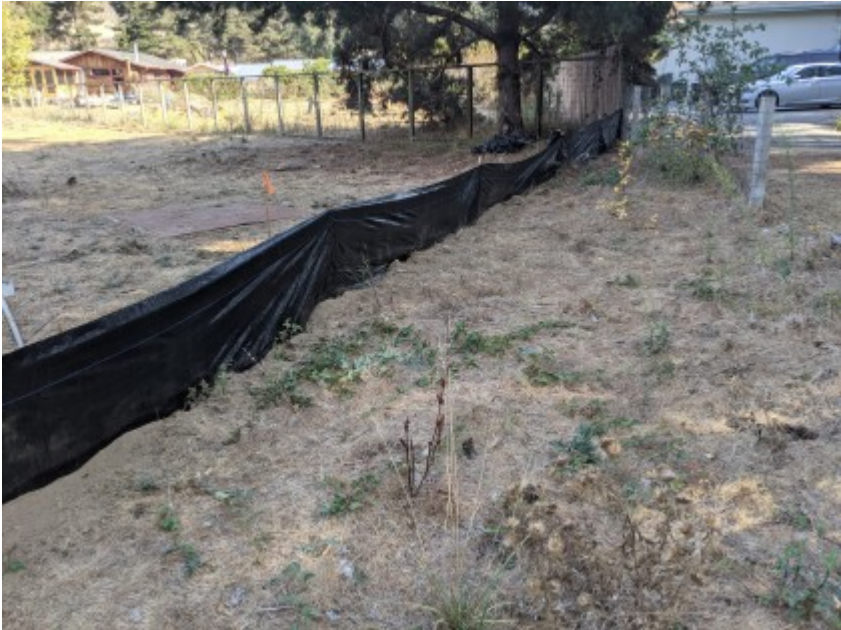
10/26/2020 - Installed exclusionary fencing surrounding construction area.
