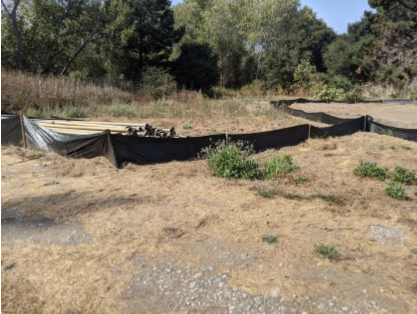
10/26/2020 - Installed exclusionary fencing surrounding construction area.
