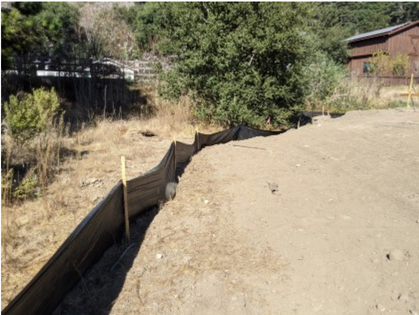
10/27/2020 - Intact exclusionary fencing surrounding construction area.
