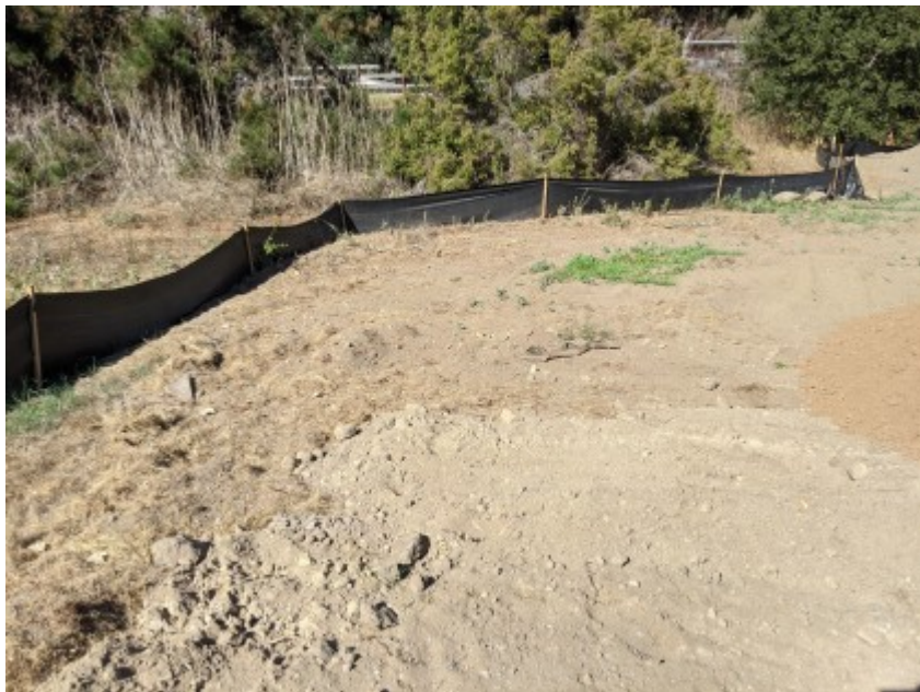
10/27/2020 - Intact exclusionary fencing surrounding construction area.
