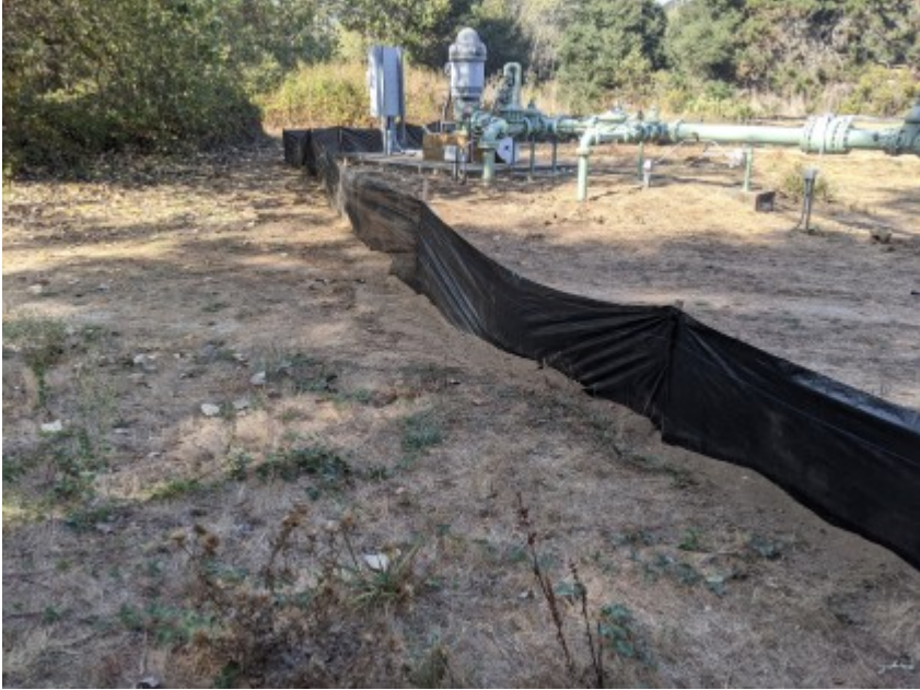
10/26/2020 - Installed exclusionary fencing surrounding construction area.
