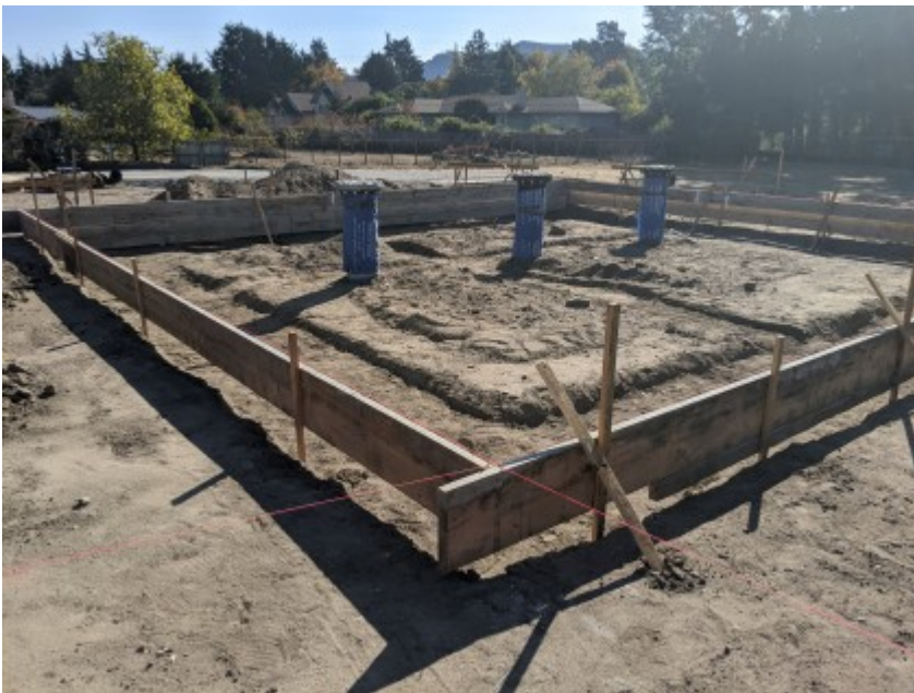
11/05/2020 - Completed concrete frames, waiting on concrete pouring.
