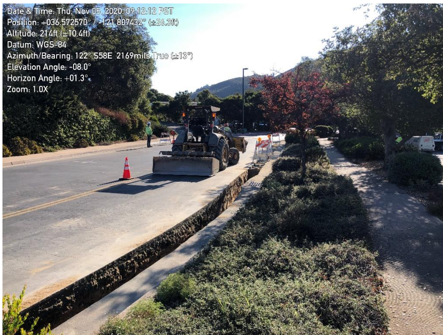
Photo 5. Ryan Ranch – Bishop Interconnection Improvements: Trenching along Blue Larkspur Lane.
