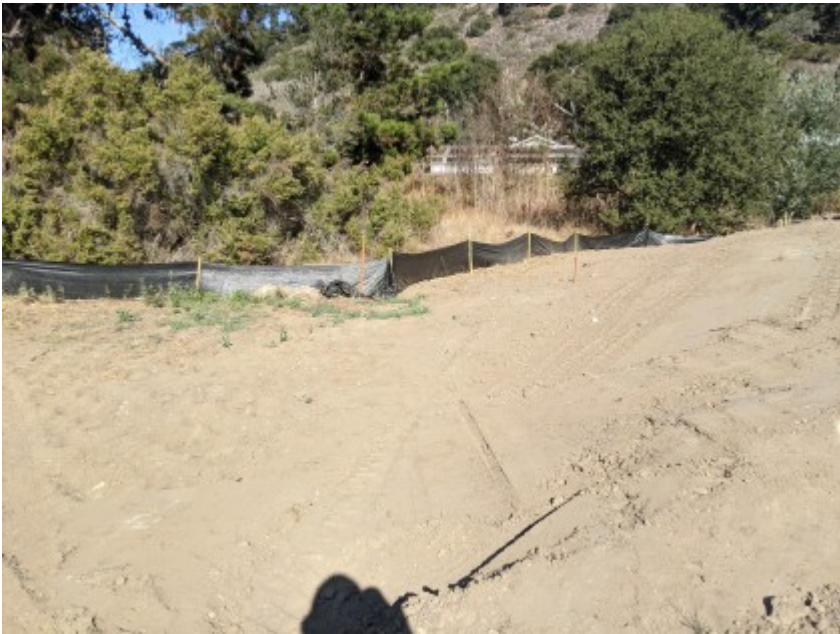
11/05/2020 - Intact silt fence surrounding construction area.
