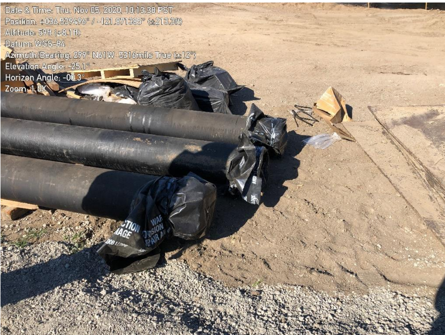
Photo 3. Carmel Valley Pump Station: ends of pipes covered.
