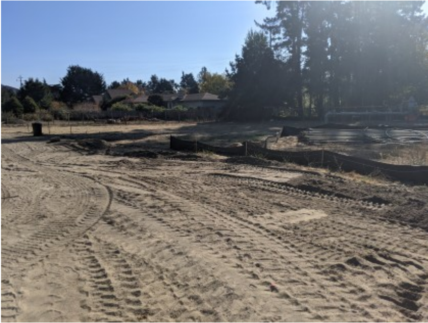
11/05/2020 - Intact silt fence surrounding construction area.
