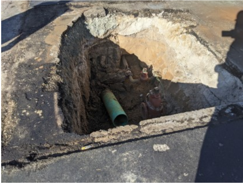
11/05/2020 - Tie-in work ongoing on Blue Larkspur Lane.
