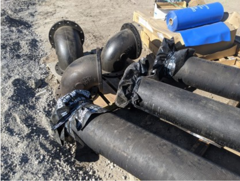
11/05/2020 - Covered and sealed pipeline onsite.
