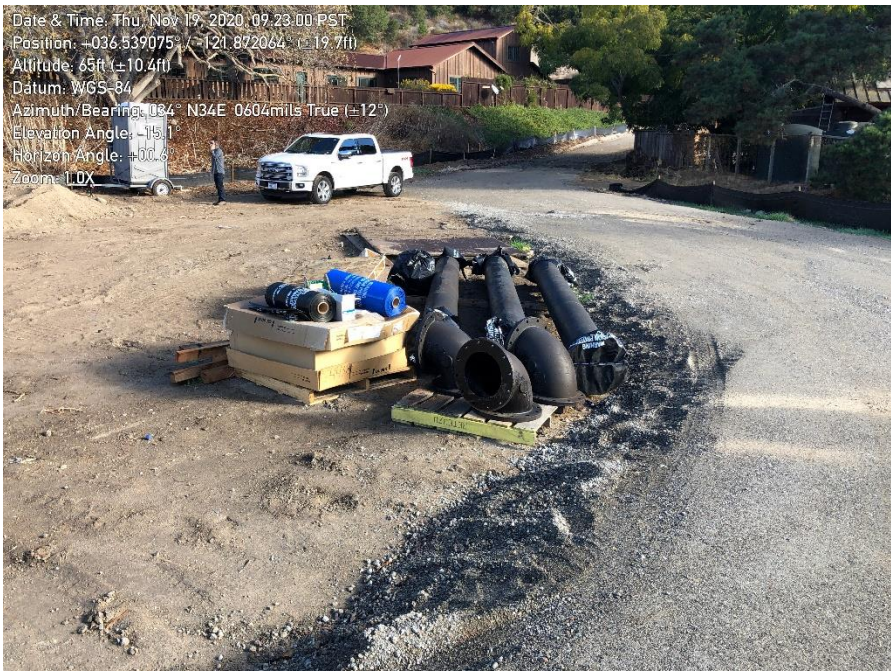
Photo 2. Carmel Valley Pump Station: ends of pipes covered.
