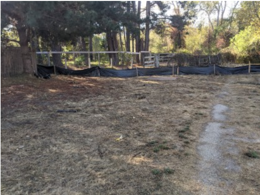
11/19/2020 - Intact silt fencing surrounding construction area
