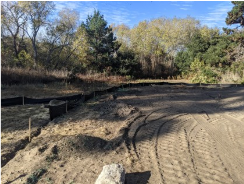
11/19/2020 - Intact silt fencing surrounding construction area
