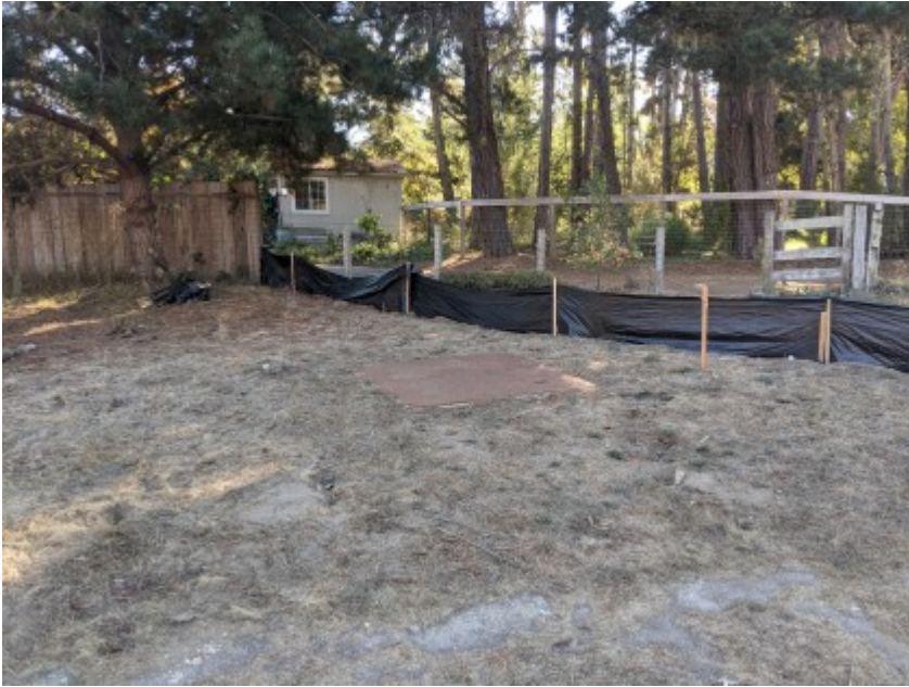
11/16/2020 - Intact silt fencing surrounding construction area
