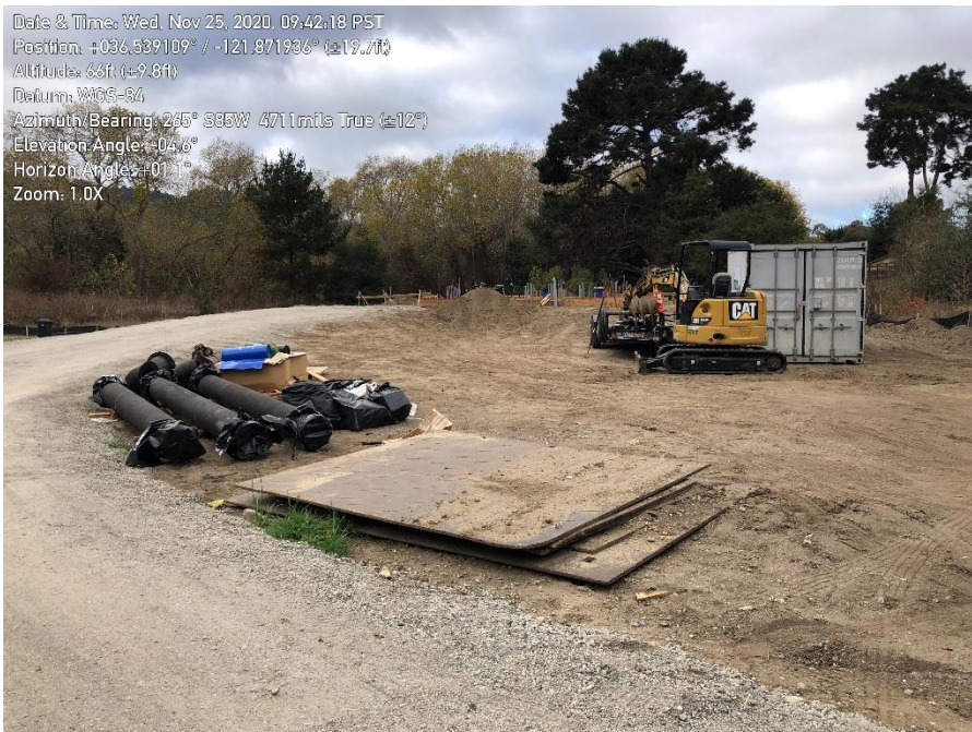
Photo 2. Pipe ends covered
