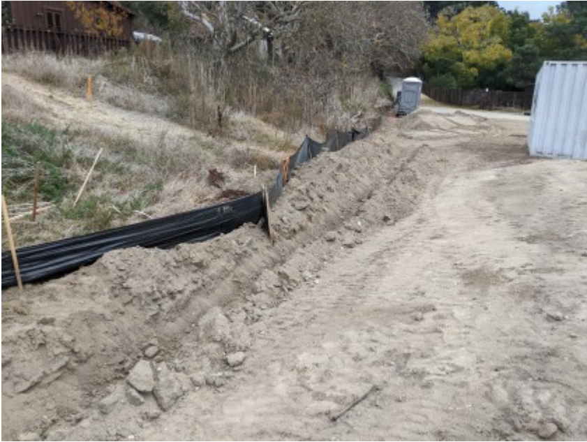
11/25/2020 - Intact silt fencing surrounding the construction area.
