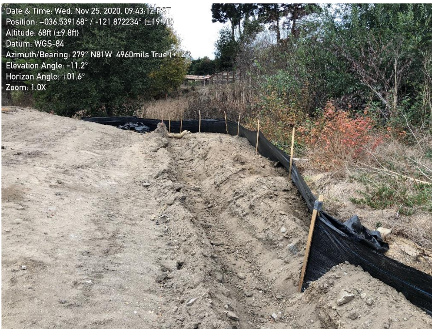
Photo 1. Silt fence in adequate condition.
