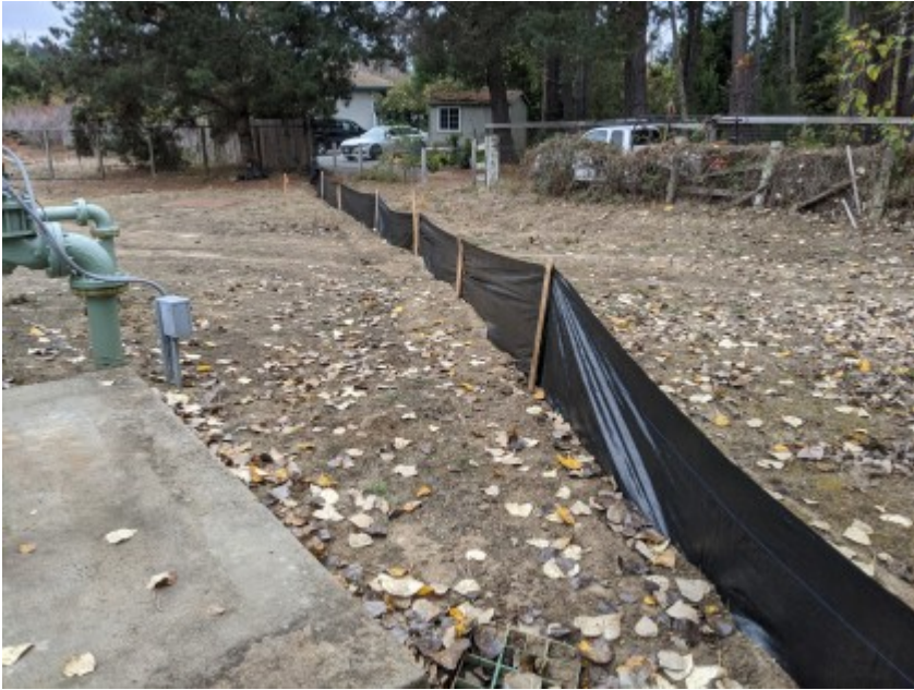
11/25/2020 - Intact silt fencing surrounding the construction area.
