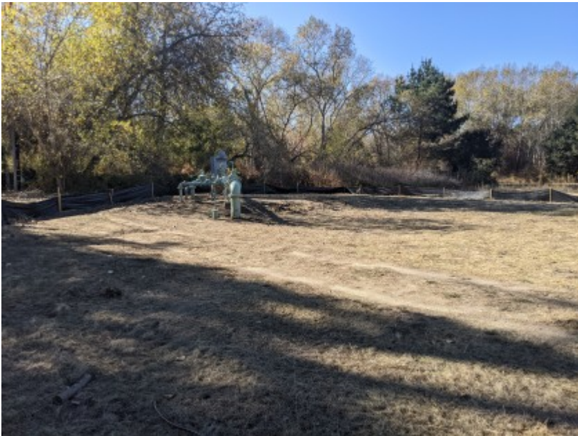
11/24/2020 - Intact silt fencing surrounding construction area.
