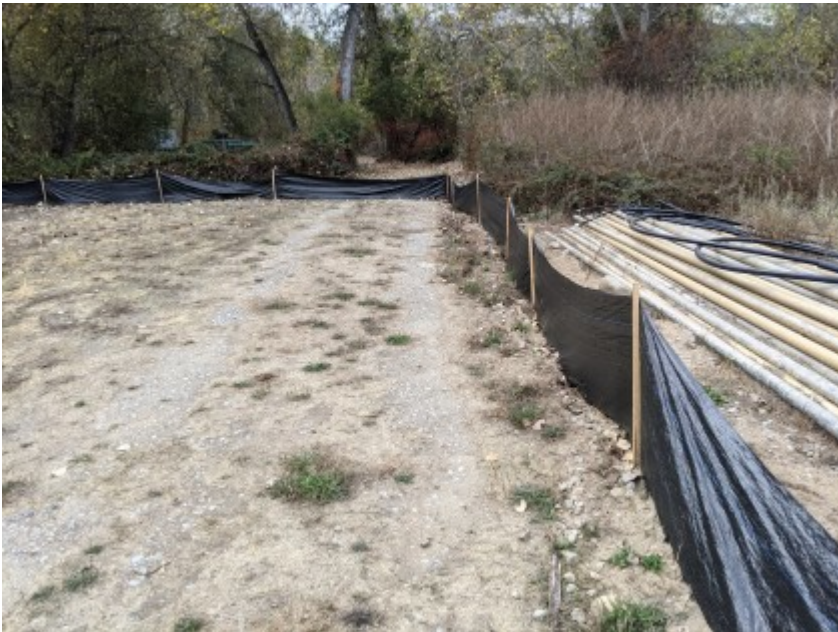
11/25/2020 - Intact silt fencing surrounding the construction area.
