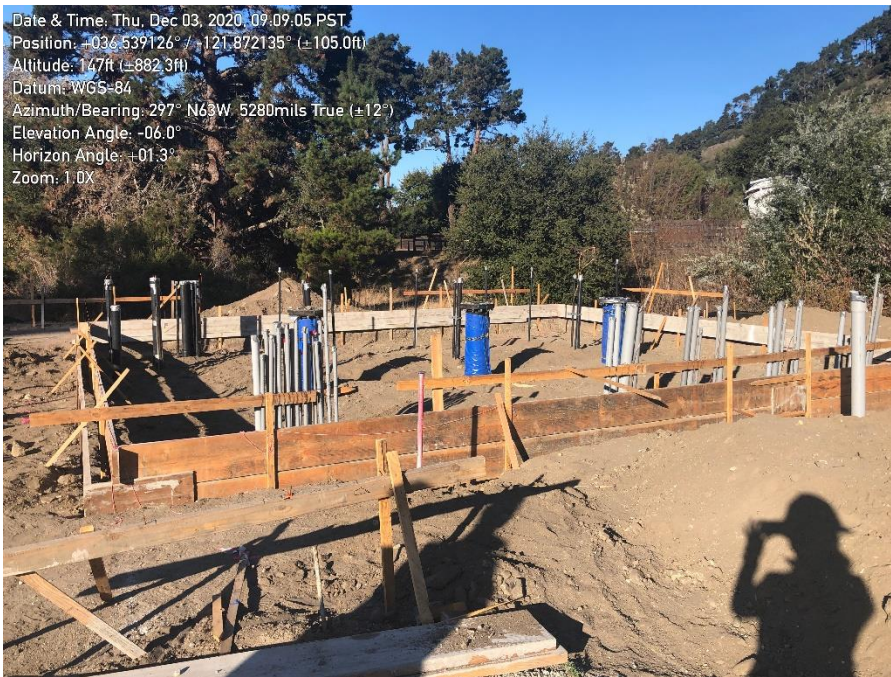
Photo 3. Conduit installation was completed.
