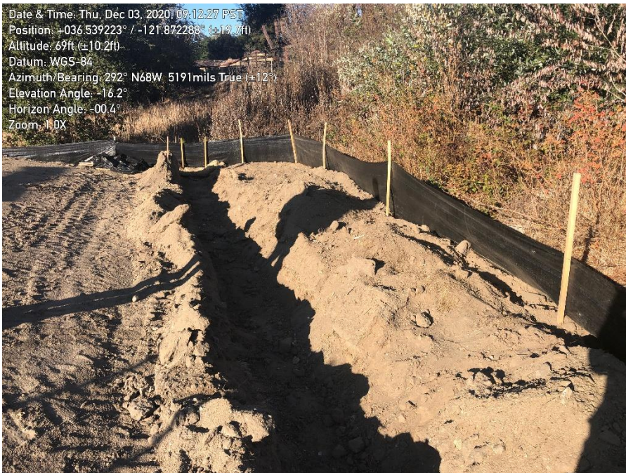
Photo 2. Silt fence in adequate condition.
