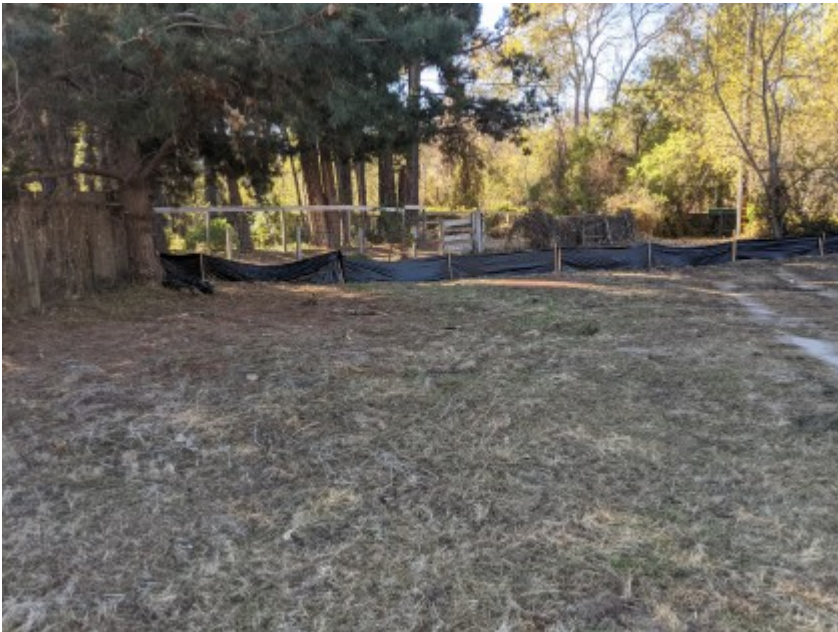
11/30/2020 - Intact silt fencing surrounding the construction area.
