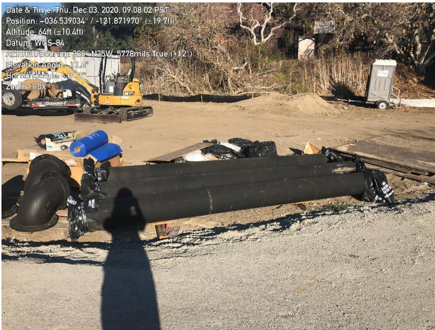
Photo 1. Pipe stored on site covered.
