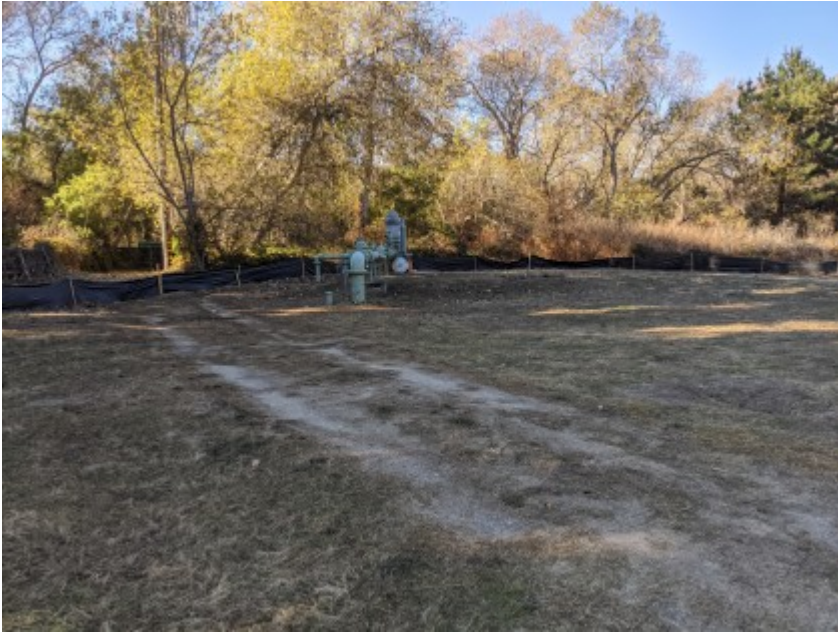
11/30/2020 - Intact silt fencing surrounding the construction area.
