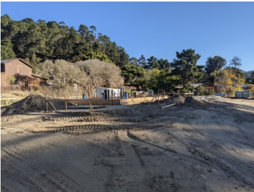
11/30/2020 - Intact silt fencing surrounding the construction area.
