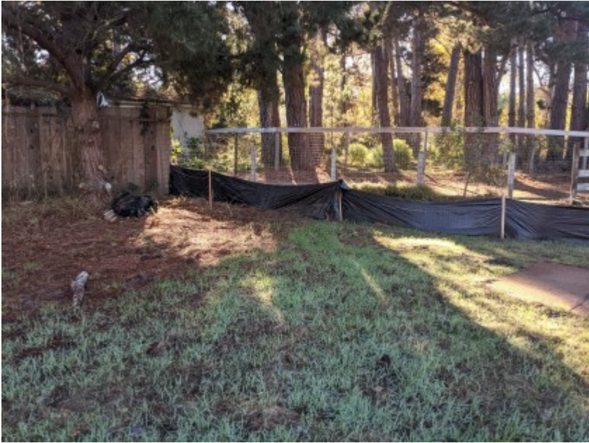
01/04/2021 - Intact exclusionary fencing surrounding work area.
