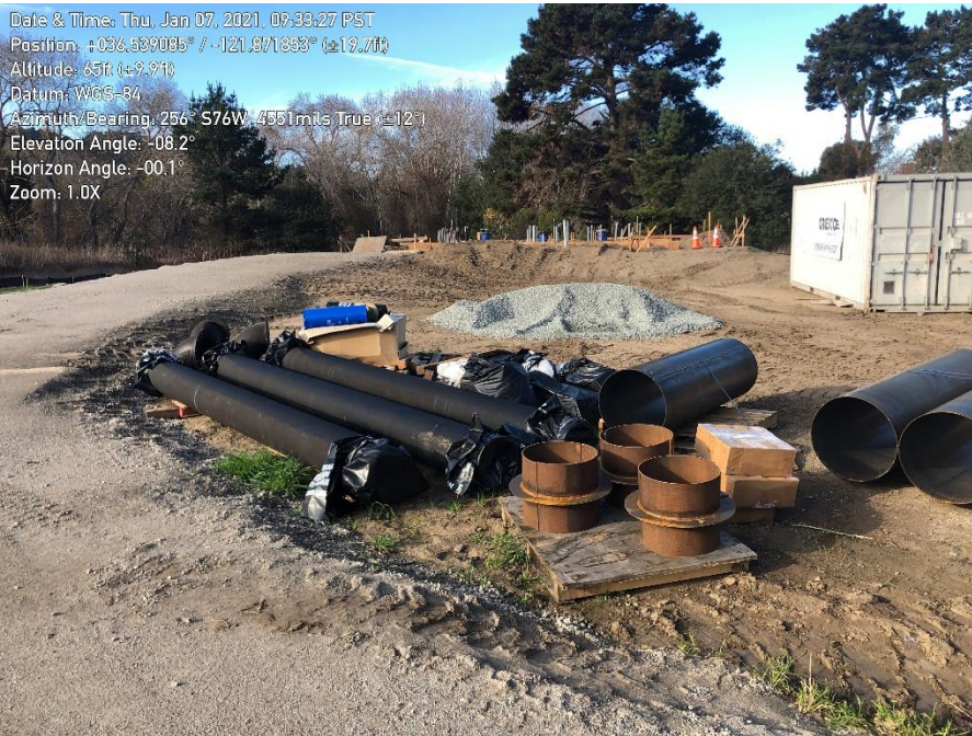
Photo 4. Smaller pipes stored on site capped.
