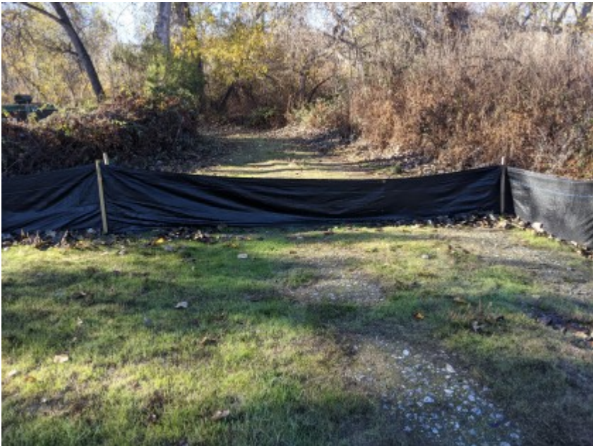
01/04/2021 - Intact exclusionary fencing surrounding work area.
