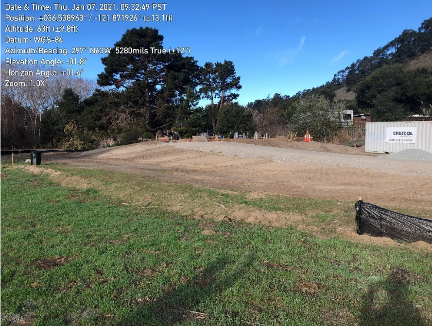
Photo 1. Overall conditions at project site.
