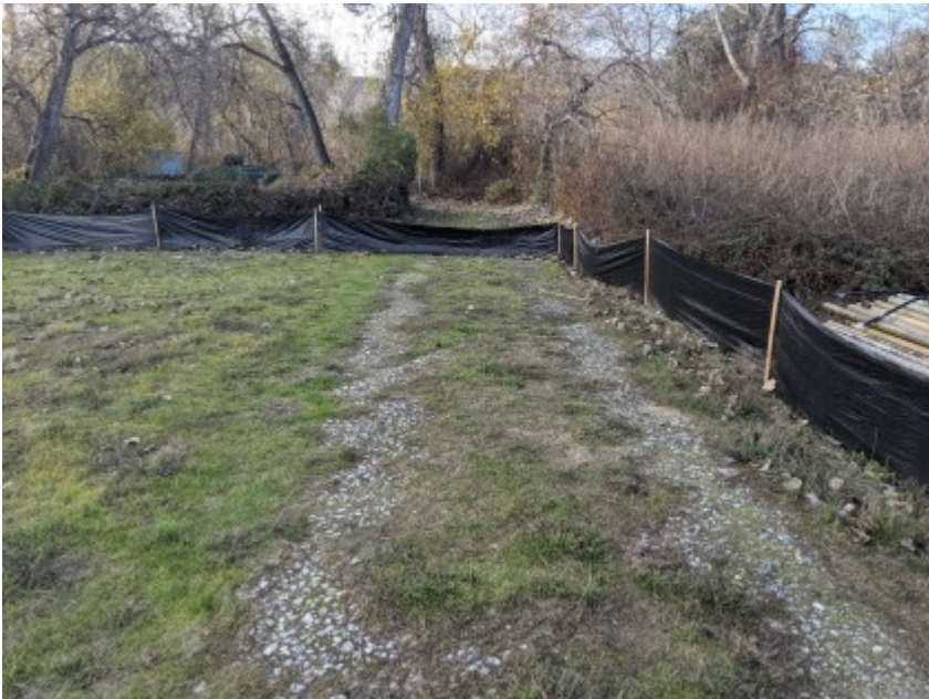
01/07/2021 - Intact exclusionary fencing surrounding work area.
