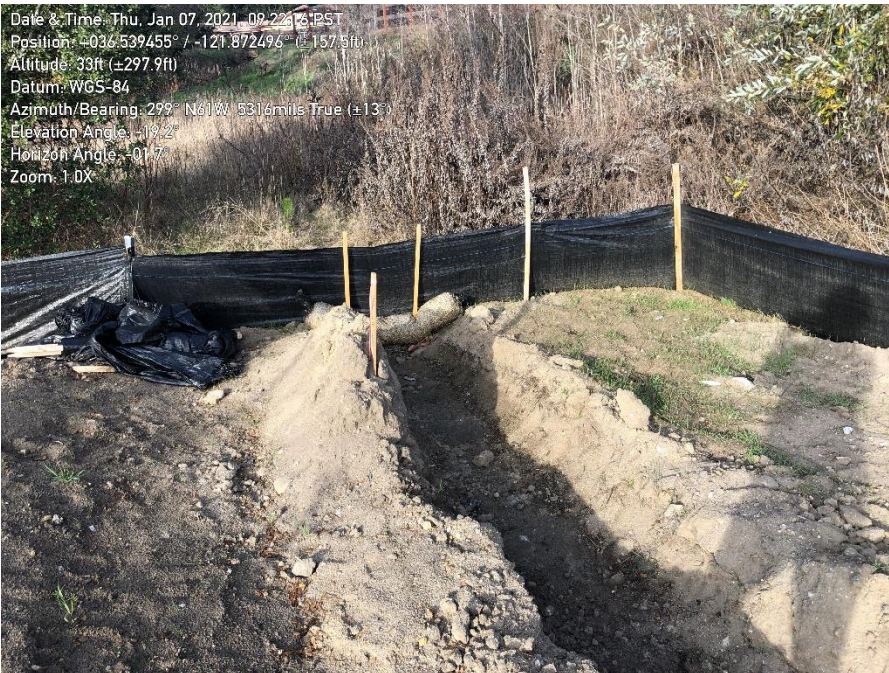
Photo 2. Silt fence and drainage area adjacent to graded pad.
