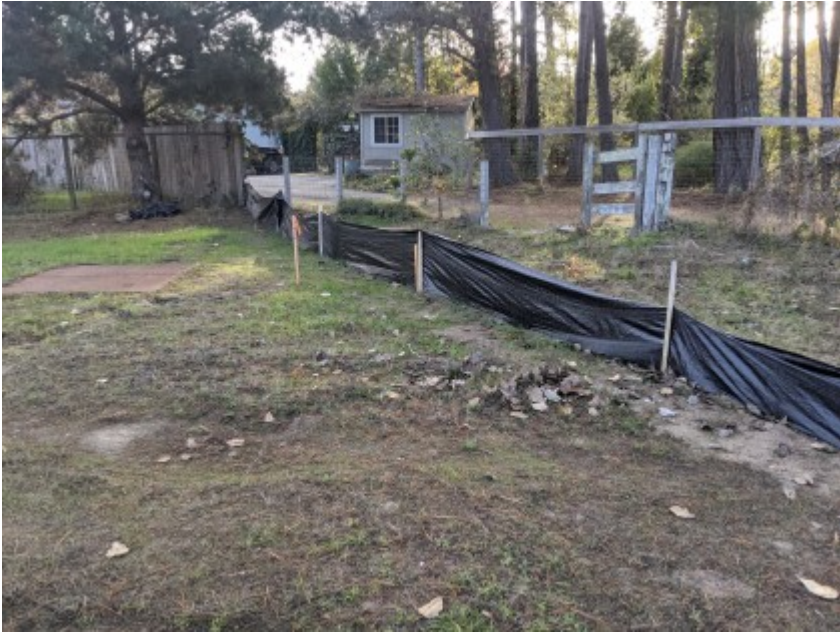
01/07/2021 - Intact exclusionary fencing surrounding work area.
