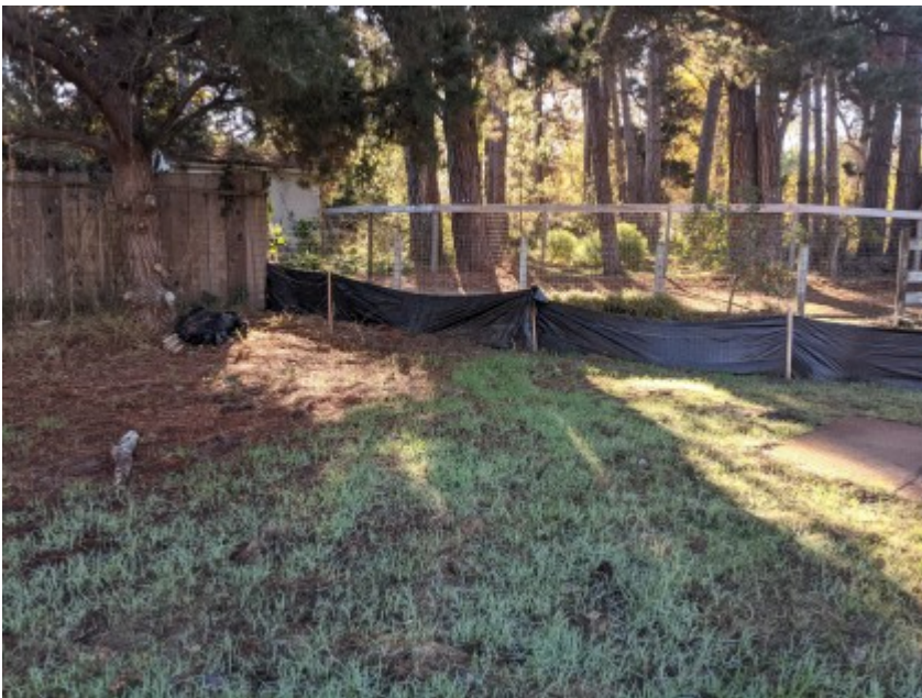
01/04/2021 - Intact exclusionary fencing surrounding work area.
