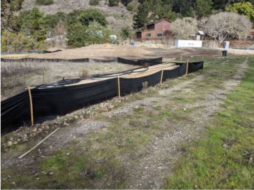
01/07/2021 - Intact exclusionary fencing surrounding work area.
