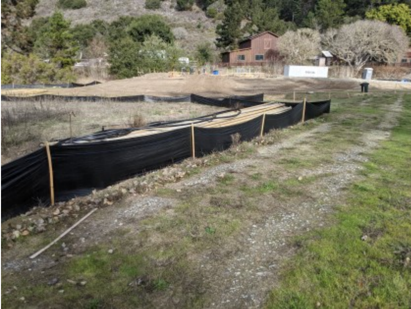
01/04/2021 - Intact exclusionary fencing surrounding work area.
