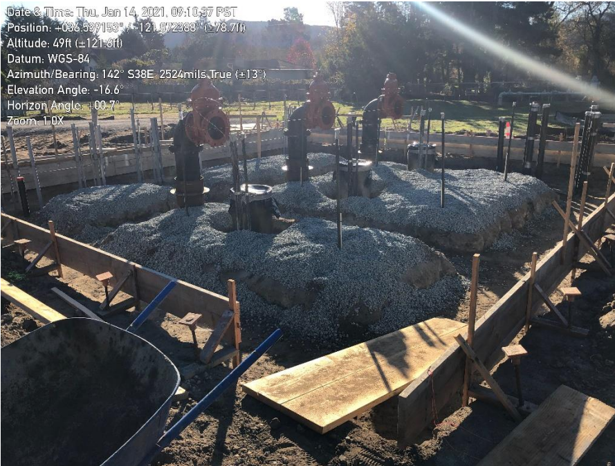
Photo 3. Graded pad with pipes installed.
