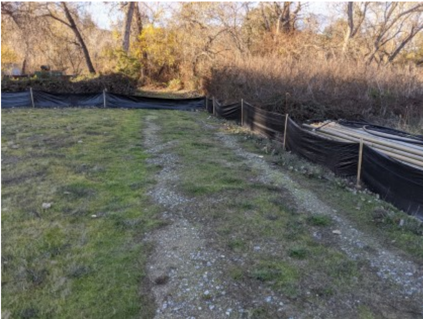
01/14/2021 - Intact exclusionary fencing surrounding work area.
