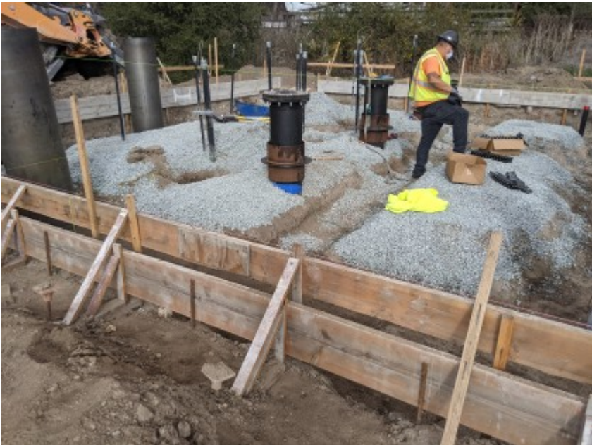
01/11/2021 - Crew onsite assembling pipe fittings in preparation for concrete pouring
