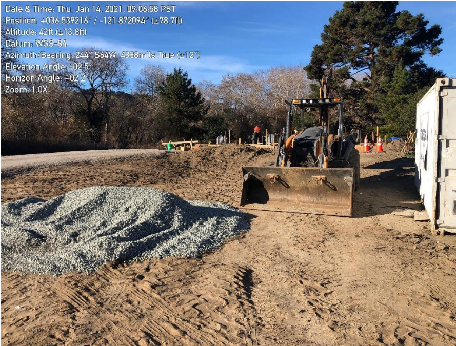
Photo 1. Overall conditions at project site.
