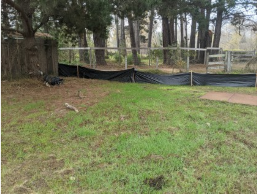
01/11/2021 - Intact exclusionary fencing surrounding work area.
