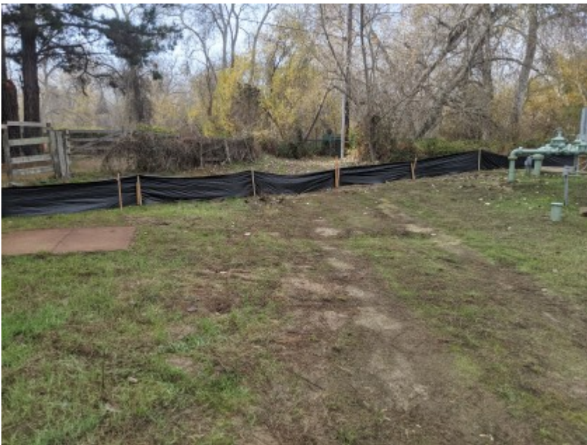
01/11/2021 - Intact exclusionary fencing surrounding work area.
