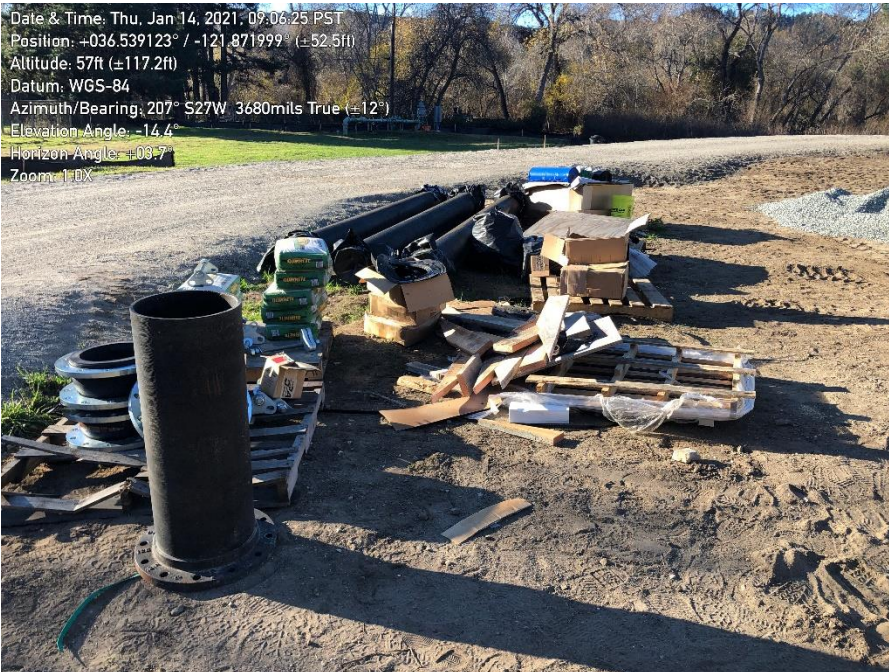
Photo 4. Smaller pipes stored on site capped.
