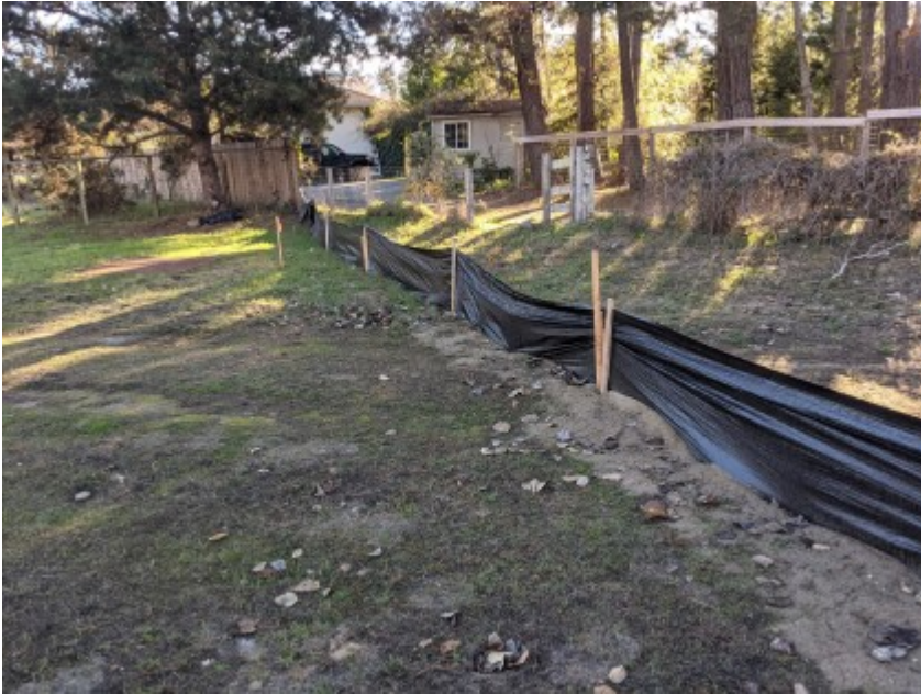
01/14/2021 - Intact exclusionary fencing surrounding work area.
