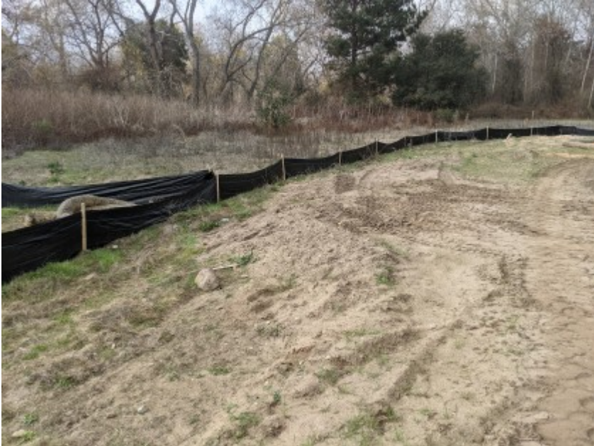
01/11/2021 - Intact exclusionary fencing surrounding work area.
