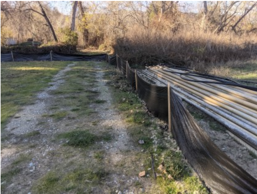
01/21/2021 - Intact exclusionary fencing surrounding work area.
