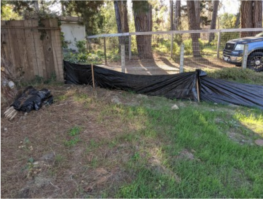
01/18/2021 - Intact exclusionary fencing surrounding work area.
