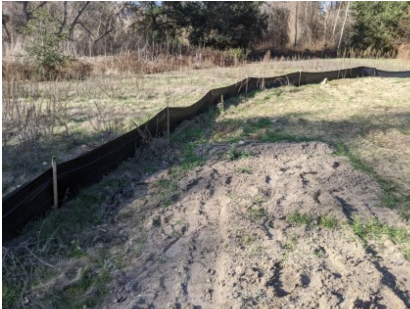
01/18/2021 - Intact exclusionary fencing surrounding work area.
