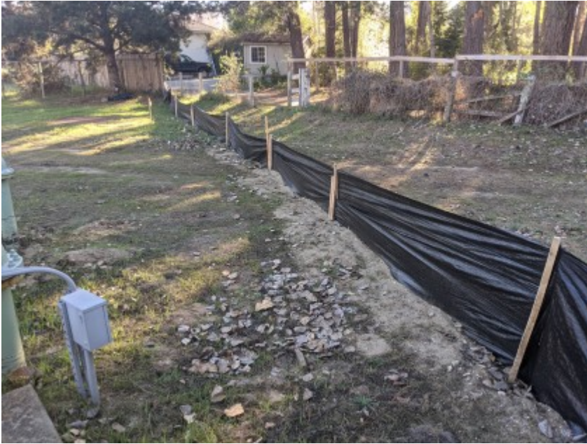
01/21/2021 - Intact exclusionary fencing surrounding work area.
