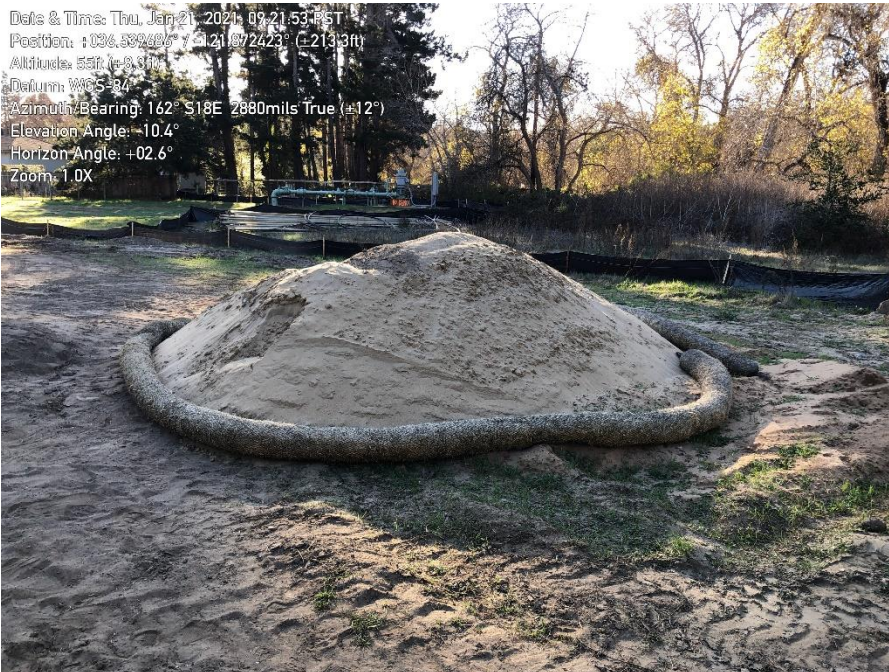
Photo 4. BMPs including straw wattle and silt fence in place.
