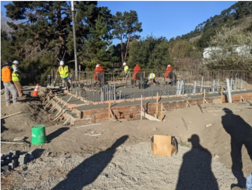
01/21/2021 - Concrete pouring for pump station slab.
