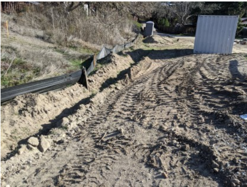
01/18/2021 - Intact exclusionary fencing surrounding work area.
