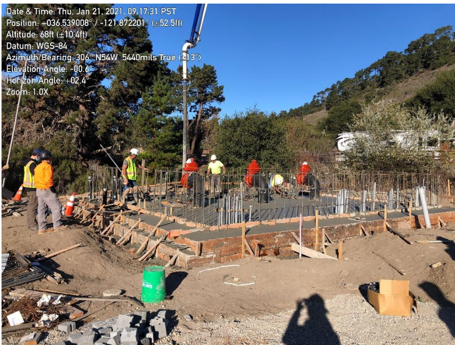
Photo 2. Pad after concrete pour.
