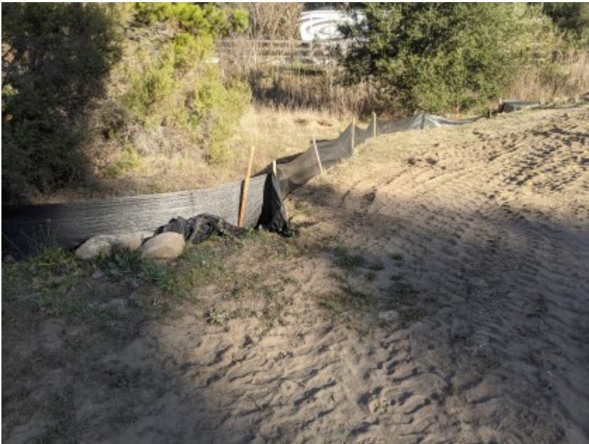
01/21/2021 - Intact exclusionary fencing surrounding work area.
