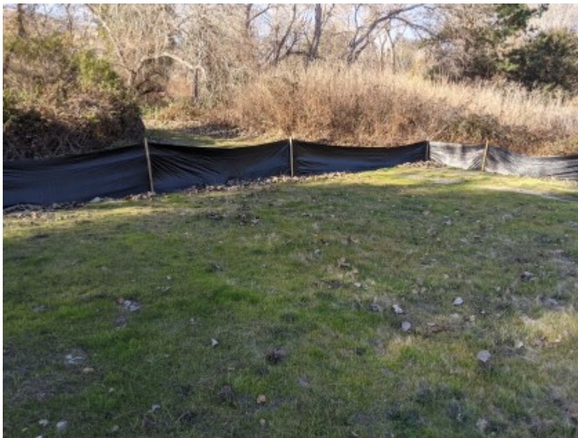
01/18/2021 - Intact exclusionary fencing surrounding work area.
