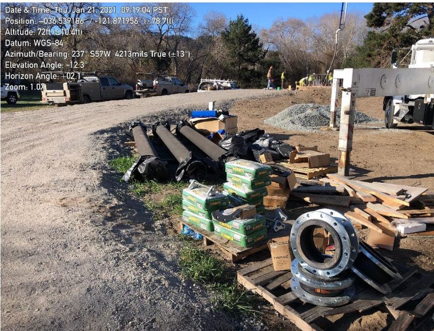
Photo 3. Smaller pipes stored on site capped.
