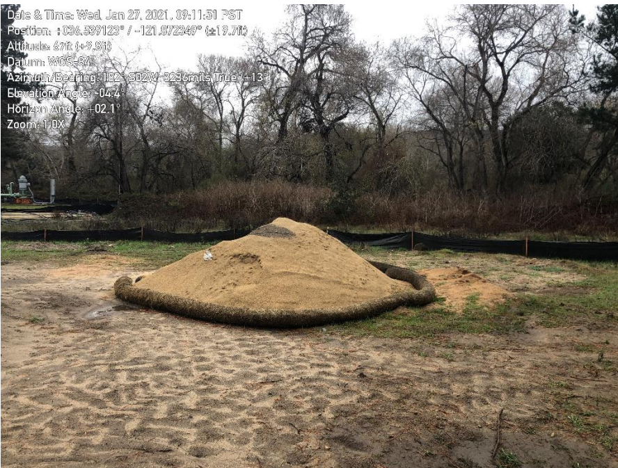
Photo 4. BMPs in place around stock pile.
