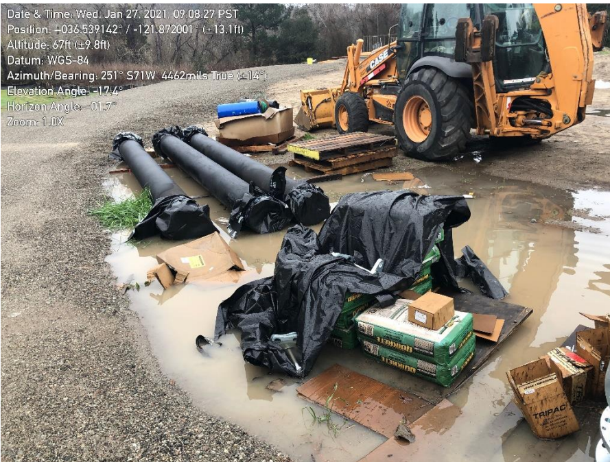
Photo 6. Pipes stored on site capped.
