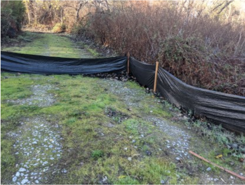
01/29/2021 - Intact exclusionary fencing surrounding work area.
