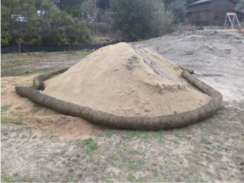
01/27/2021 - Intact straw wattle erosion control.
