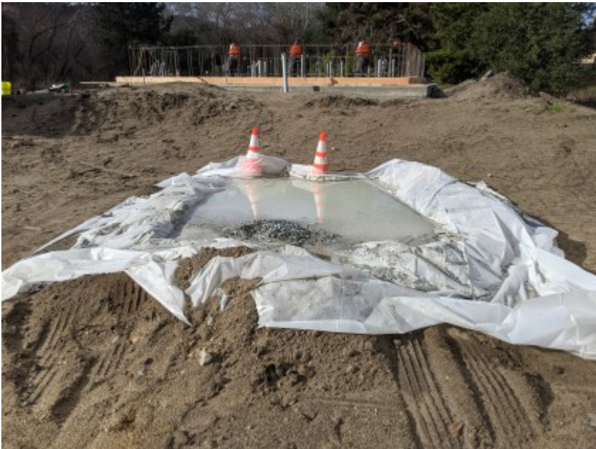
01/25/2021 - Concrete washout containment within work area.
