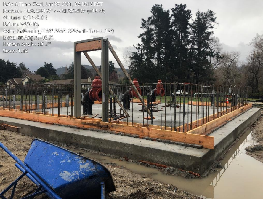
Photo 3. Partially developed pad.
