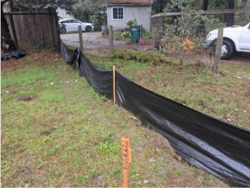
01/27/2021 - Intact exclusionary fencing surrounding work area.
