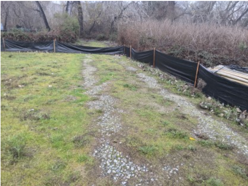
01/27/2021 - Intact exclusionary fencing surrounding work area.
