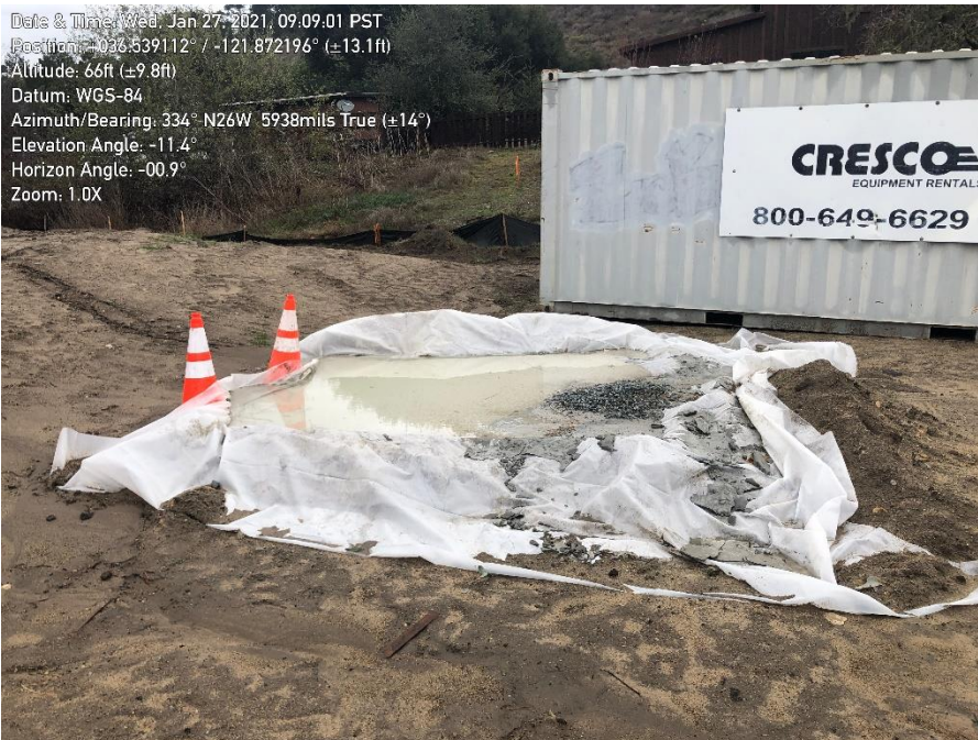
Photo 2. Concrete washout contained.
