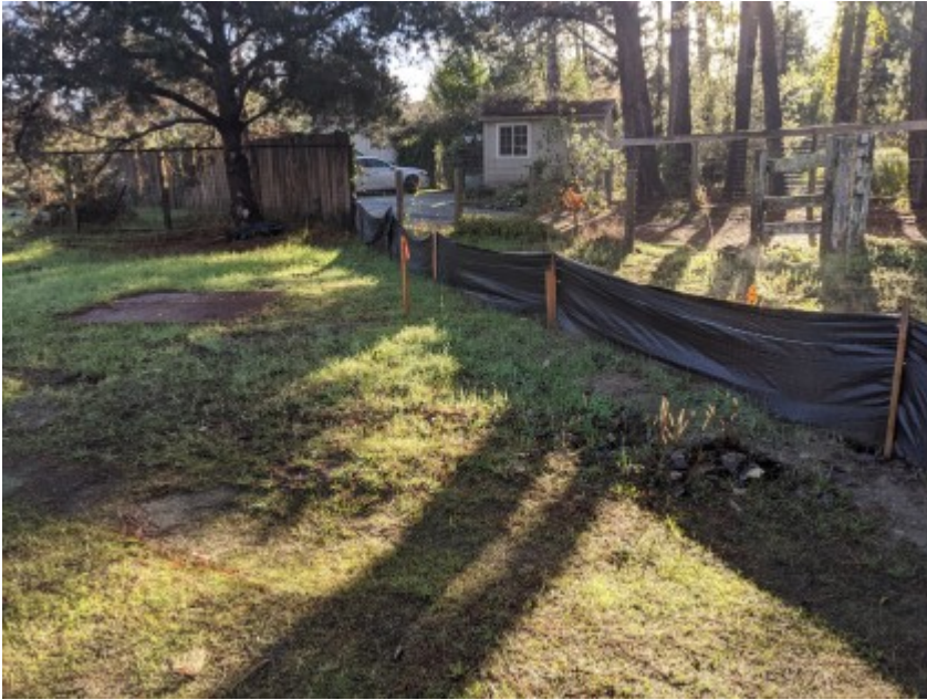
01/29/2021 - Intact exclusionary fencing surrounding work area.
