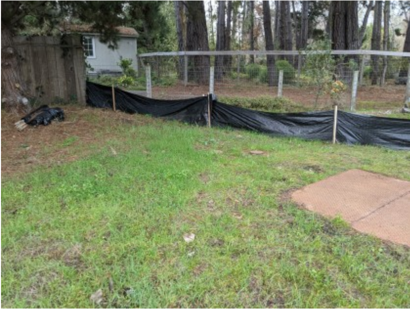
01/25/2021 - Intact exclusionary fencing surrounding work area.
