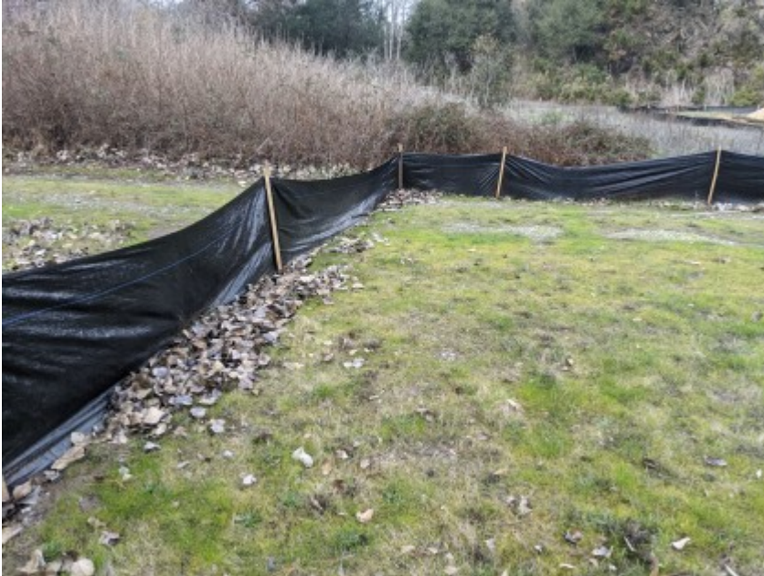
01/25/2021 - Intact exclusionary fencing surrounding work area.
