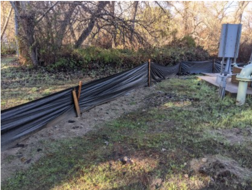
01/29/2021 - Intact exclusionary fencing surrounding work area.
