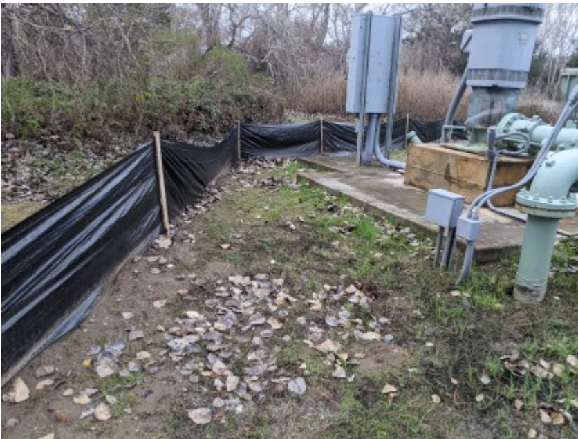
01/25/2021 - Intact exclusionary fencing surrounding work area.
