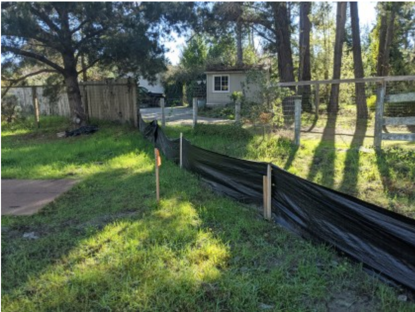
02/18/2021 - Intact exclusionary fencing surrounding work area.
