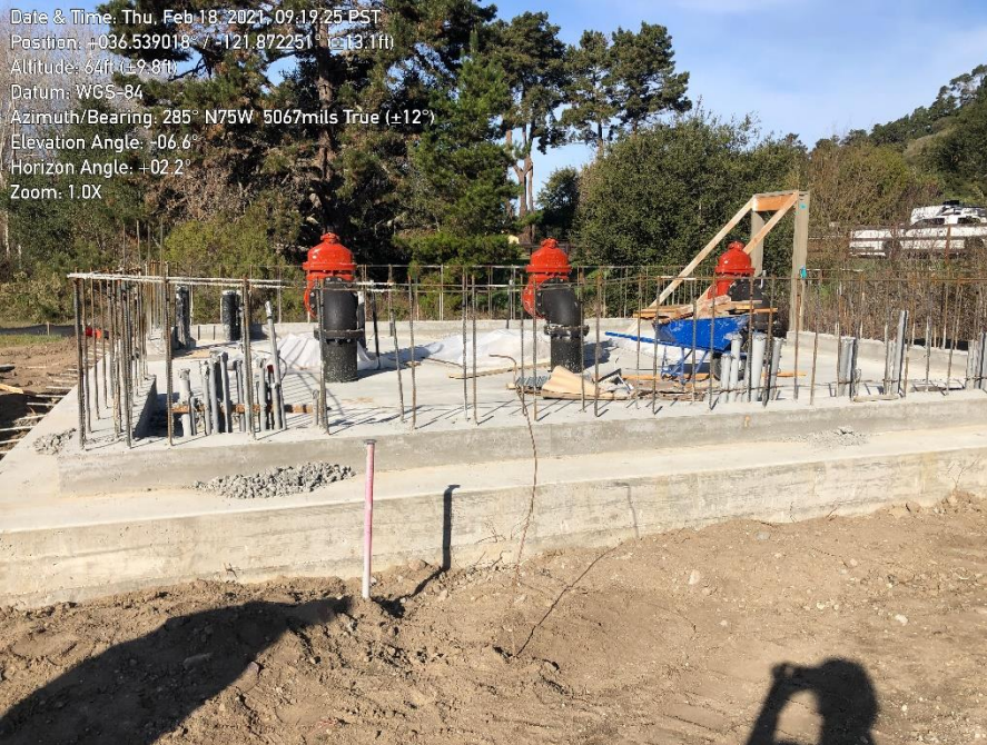
Photo 1. Foundation for pump station.
