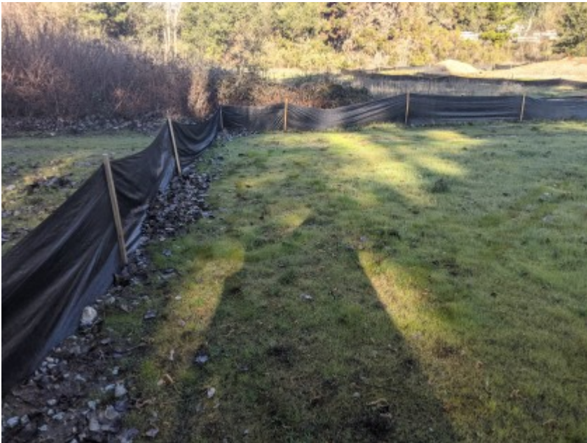
02/17/2021 - Intact exclusionary fencing surrounding work area.
