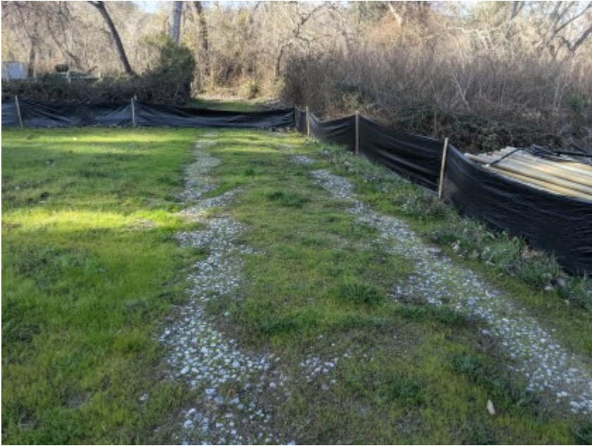
02/18/2021 - Intact exclusionary fencing surrounding work area.
