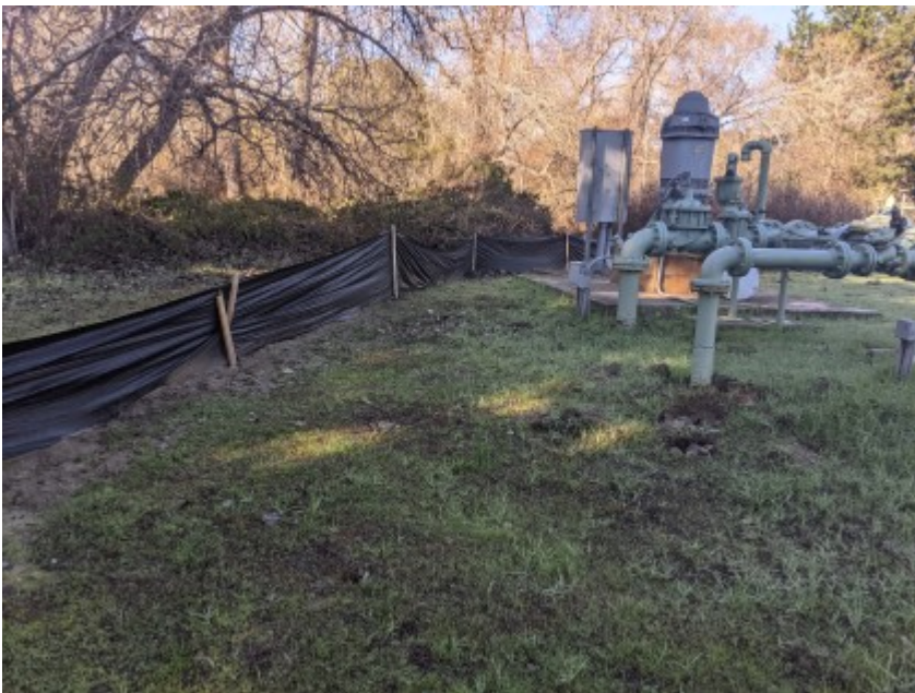
02/17/2021 - Intact exclusionary fencing surrounding work area.
