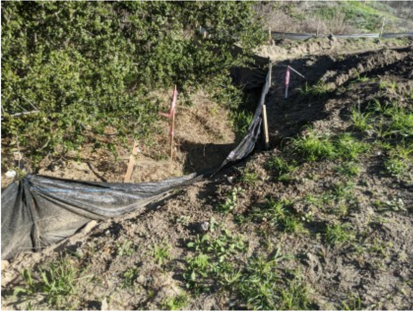
02/17/2021 - Section of exclusionary fencing damaged by erosional feature.
