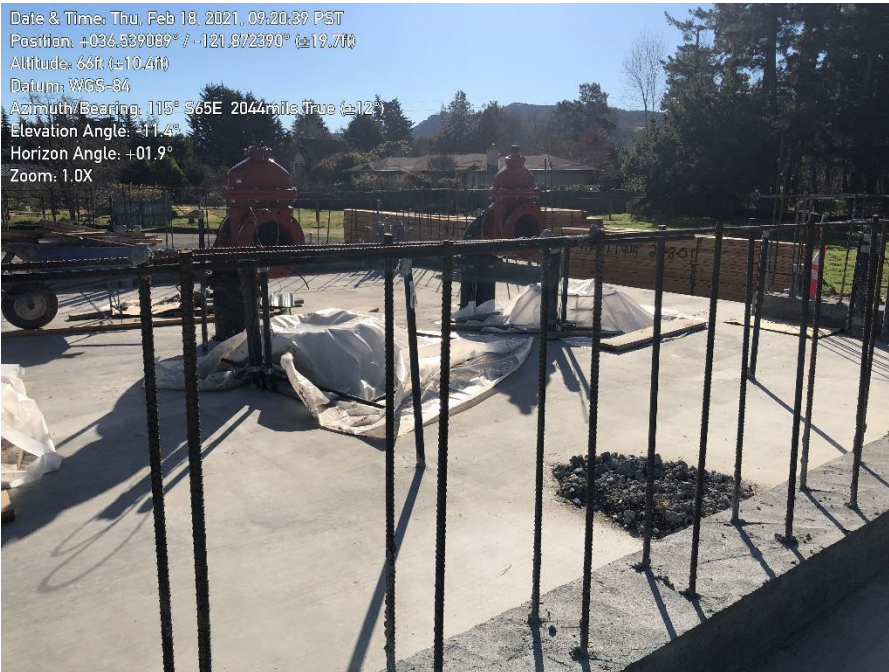
Photo 4. Openings on pump station foundation covered.
