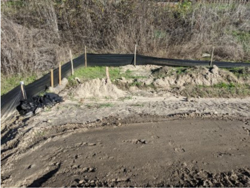
02/17/2021 - Intact exclusionary fencing surrounding work area.
