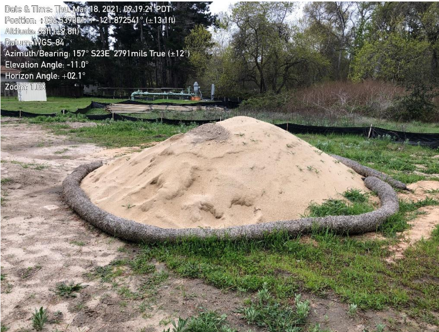
Photo 4. BMPs in place.
