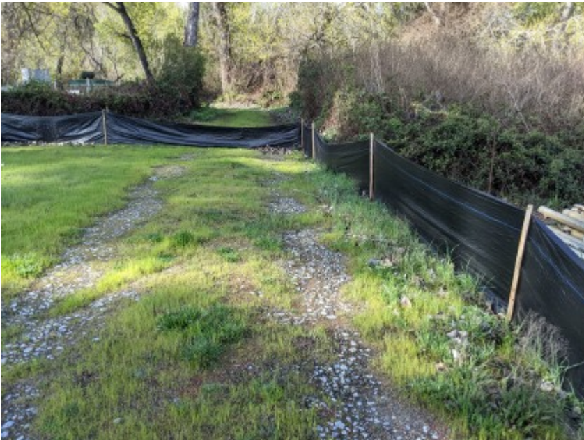
03/15/2021 - Intact exclusionary fencing surrounding work area.
