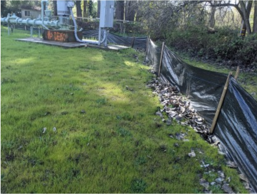
03/15/2021 - Intact exclusionary fencing surrounding work area.
