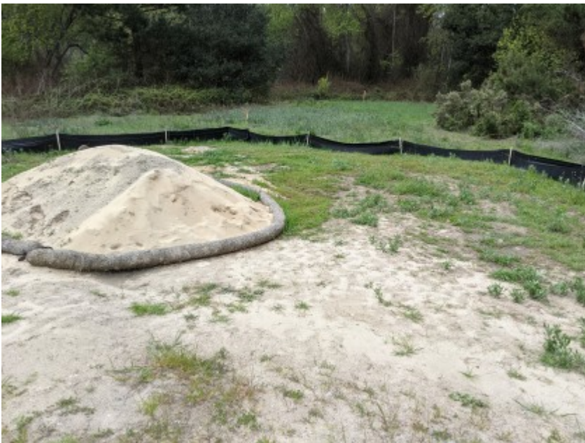
03/17/2021 - Intact exclusionary fencing surrounding work area.
