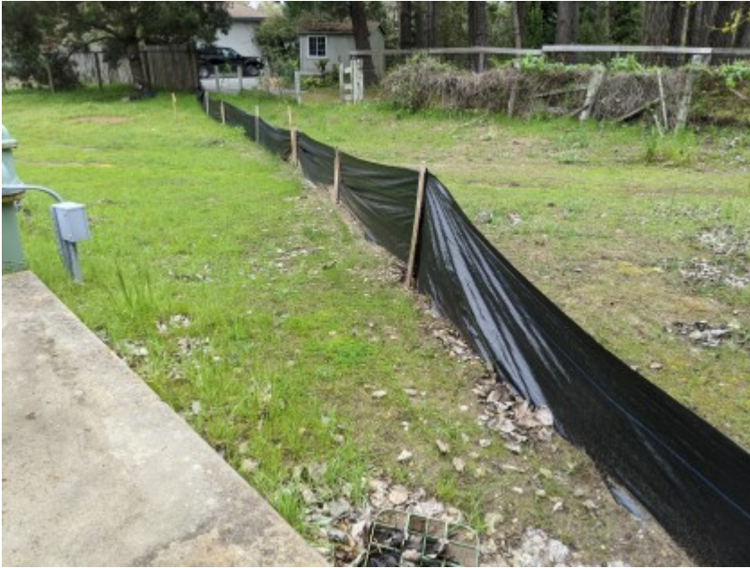
03/17/2021 - Intact exclusionary fencing surrounding work area.
