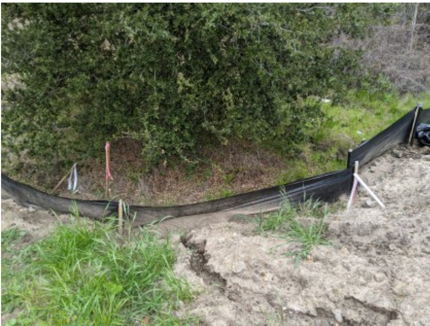
03/18/2021 - Intact exclusionary fencing surrounding work area.
