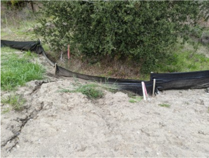
03/17/2021 - Intact exclusionary fencing surrounding work area.
