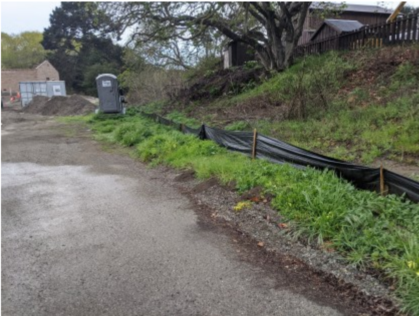
03/15/2021 - Intact exclusionary fencing surrounding work area.
