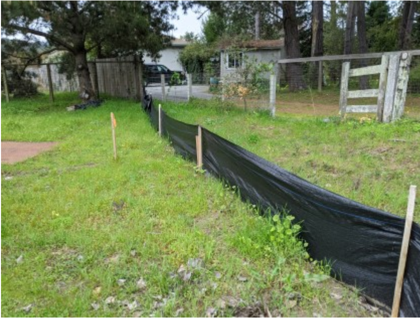
03/18/2021 - Intact exclusionary fencing surrounding work area.
