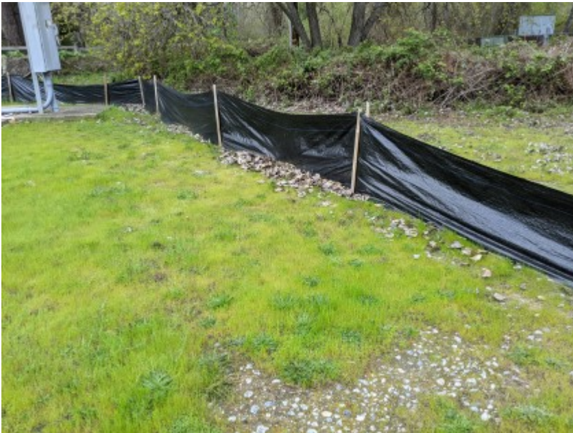
03/18/2021 - Intact exclusionary fencing surrounding work area.
