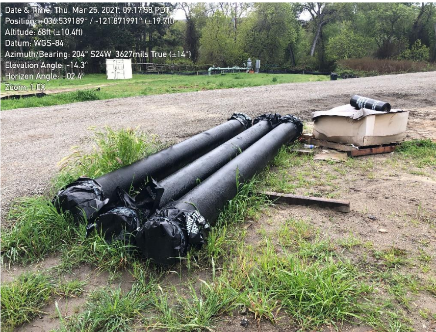
Photo 3. Pipes capped.
