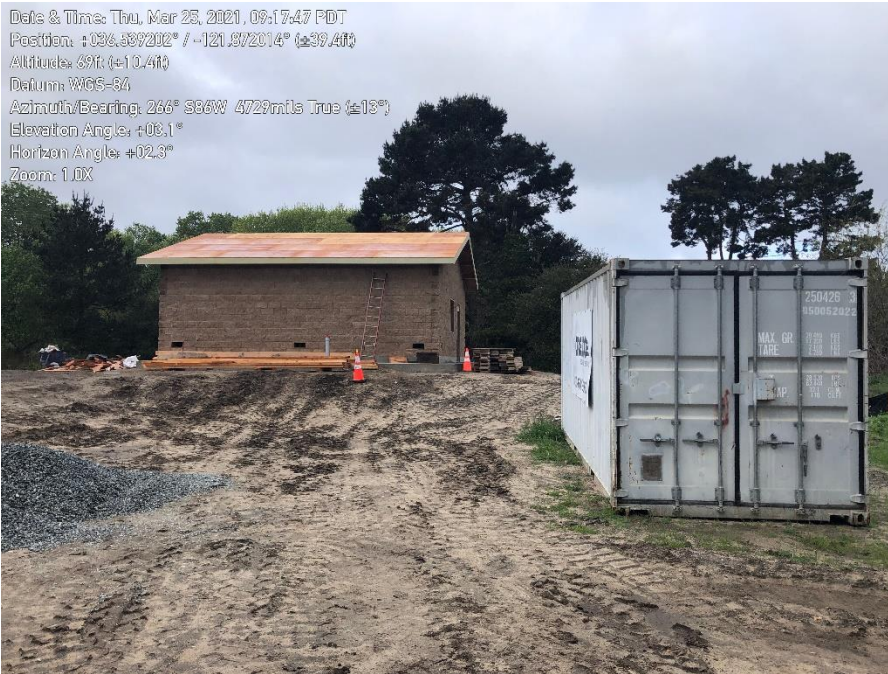
Photo 1. Pump station and overall site conditions.
