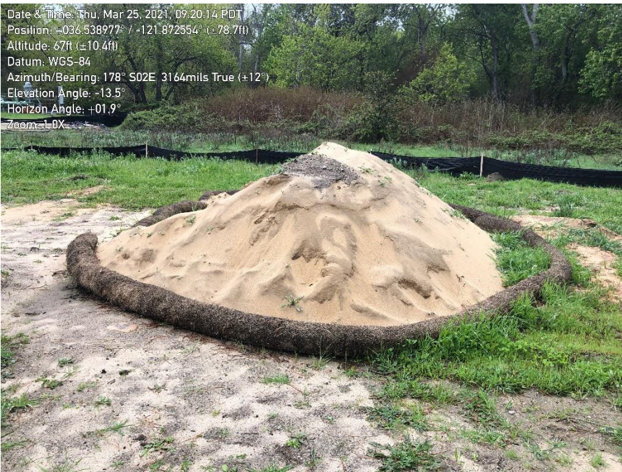
Photo 4. BMPs in place.
